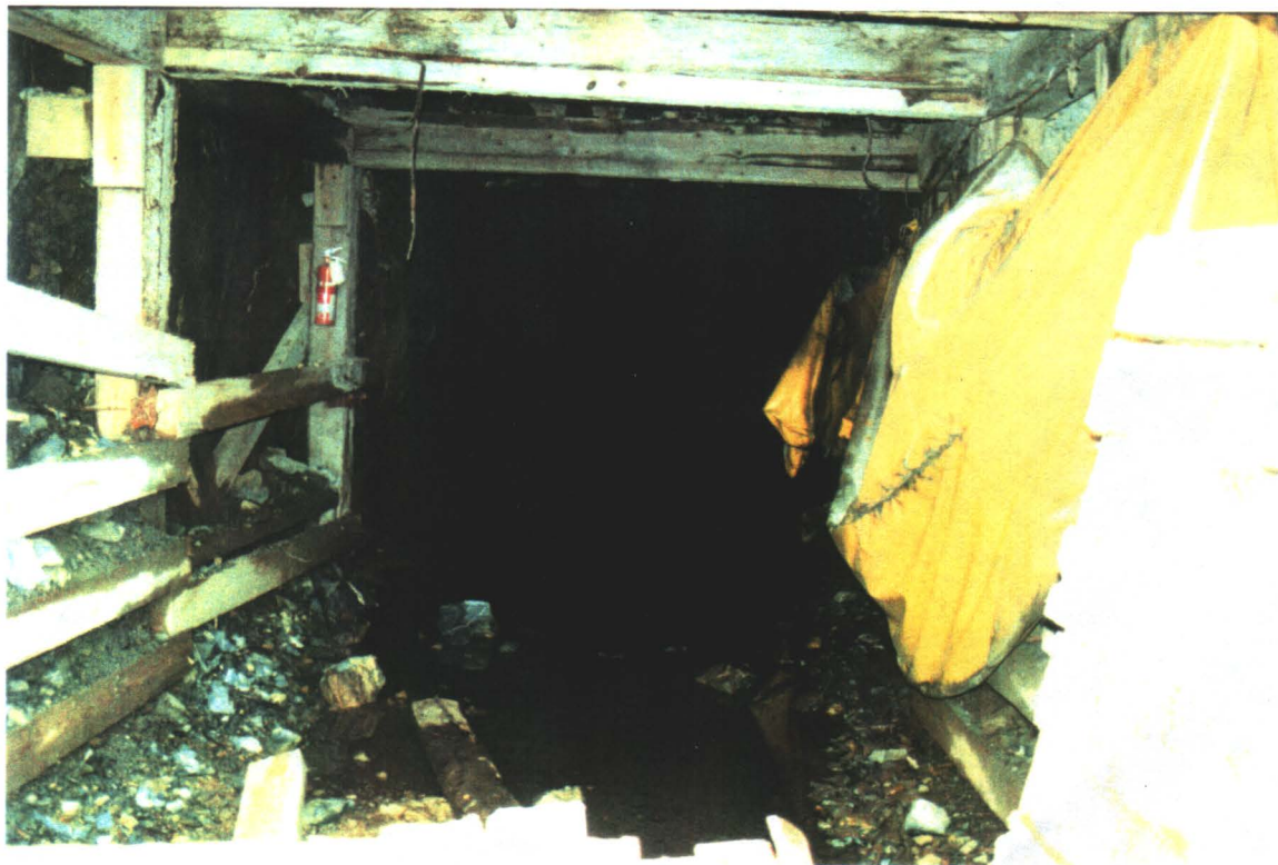
INTERIOR OF OPEN ADIT
