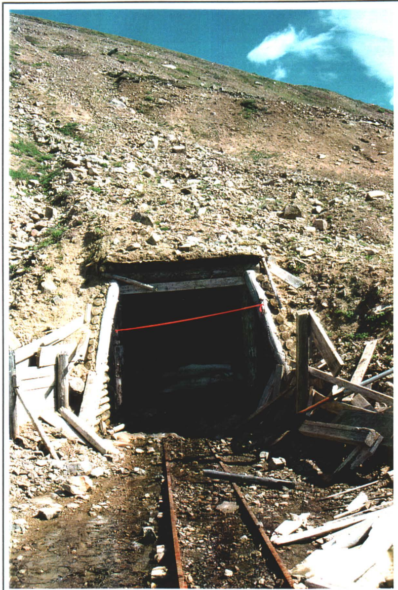
Photo # 10 - Adit - Exterior
