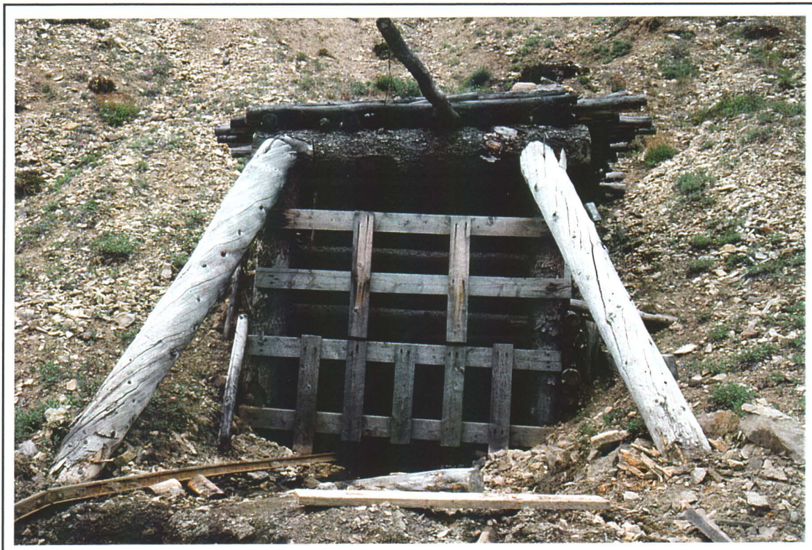
Photo # 5 - Lower Adit - A 1
