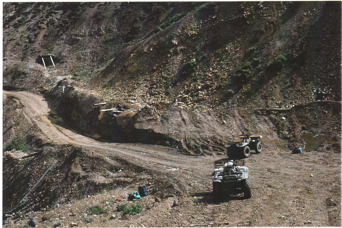
Photo # 8 - Road and Remains of Trestle
