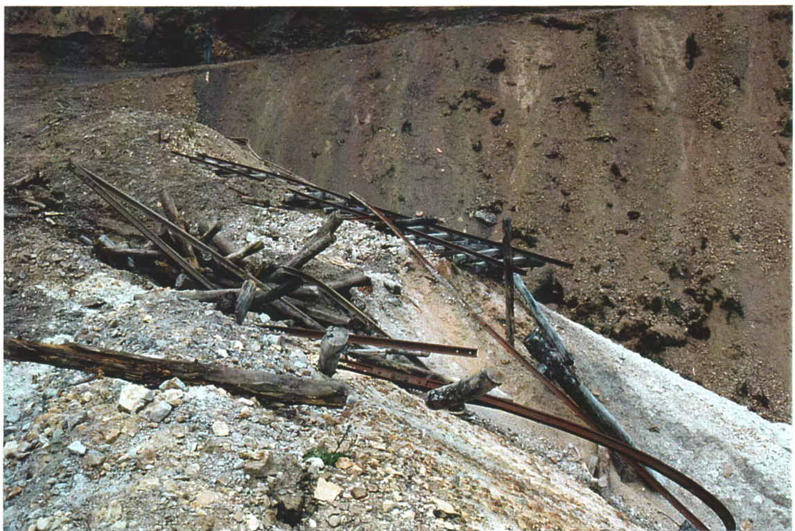
Photo # 2 - Track and Debris
