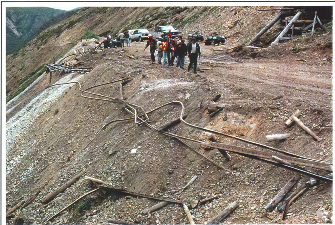
Photo # 3 - Miscellaneous Pipe, Rails and Debris
