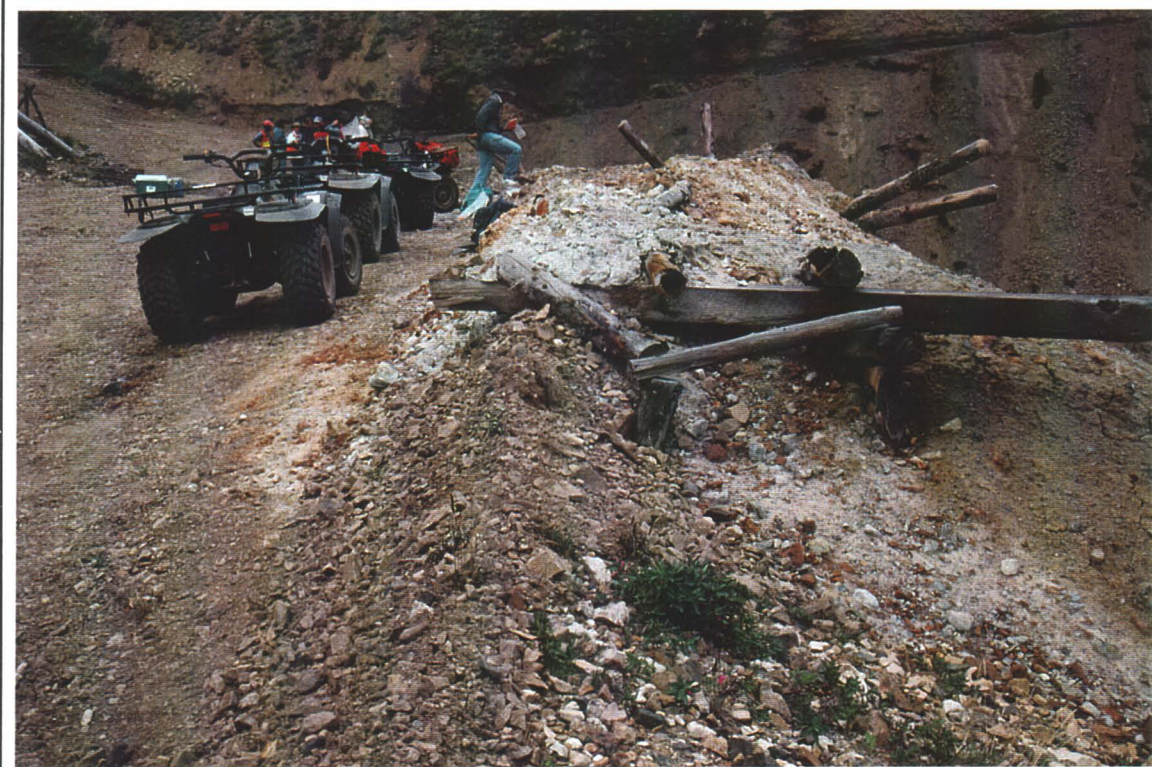
Photo # 4 - Wood Debris
