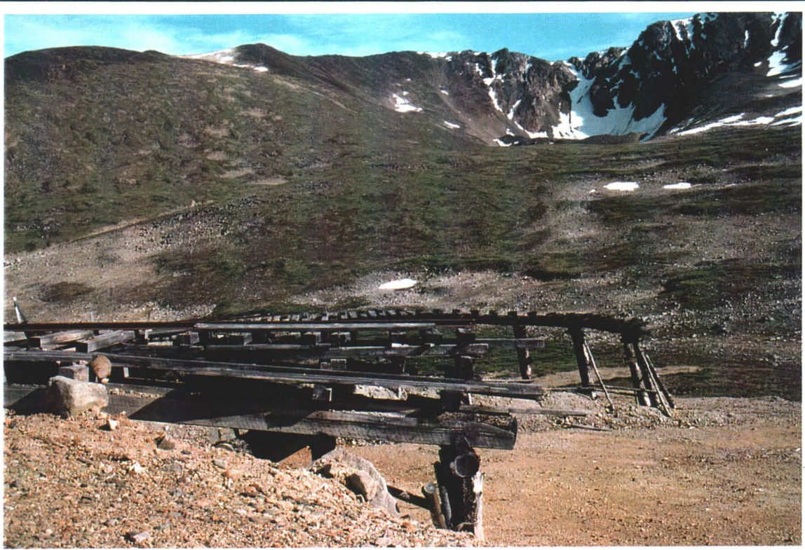
Photo # 23 - Loadout Facilities, Lower Loading Facility
