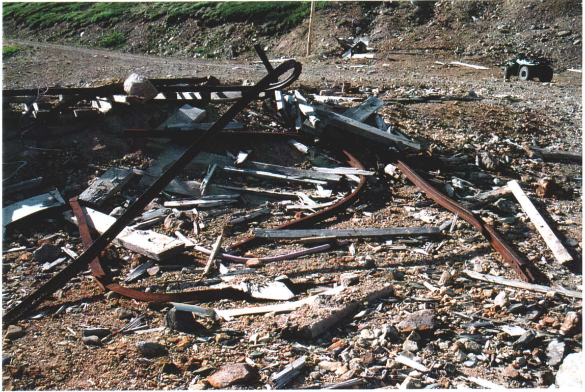
Photo # 29 - Twisted Rails and Debris by Road
