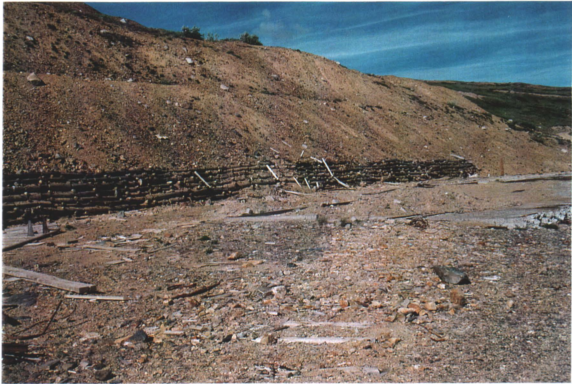
Photo # 7 - Foundations and Debris North of Adit
