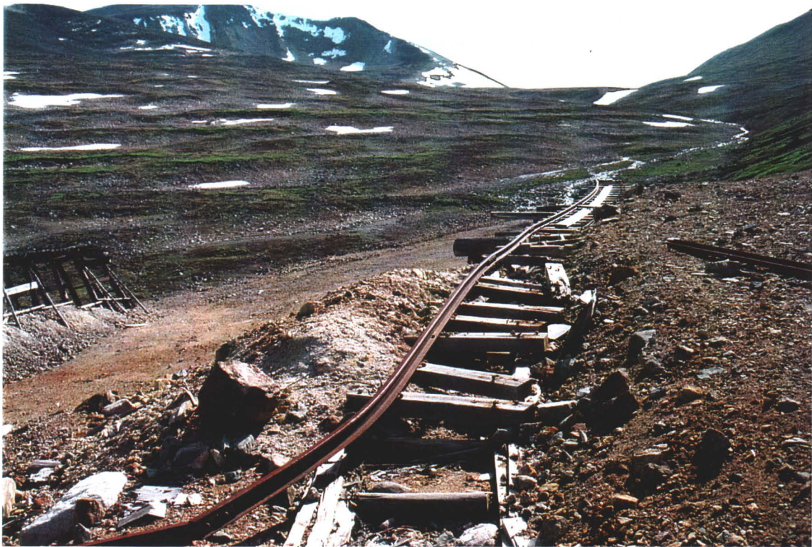
Photo # 22 - Deteriorated Track, Lower Loading Facility
