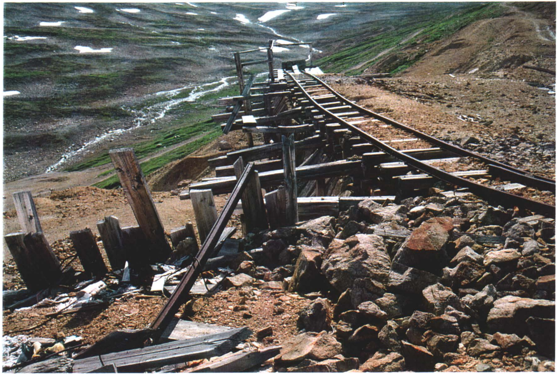
Photo # 13 - Top of Loadout Facility looking South
