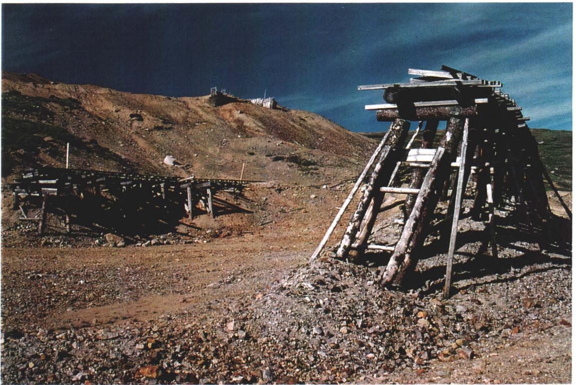
Photo # 24 - Loadout Facilities
