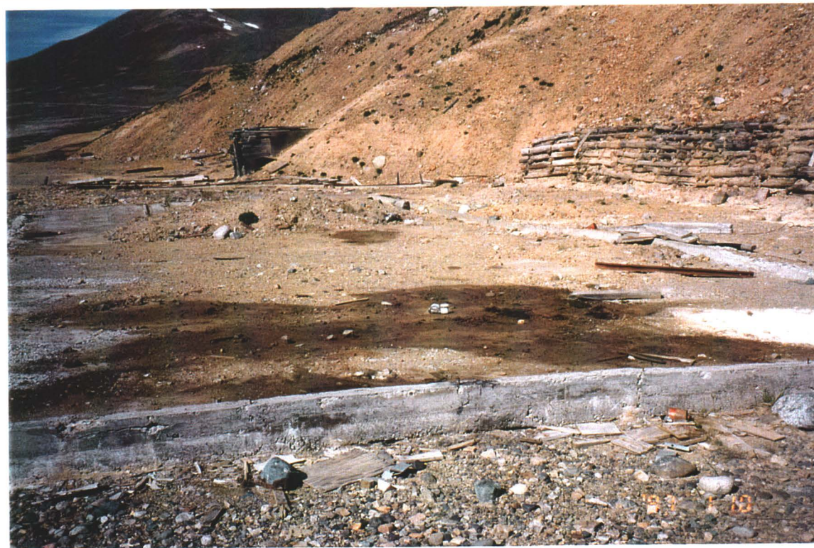
Photo # 45 - Soil Stains on Concrete Pad
