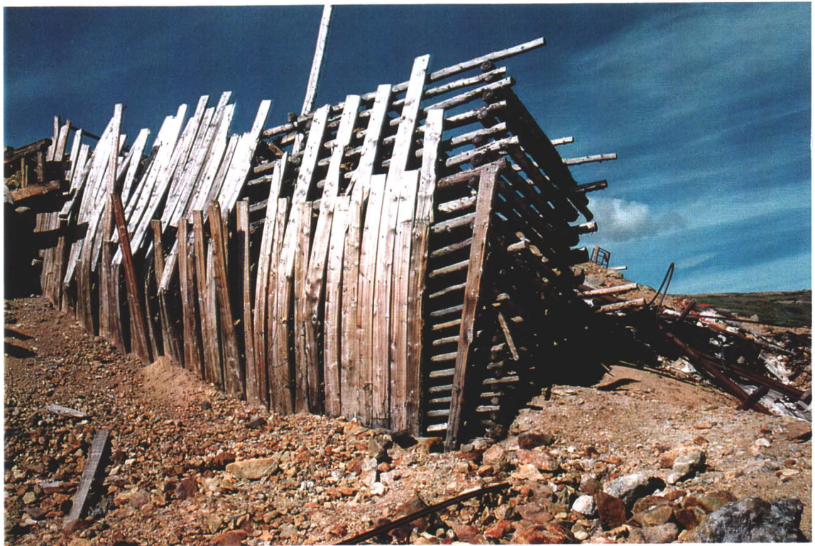
Photo # 10 - Loading Facility - Detail
