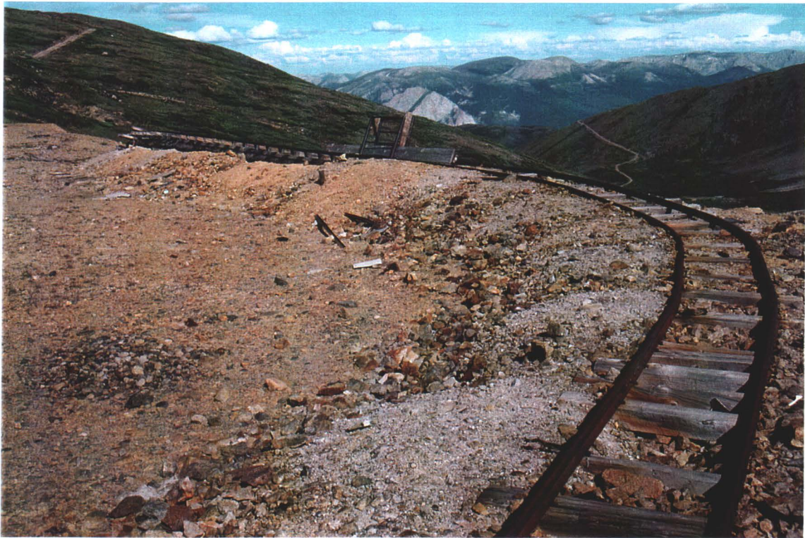
Photo # 8 - Track to Loading Facilities
