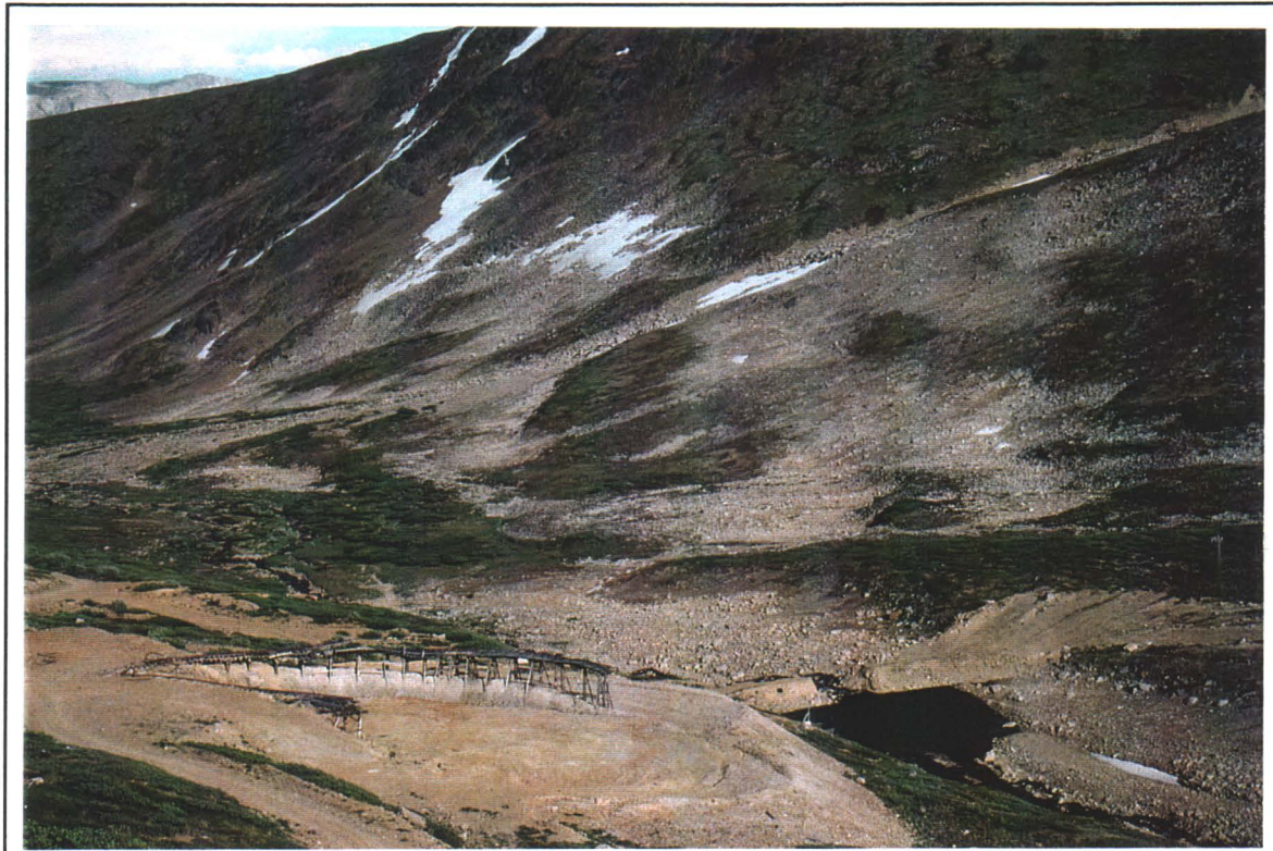
Photo # 32 - Lower Loadout Facility from Upper Drift
