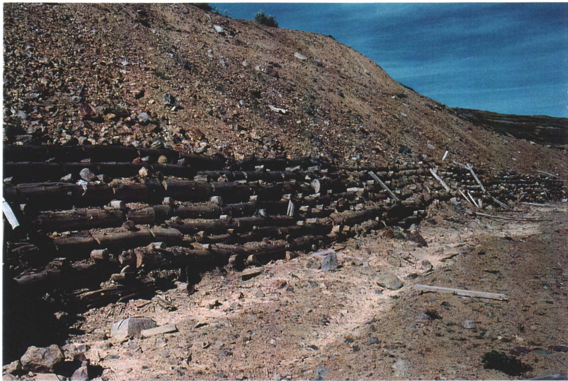
Photo # 5 - Retaining Wall
