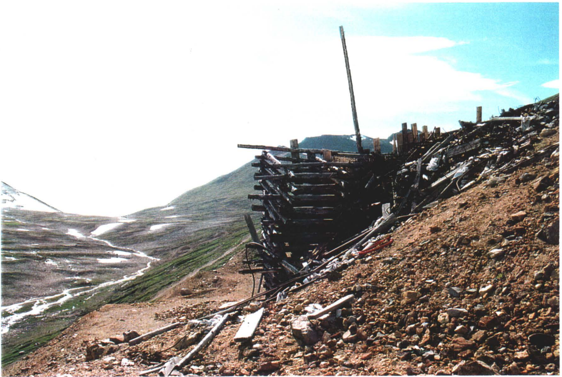
Photo # 16 - Debris by Loadout Facility
