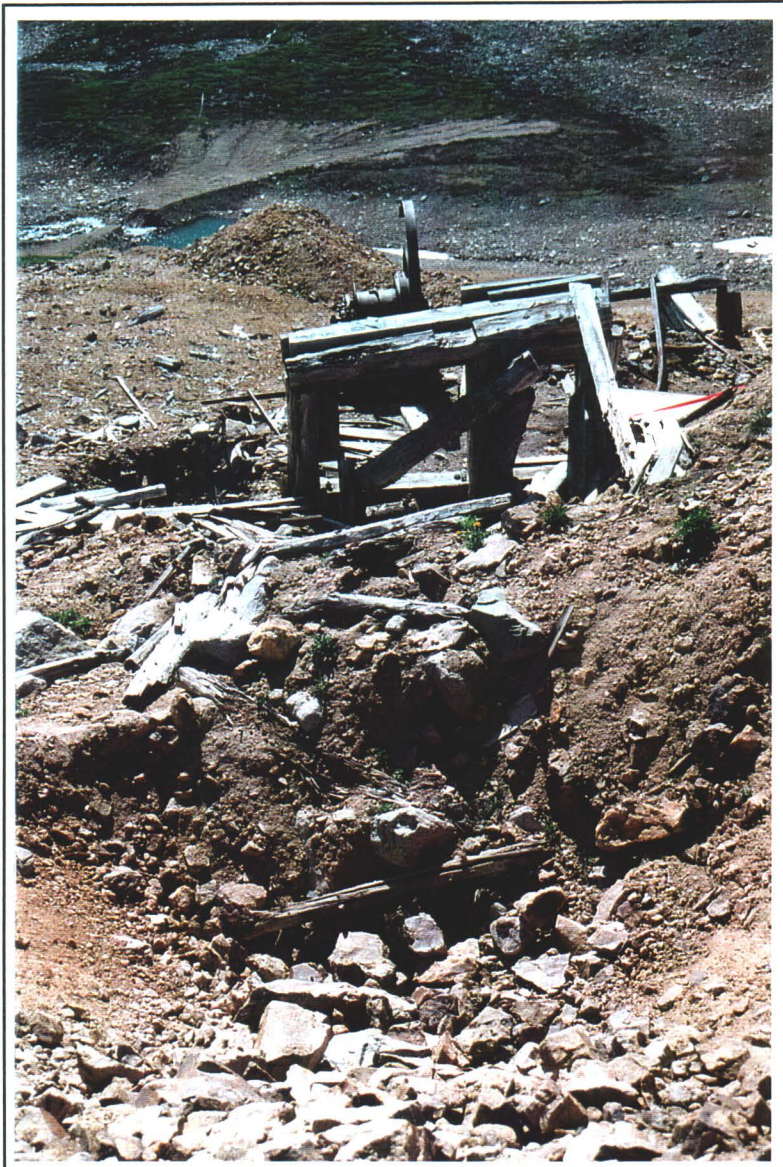
Photo # 34 - Collapsed Upper Drift Site
