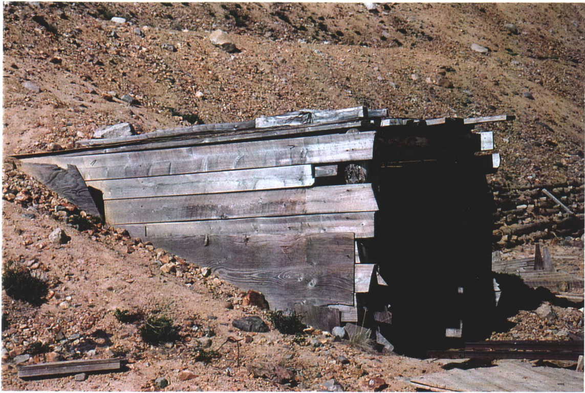
Photo # 1 - Entrance to Middle Adit
