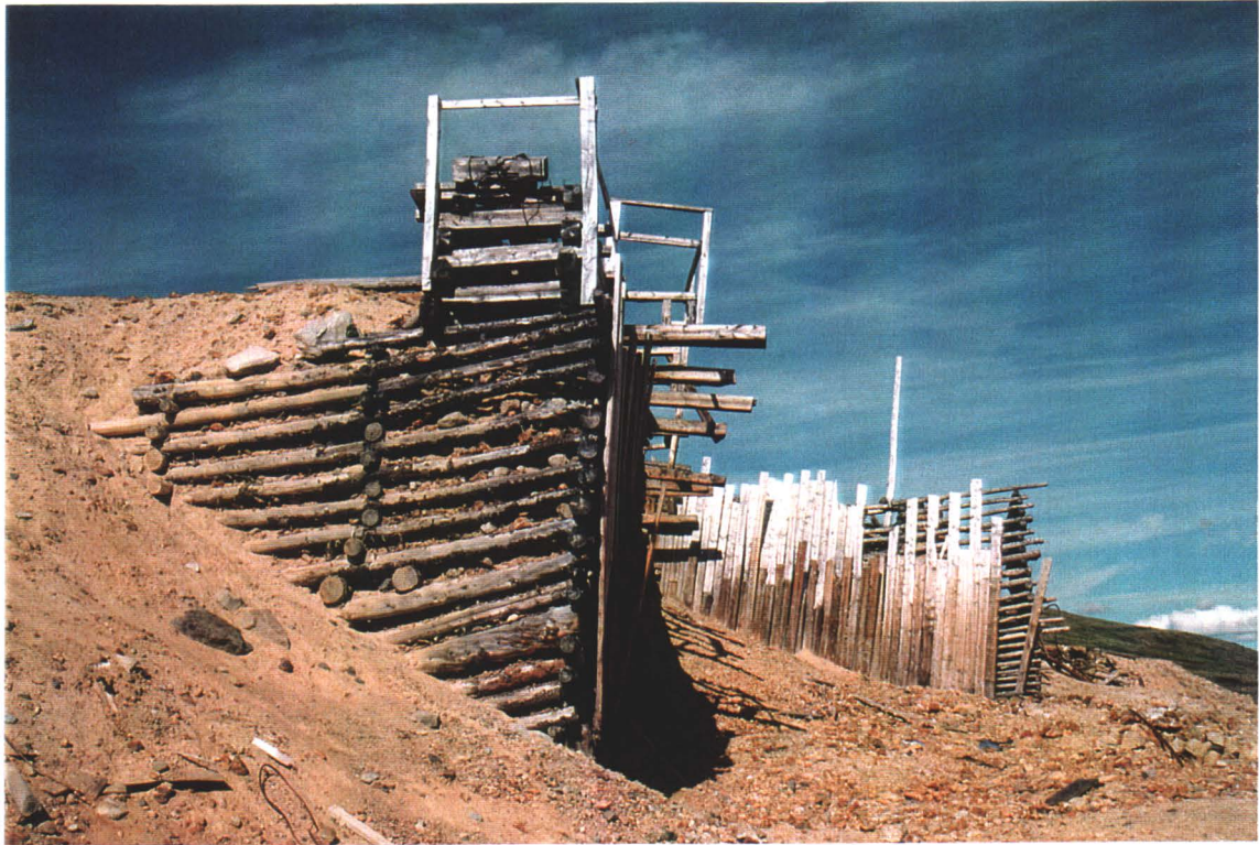
Photo # 9 - Structures Supporting Loadout Facilities, Middle Adit
