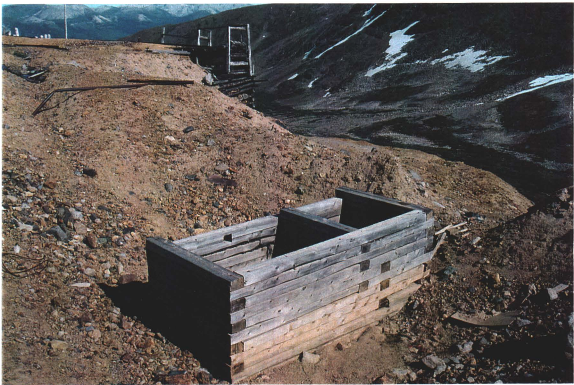
Photo # 6 - Timber Crib
