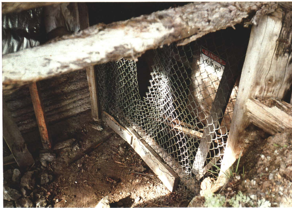
Photo 6. Adit entrance has been screened off and sign posted warning of danger, keep out. Note screen has been cut to allow access.
