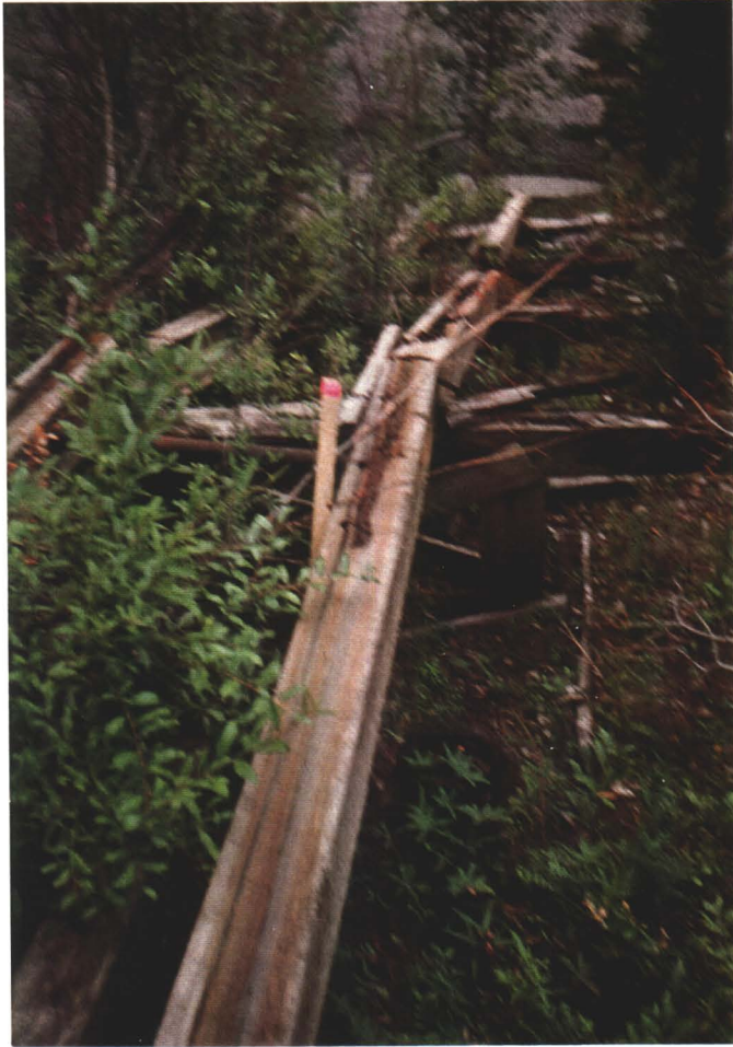
Photo 9. Wooden trestle running up bank above the adit.
