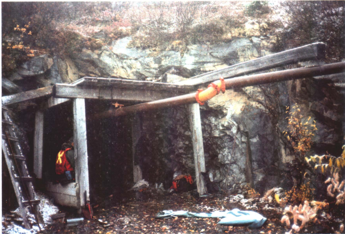
Photo 4: Open adit, suspended compressed air pipe, vent tubing in foreground, looking southwest. September 19, 1996.
