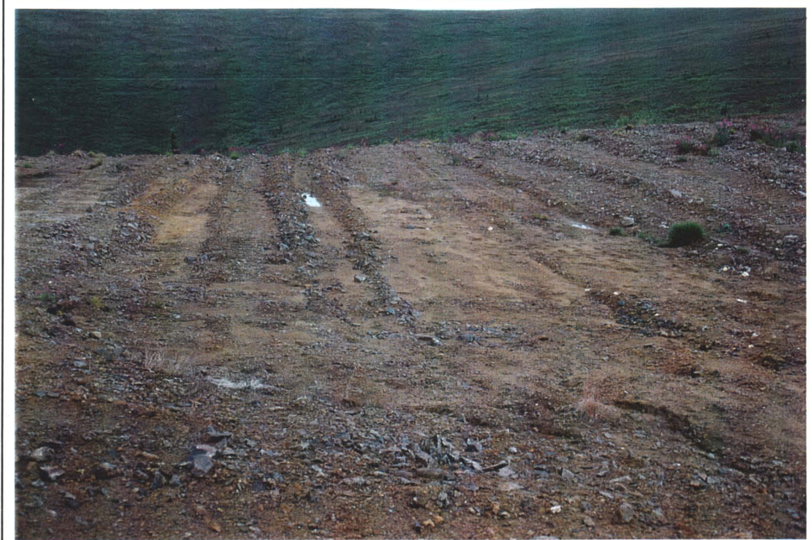
Photo # 6 - View of Stripped Area looking East
