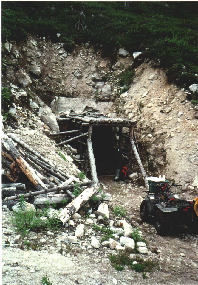
Photo 3. Under built single adit (1.7 m X 2.2 m) built of fir logs.
