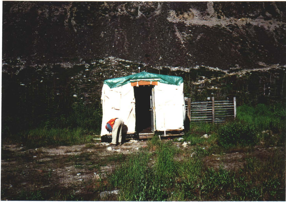
Photo 15. Log structure living quarters covered with tarpaulin (wood floor)
