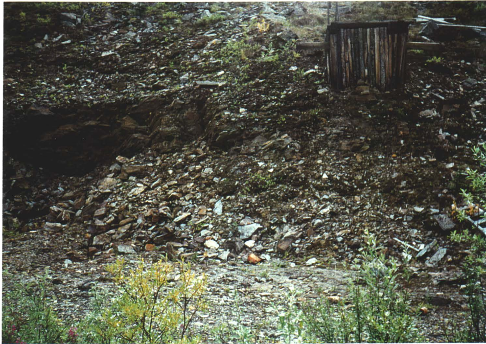
Photo 3. Wood waste upslope and downslope of shaft enclosure and excavation material below shaft entrance.
