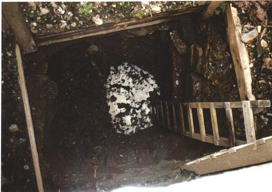
Photo 6. Interior of shaft enclosure with frozen water 3 m below.
