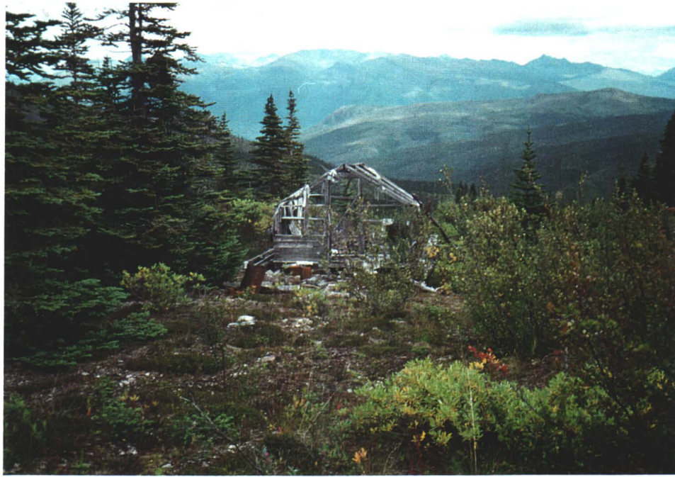
Photo 7. Dilapidated wood tent frame upslope from shaft entrance.
