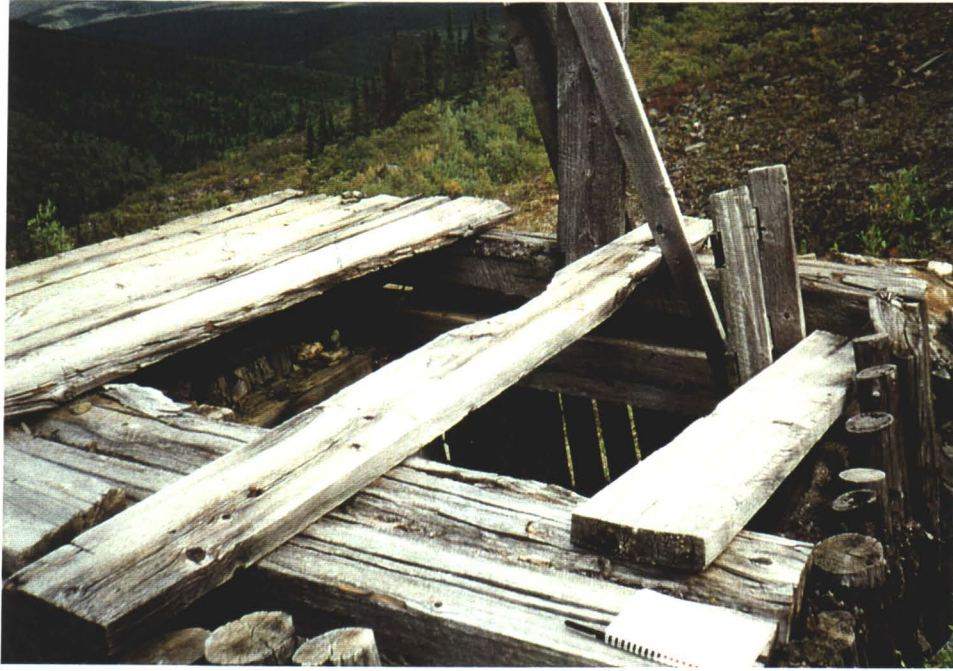
Photo 5. Top of timber shaft enclosure with access ladder at right.
