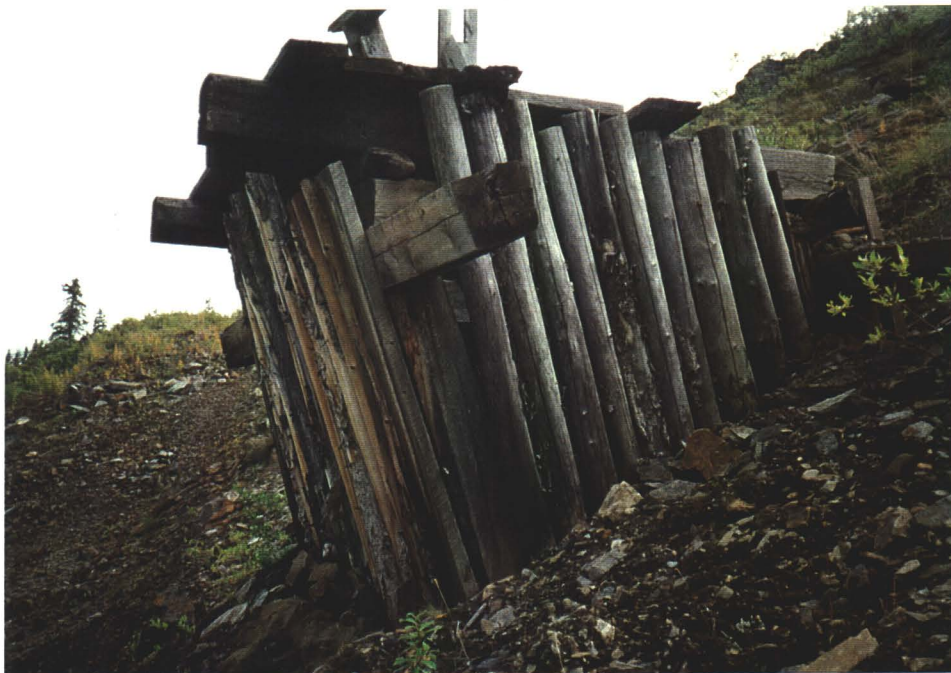
Photo 4. Timber shaft enclosure.
