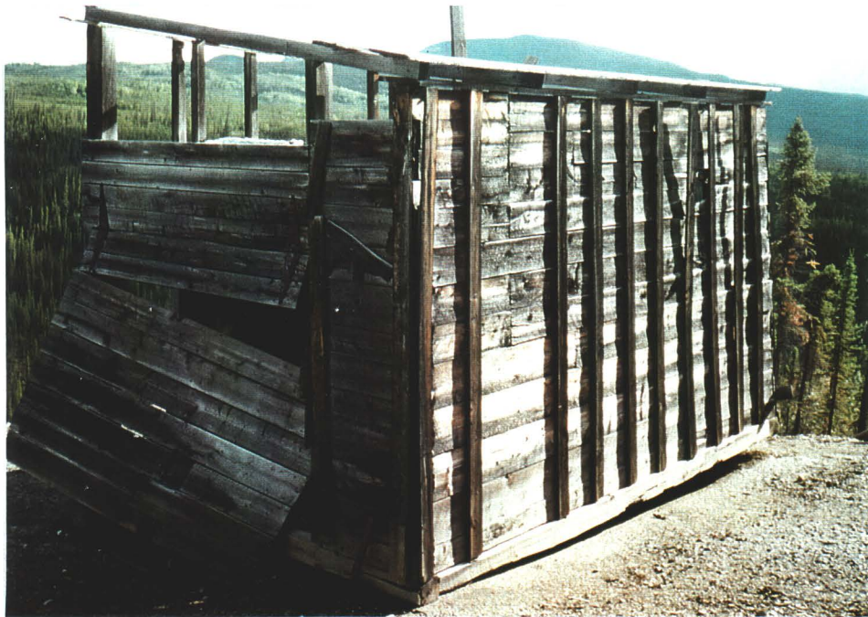
Photo 6. Wood frame wood clad shed at lower adit looking east.
