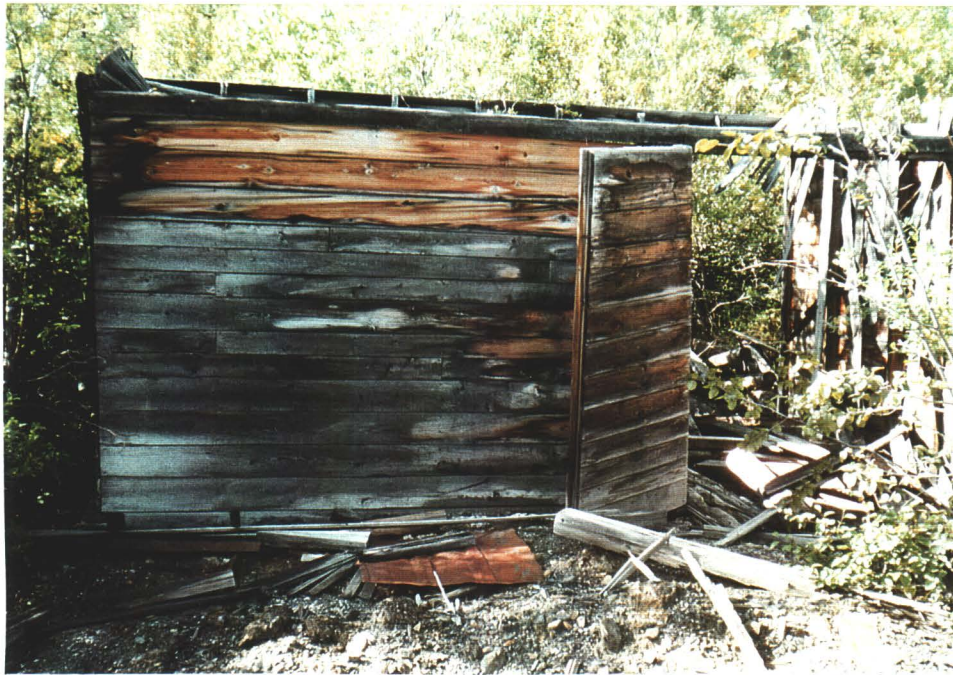
Photo 5. Wood frame wood clad workshop at entrance to lower adit looking southwest.
