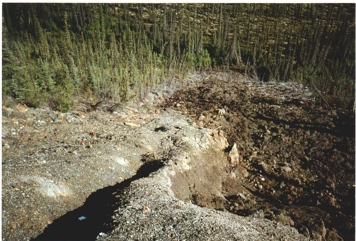
Photo 10. Slumped overburden and waste rock, with recent tension cracks at head of unstable lobe.
