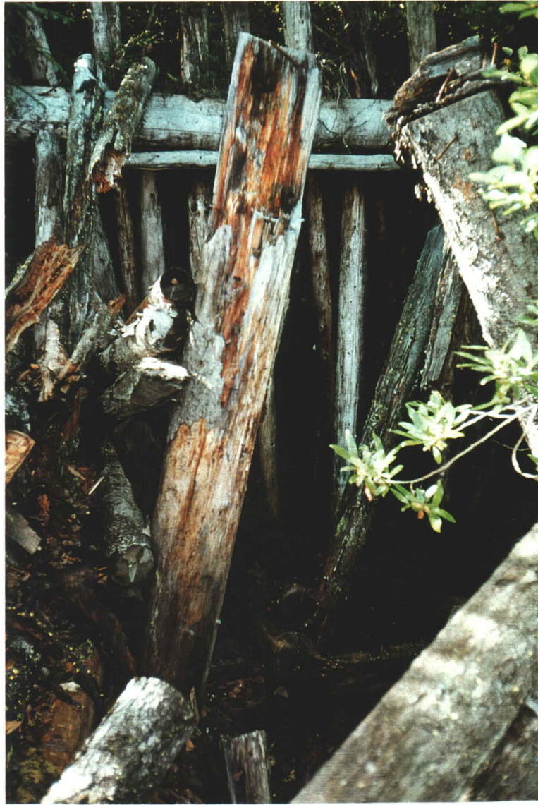
Photo 11. Remnants of log and timber barrier at entrance of lower adit.
