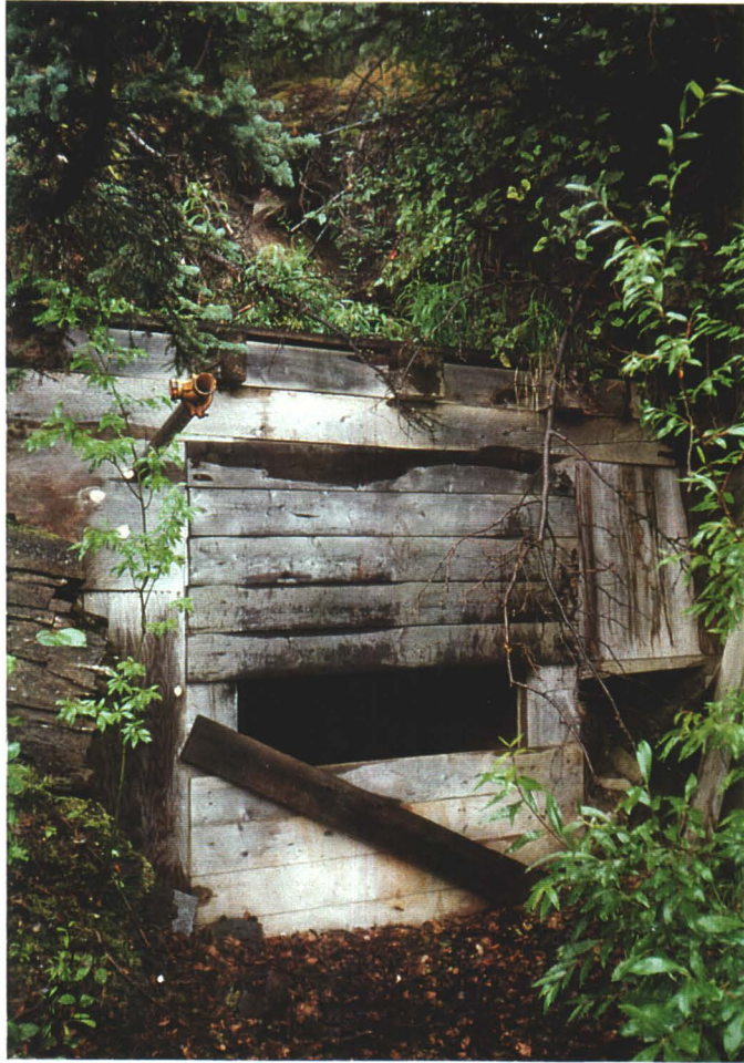
Photo 12. Middle adit enclosure and entrance.
