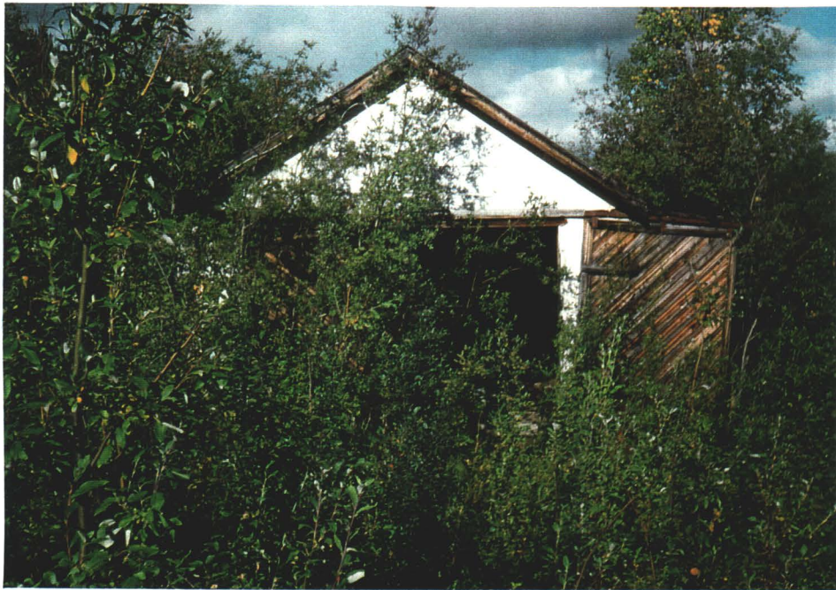
Photo 2. Wood frame wood clad core shed located southwest of upper workings area.
