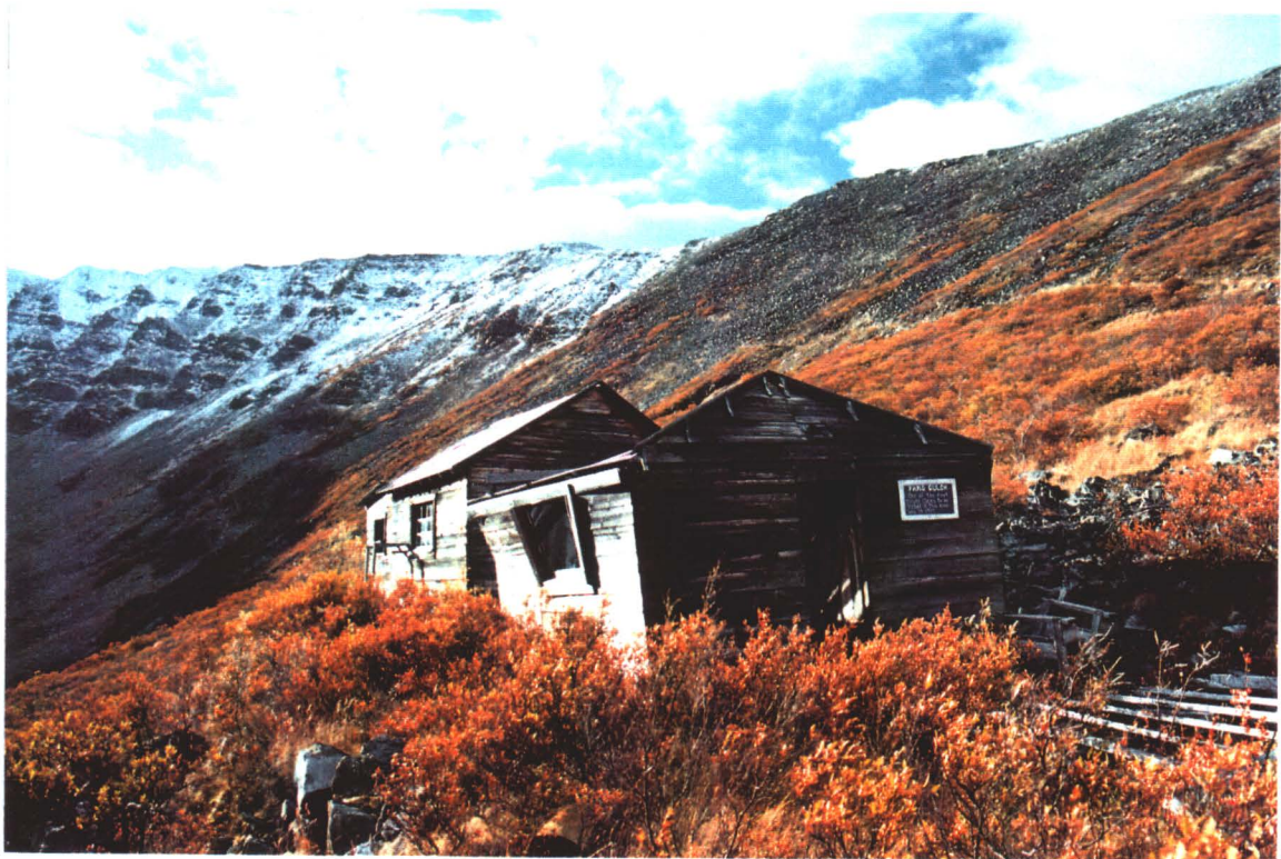
Photo 2: Gambler Mine Site, Main Cabin and partially collapsed cabin looking southwest. September 18, 1996.
