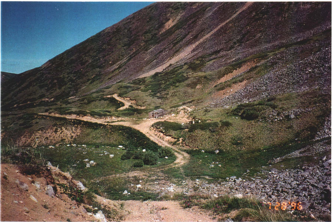
Photo # 6 - Access Road to Camp in Valley below Mine Works
