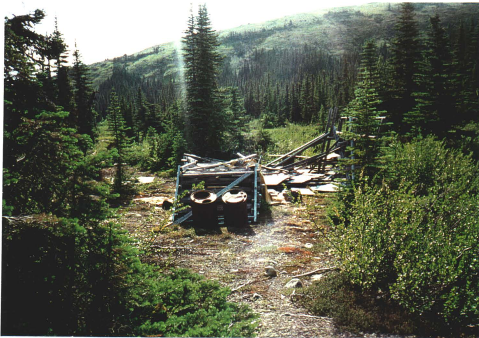
Photo 4. Barrels and wood core storage structure at western edge of site. Note old metal "airtight" stoves.
