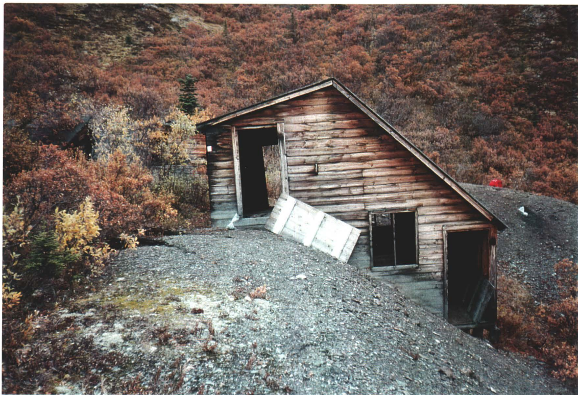
Photo 4: Ore processing building, tool sheds behind trees, looking southwest.
