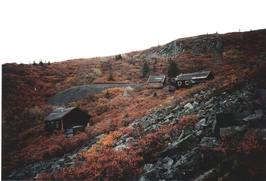
Photo 2: Cabins, tipped outhouse and ore processing building, looking east.
