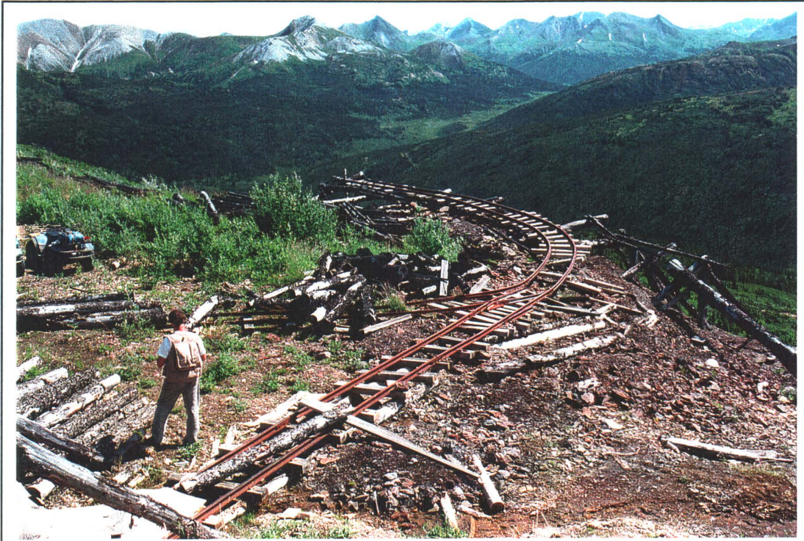
Photo# 7: Track and Trestle - Lower Site
