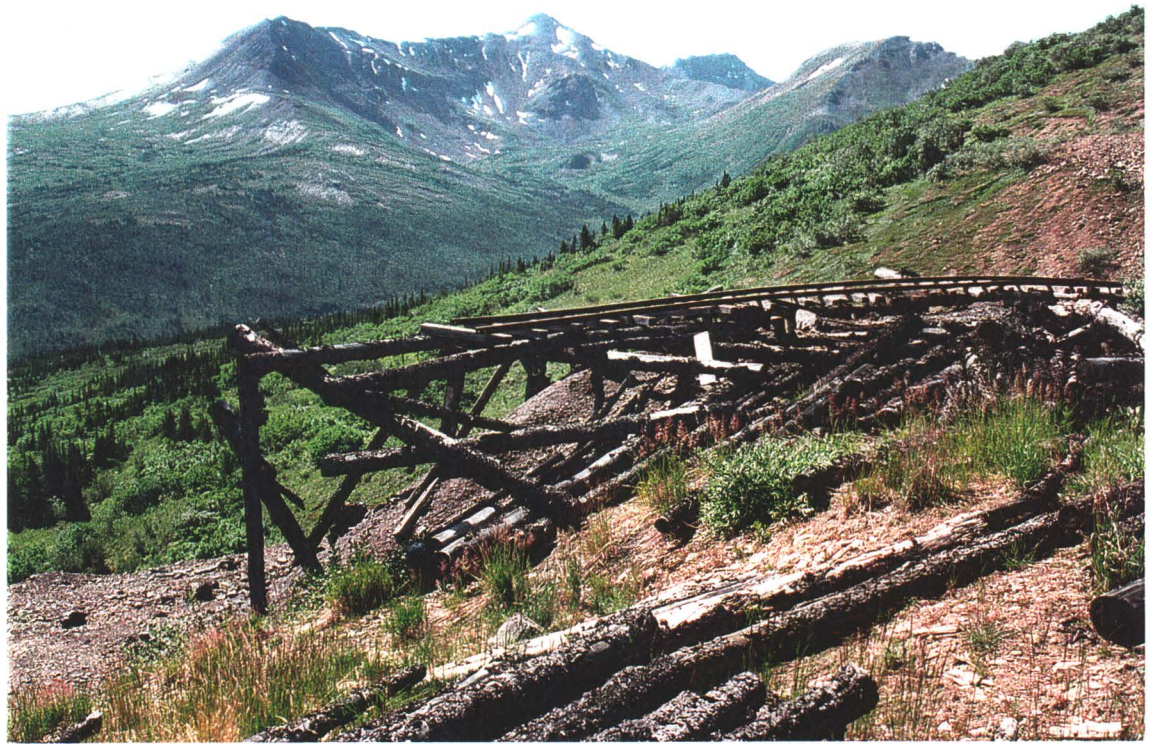
Photo# 8: Track and Trestle - Lower Site
