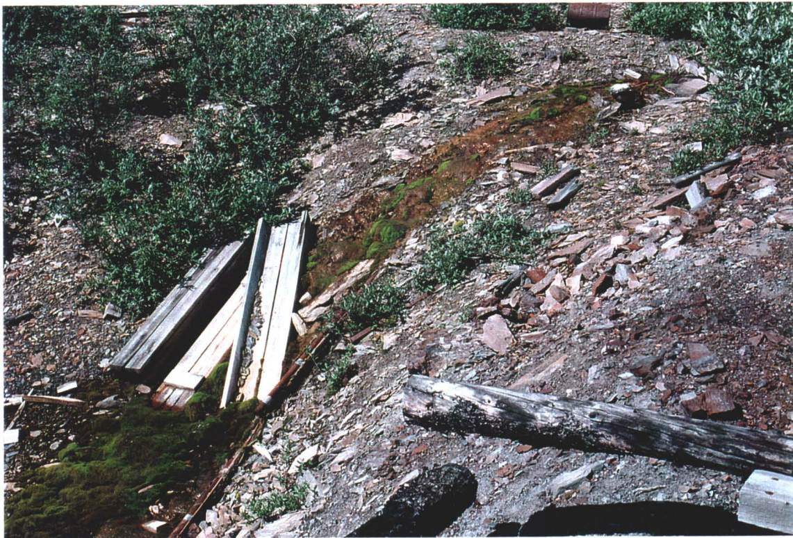
Photo# 10: Mine Water Seepage and Channel - Lower Site
