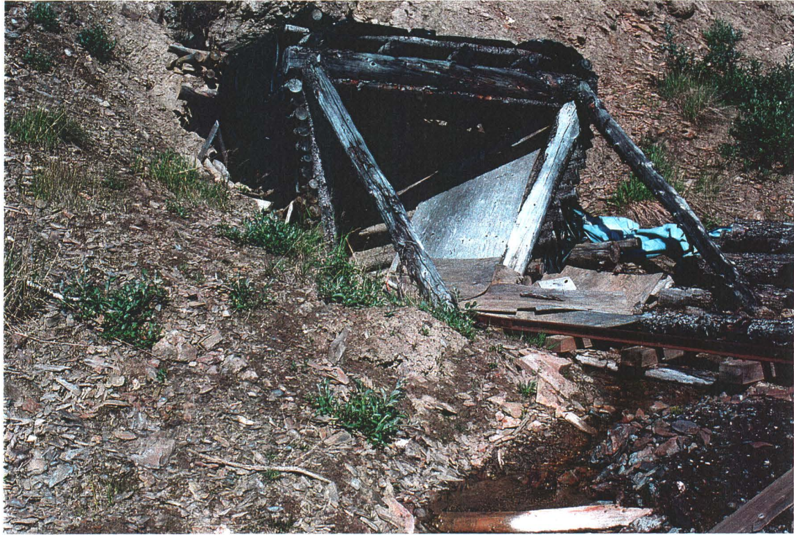
Photo# 5: Lower Adit
