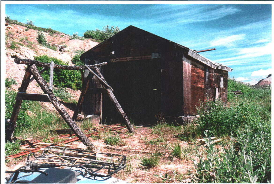
Photo# 3: Processing Building - Lower Site
