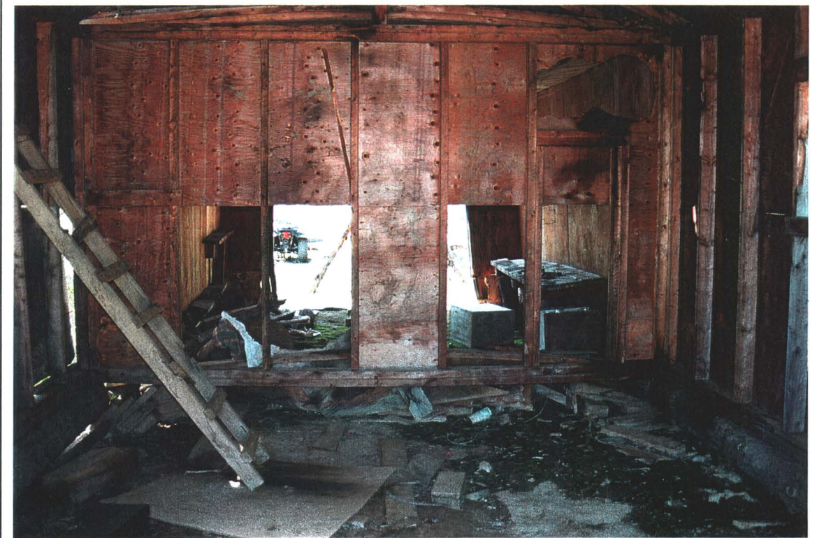
Photo# 4: Interior of Processing Building - Lower Site
