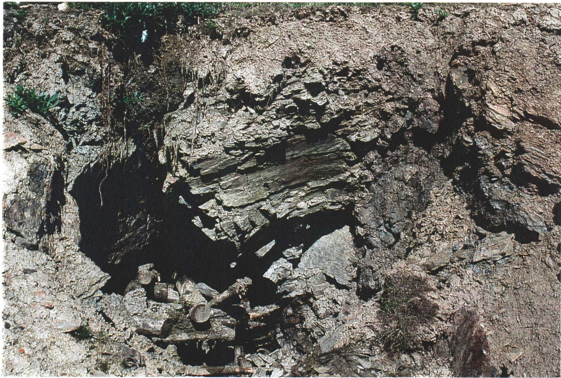
Photo# 6: Sloughing Above Lower Adit
