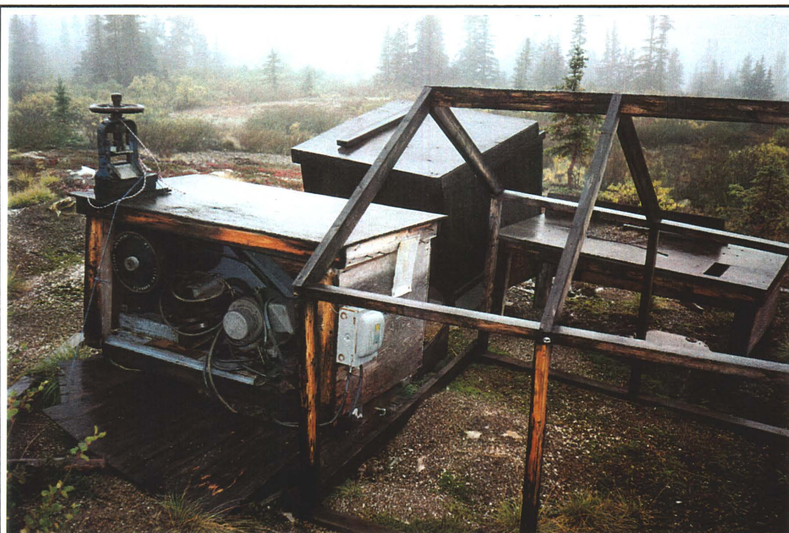
Former generator stand with core splitter.
