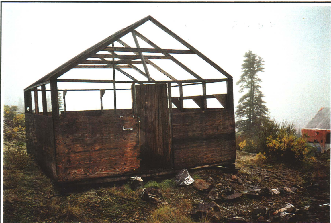
Abandoned housing cabin.
