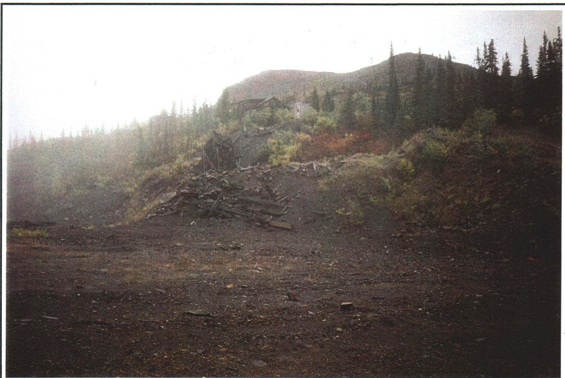
Collapsed mine workings and building structure at centre of camp.
