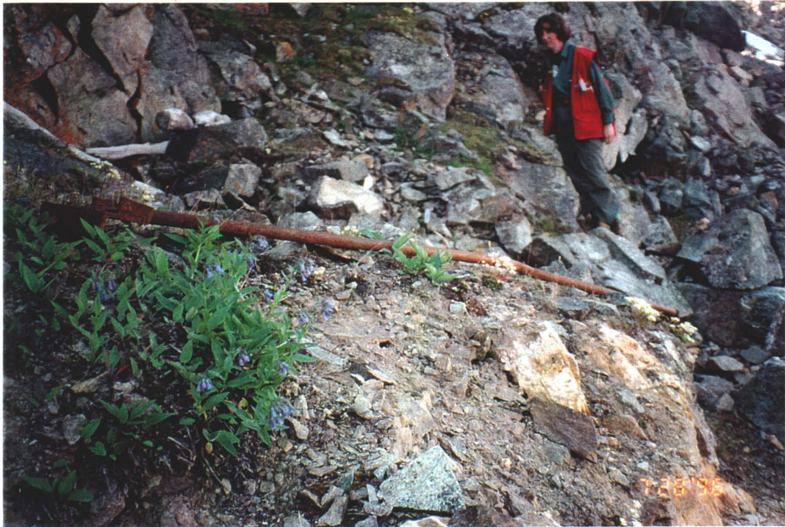
Photo # 3 - Wood and Metal Debris at Adit
