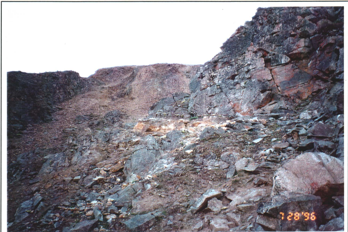
Photo # 5 - Unstable Rocky Slope above Adit
