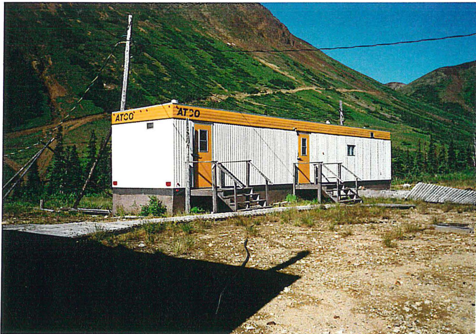
Photo 4. Kitchen trailer with power lines to generator shed.
