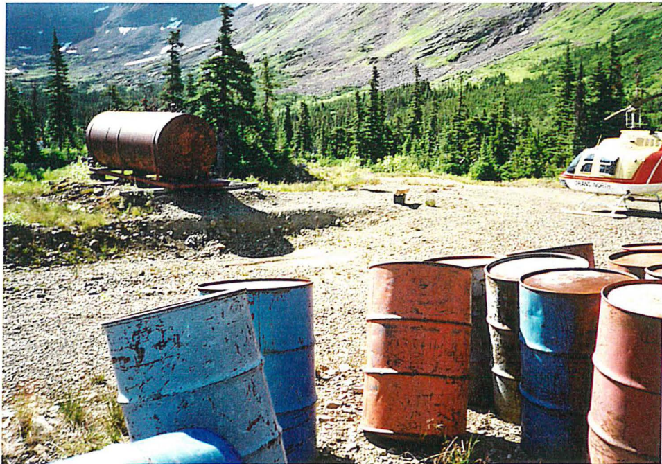
Photo 8. Empty AST with assortment of 205 litre metal barrels previously reported as all empty.
