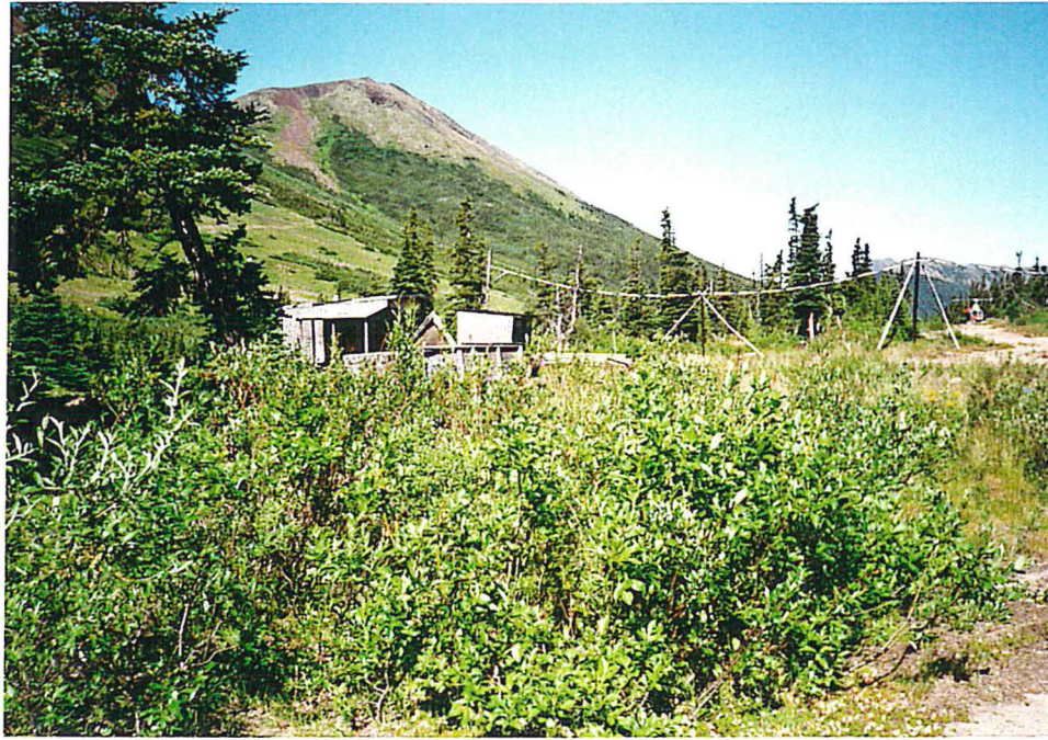
Photo 7. Electrical generator shed with power line to trailer compound visible.
