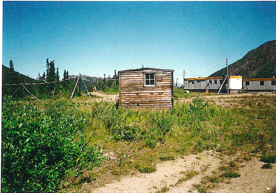
Photo 6. Maintenance shed southwest of trailer compound.
