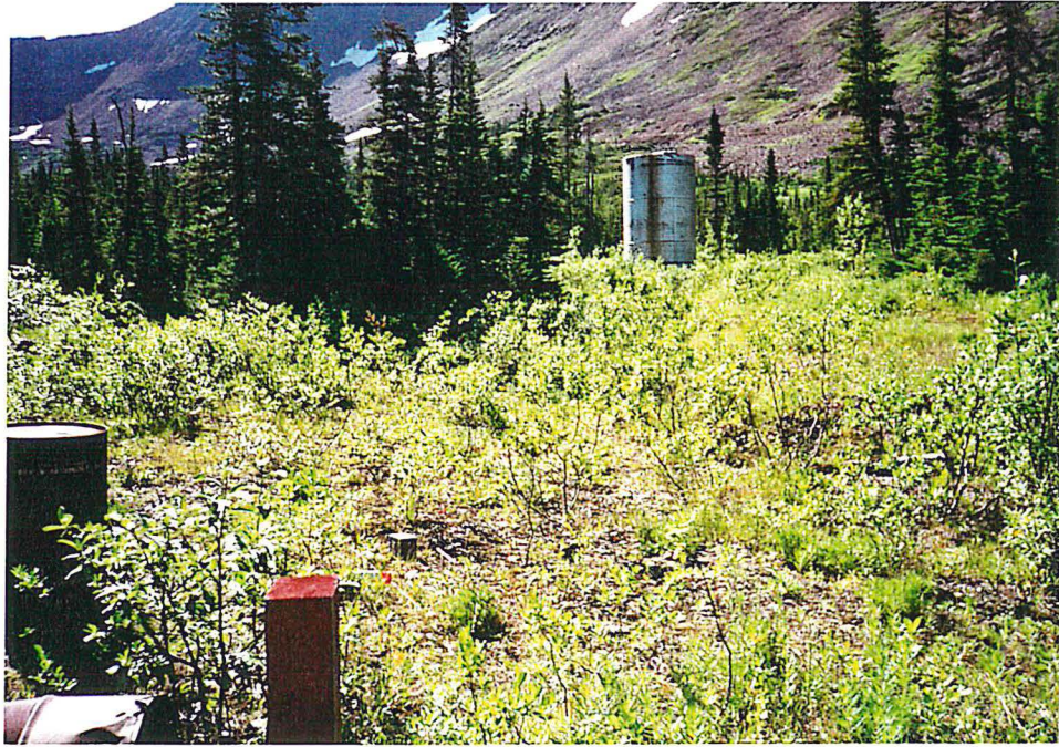
Photo 9. Large vertical AST located approximately 600 m south of trailer camp area.
