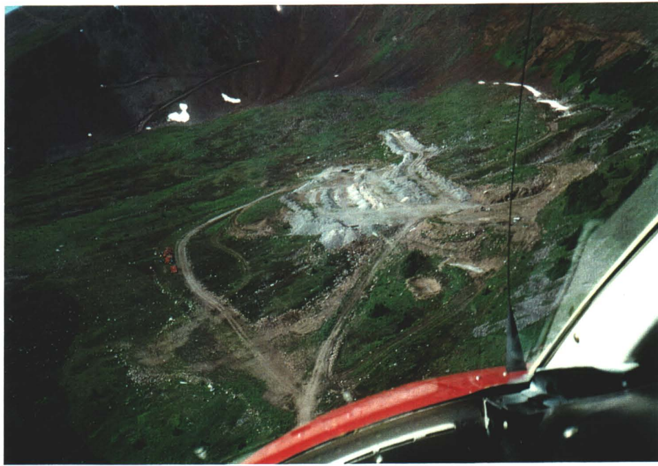
Photo 4. Aerial view of upper exploration area from east with access road to camp area at left. Note barrels by side of access road(left) and adit at right.
