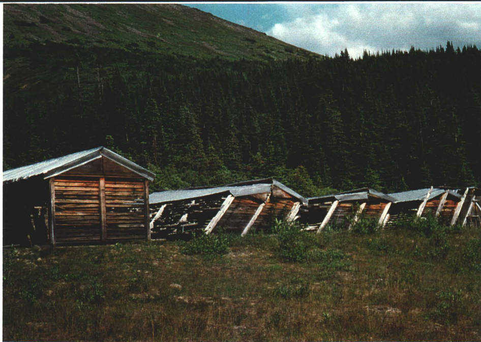
Photo12. Collapsing wood frame core sheds at lower camp level. Shed at left is only partially filled with core while other sheds have had core placed on upper racks.
