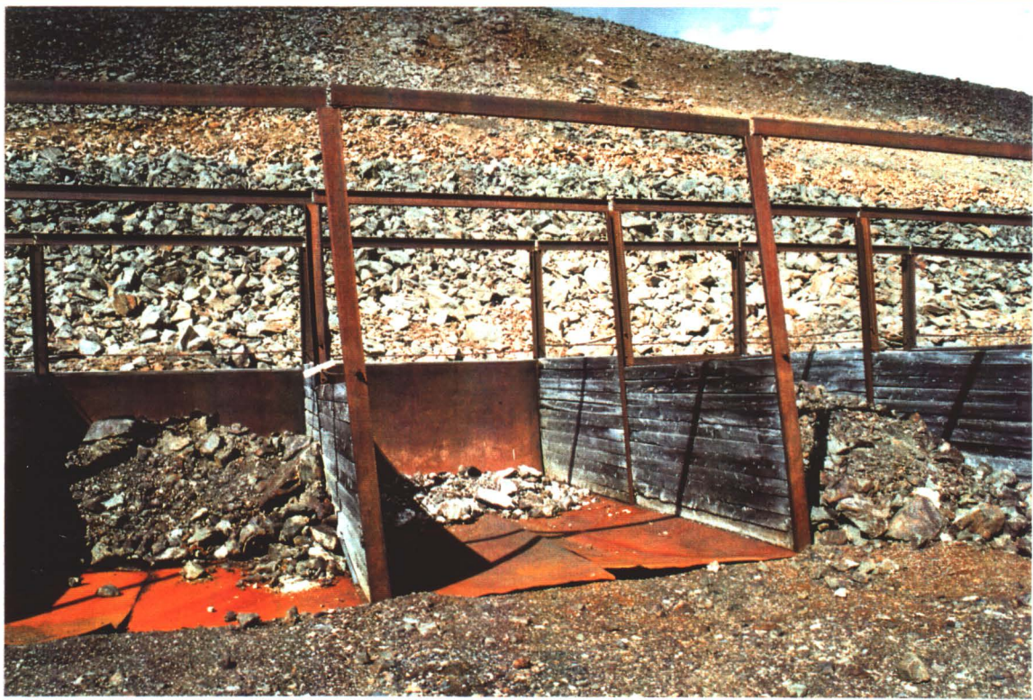
Photo 10. Ore bins constructed from steel I-beams, sheet steel back walls and floors, and timber side walls.
