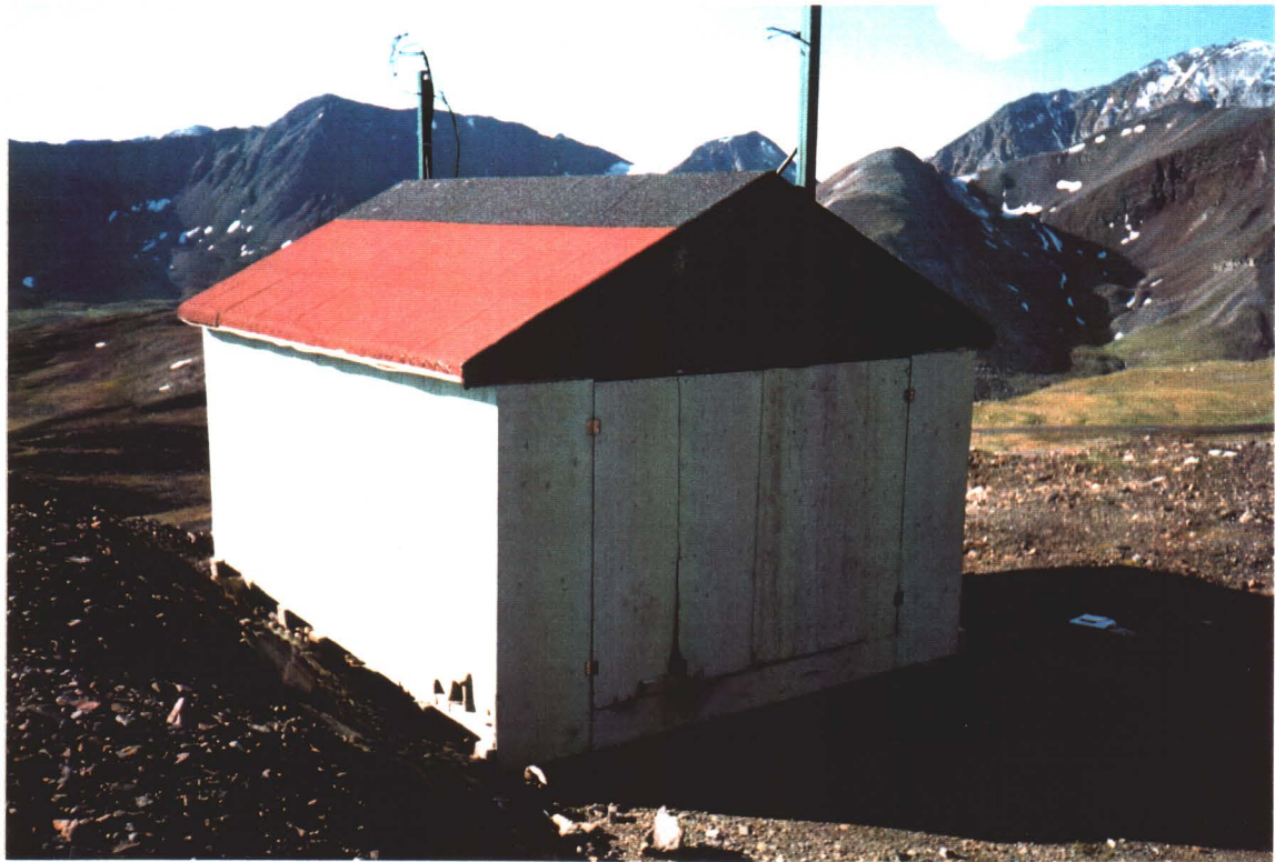
Photo 7. Generator shed, looking southwest.
