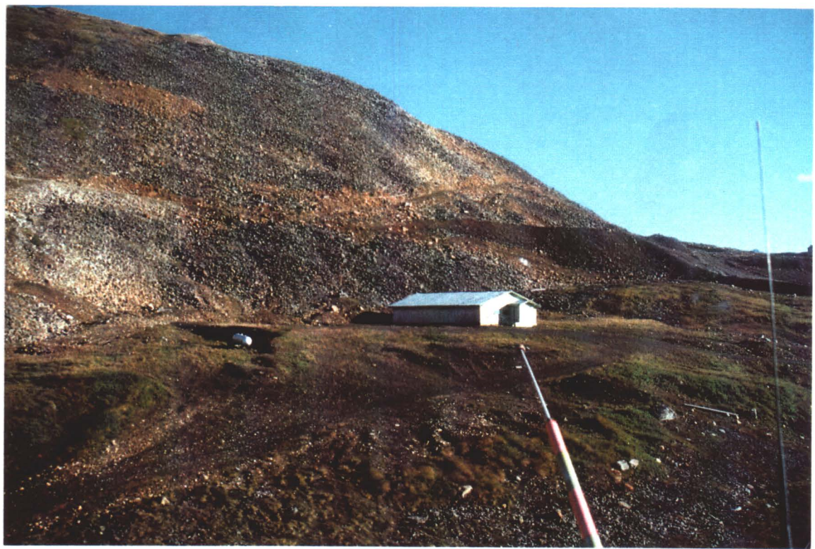
Photo 4. Core shed and propane tank.
