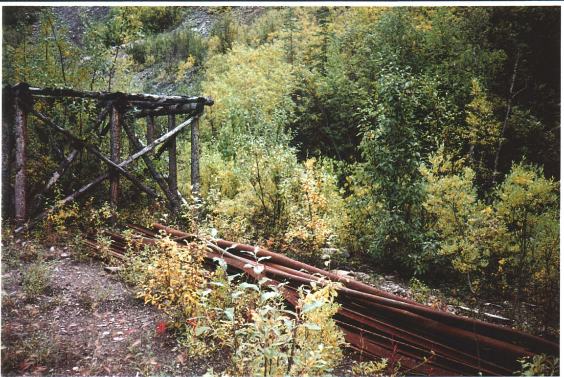
View of piping abandoned along Lower Road.
