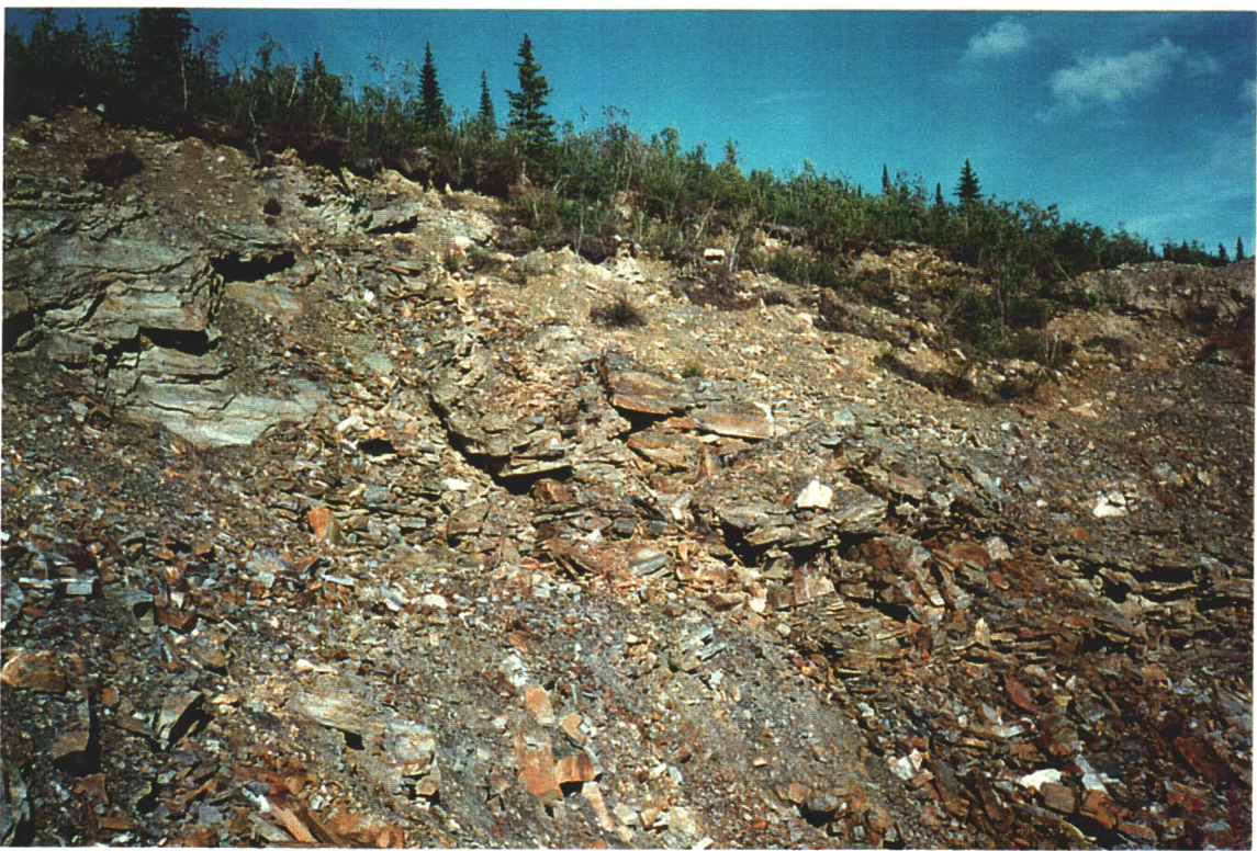
Photo 18. View of upper workings looking northeast. Note evidence of undercut (left side of photo) and rotational slumping (right side) along vegetated edge of workings.
