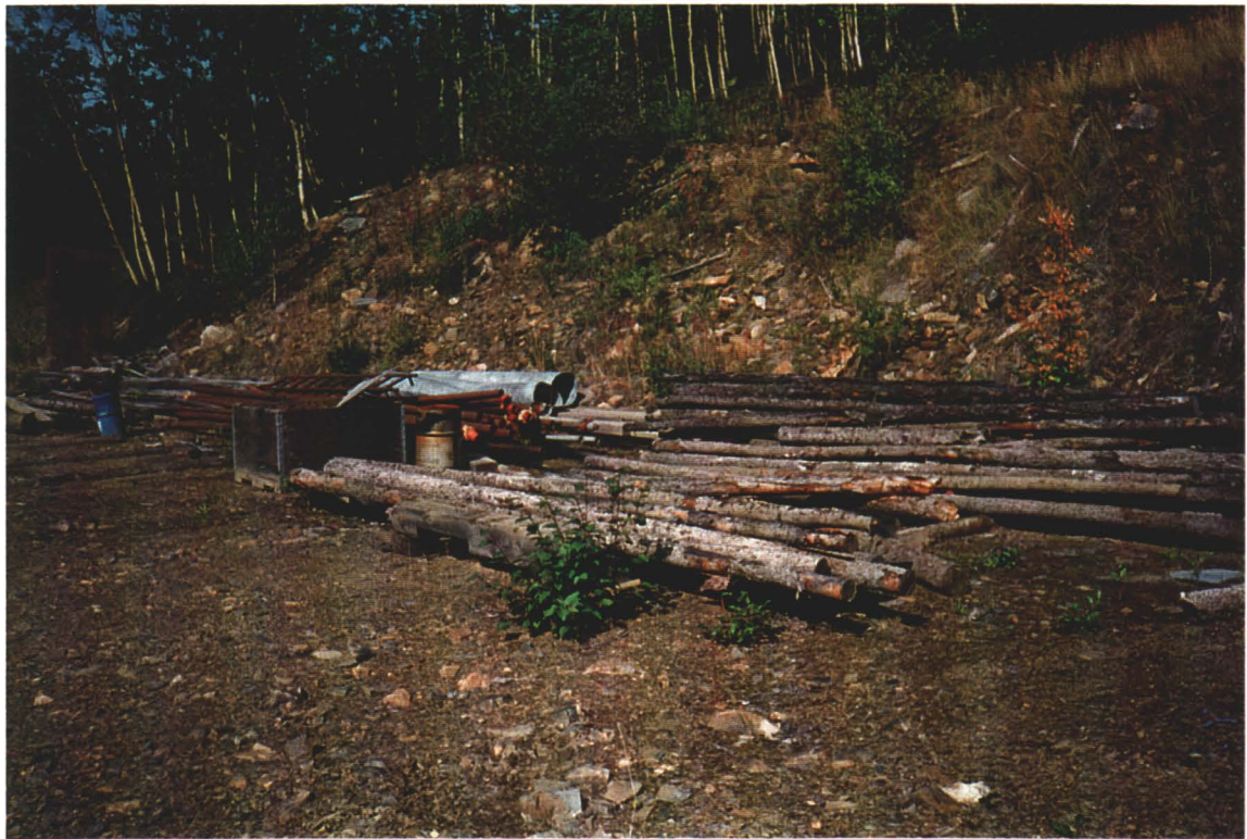
Photo 9. Material laydown area west of storage shed, viewed toward northwest.
