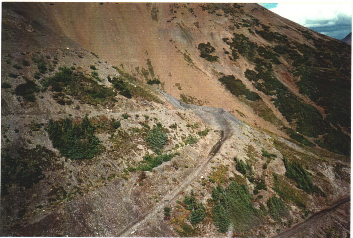
Photo 4. Access road to upper level trenches; seep visible as wet patch on the road near the centre of the photo.
