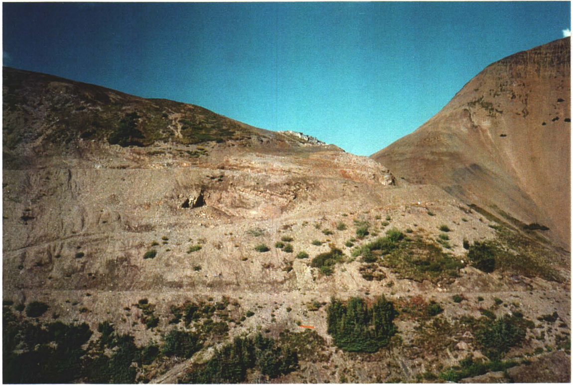
Photo 3. Upper level trenching; excavation face visible near centre of photo.
