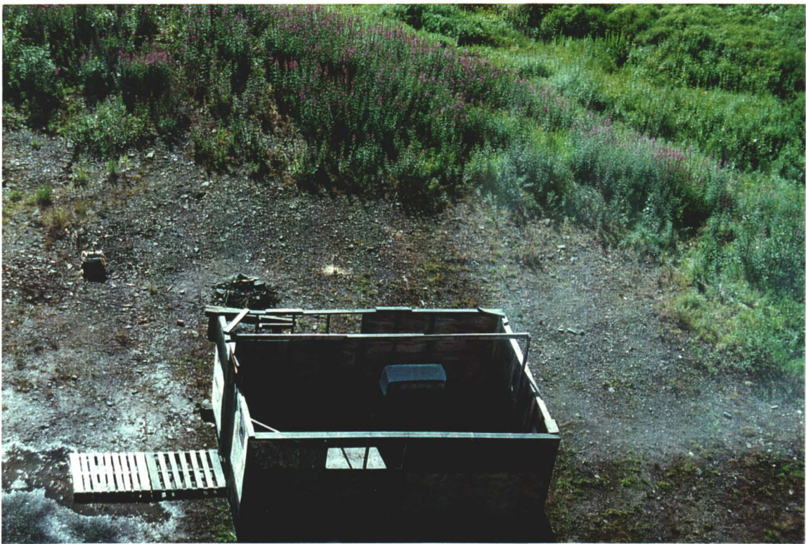
Photo 6. Cabin on mine access road.
