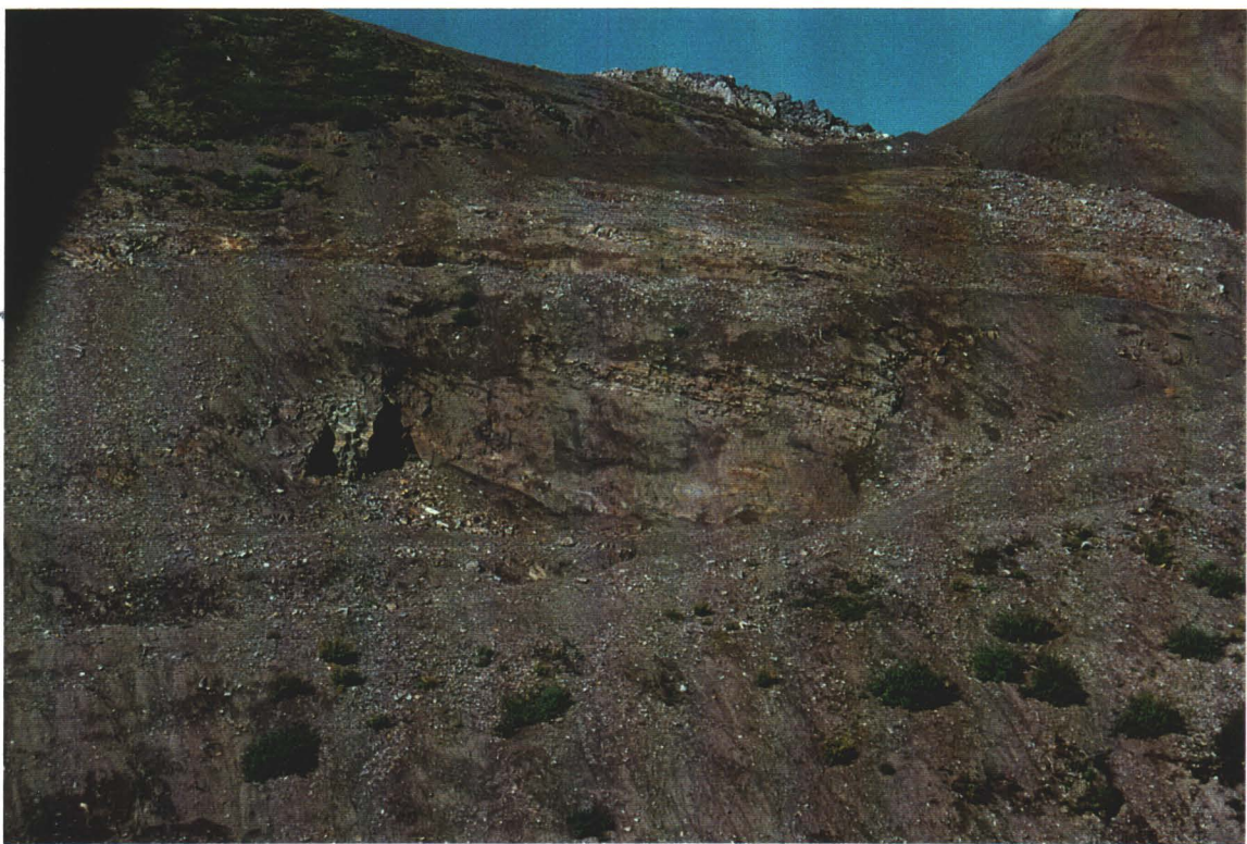
Photo 2. Excavation in upper trench area.
