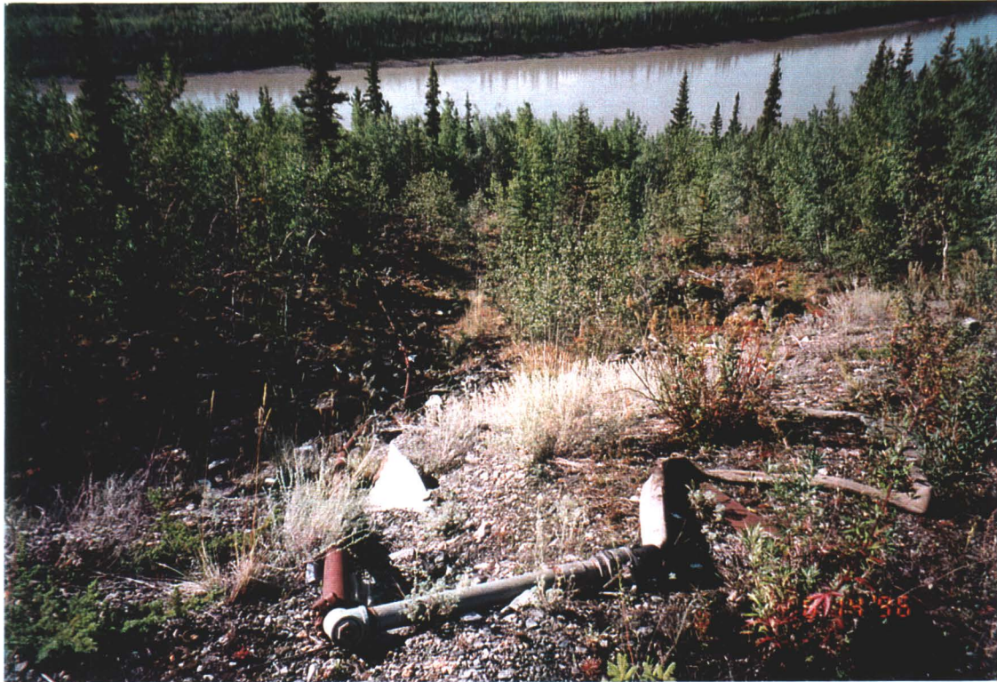
Photo # 5 - Top End of Steel Pipe Leading down Mountainside
