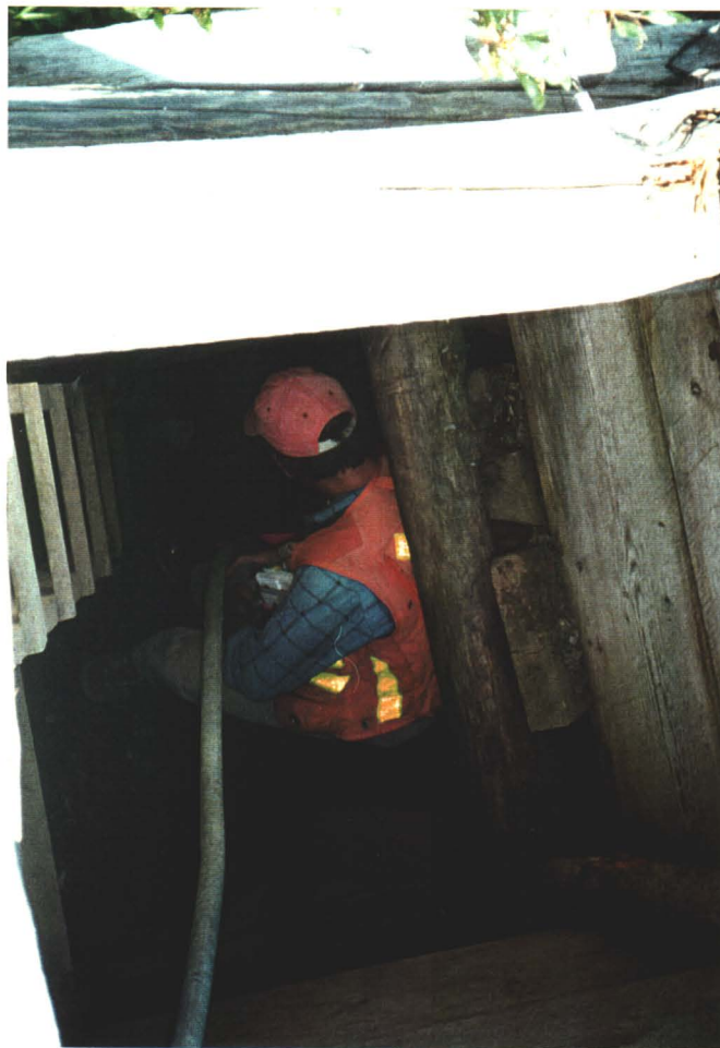
Photo 12. Inspecting interior of upper level raise.
