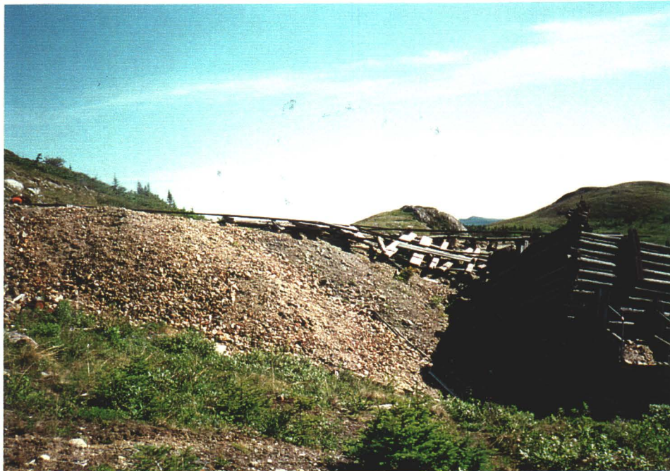
Photo 2. Trestle on top of waste rock leading to log framed ore bin at right.
