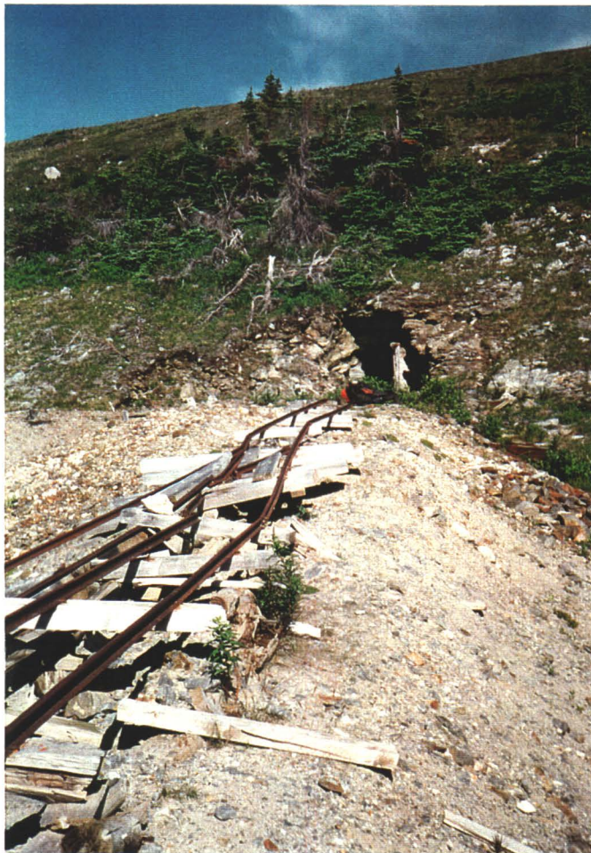
Photo 3. Rusted metal track running from adit entrance along waste rock escarpment.
