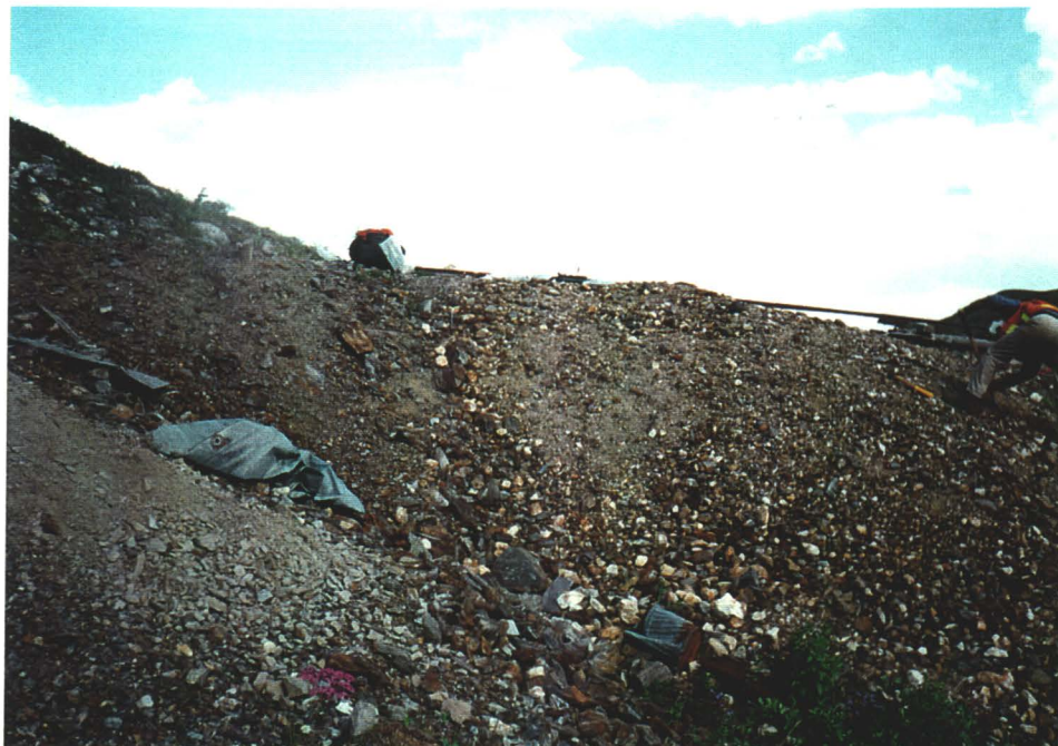
Photo 6. Excavating on west side of trestle for waste rock samples.
