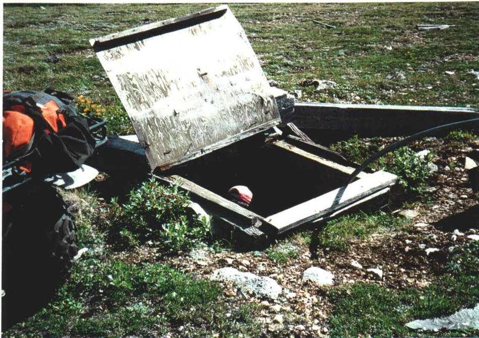
Photo 11. Entrance to upper level raise with plywood cover attached.
