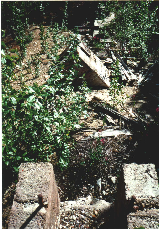
Photo 14. View down slope from access road to foundations of former Silver Seven mill site..
