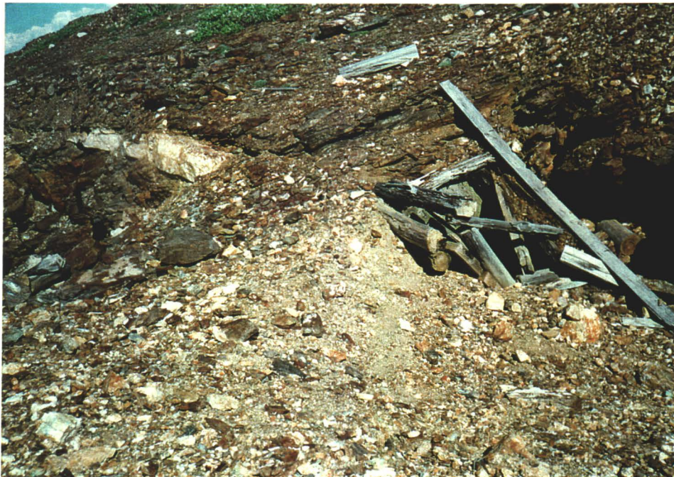
Photo 10. Collapsed shaft found in upper trenching area.
