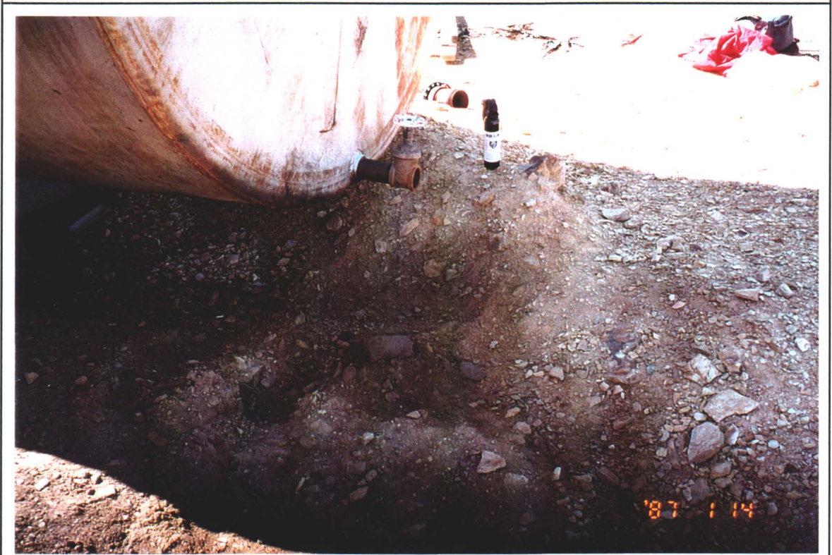
Photo # 2 - Stained Soil adjacent to Large Storage Tank
