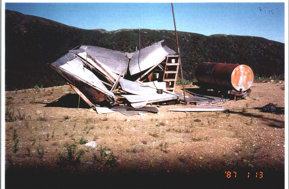
Photo # 4 - Demolished Generator Shack and Storage Tank
