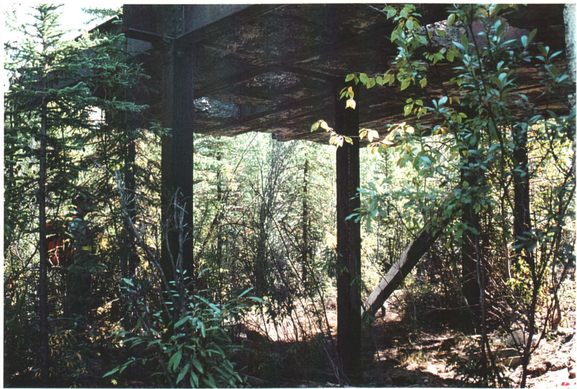
Photo # 17 - Powerhouse Structure
