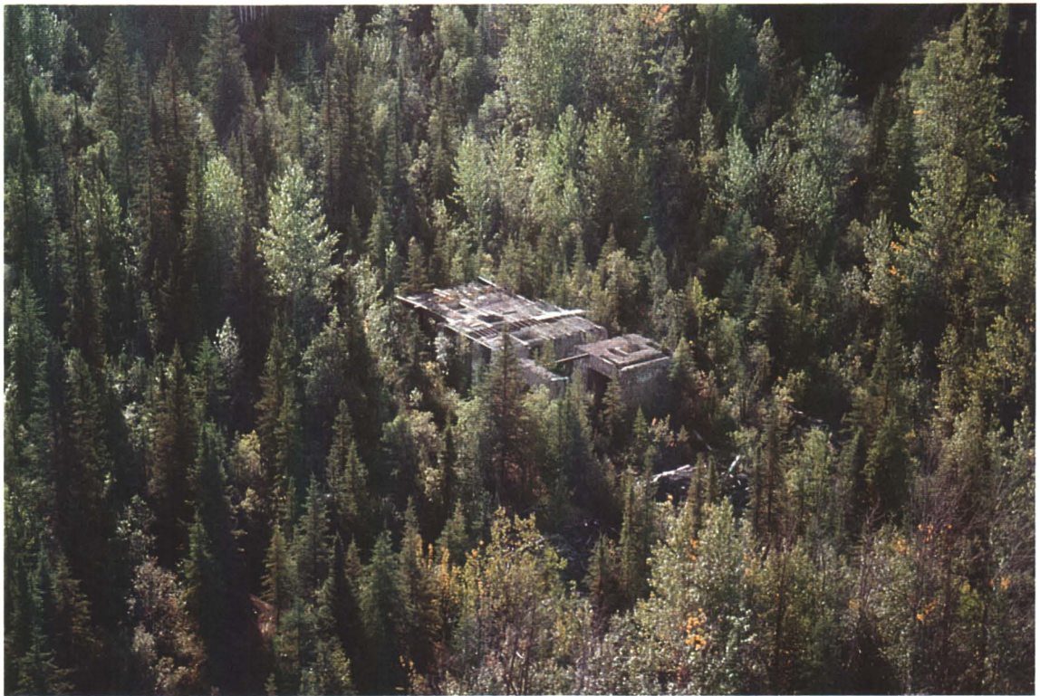
Photo # 15 - View of Powerhouse from southeast
