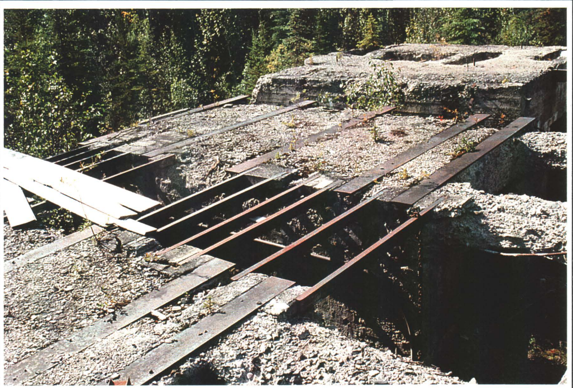
Photo # 18 - Top of Powerhouse Facility
