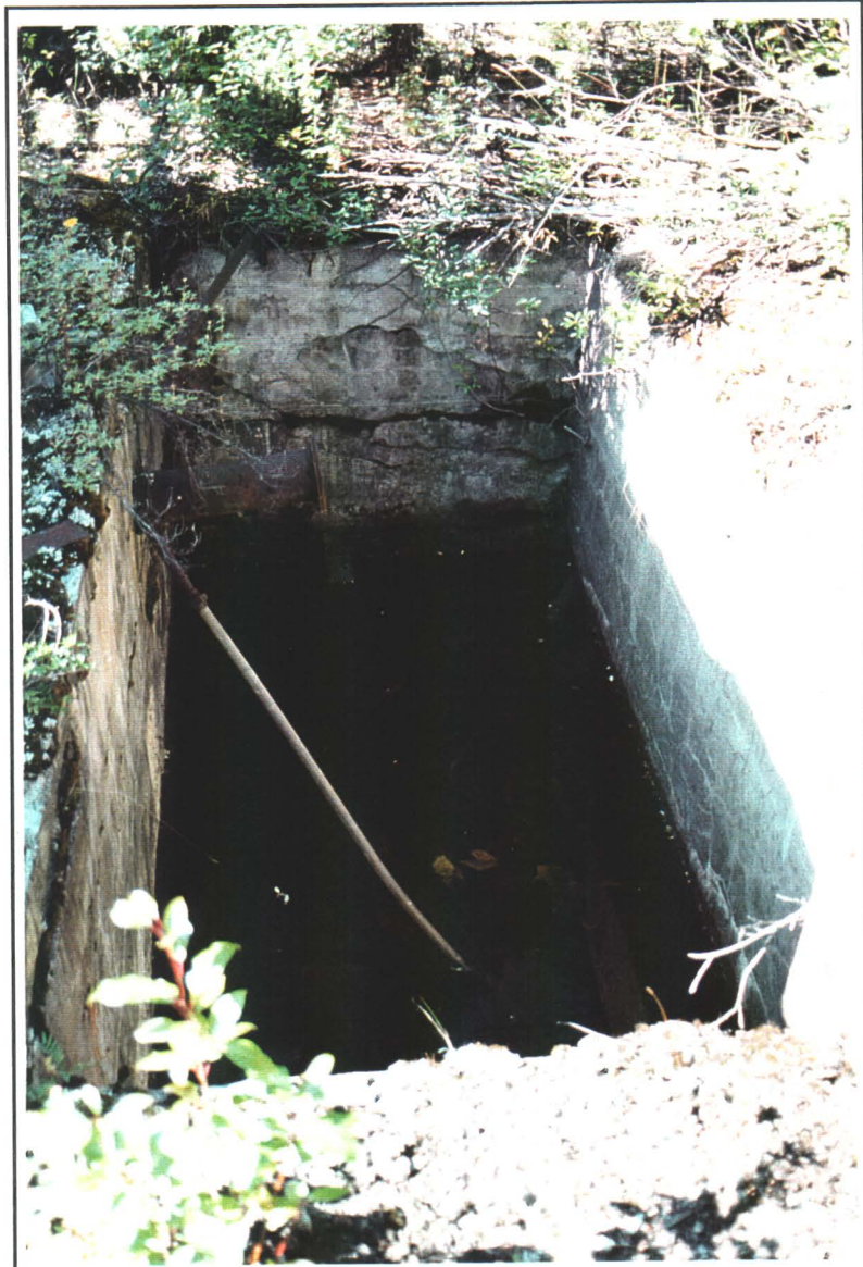
Photo # 19 - Typical Sump Structure near Powerhouse
