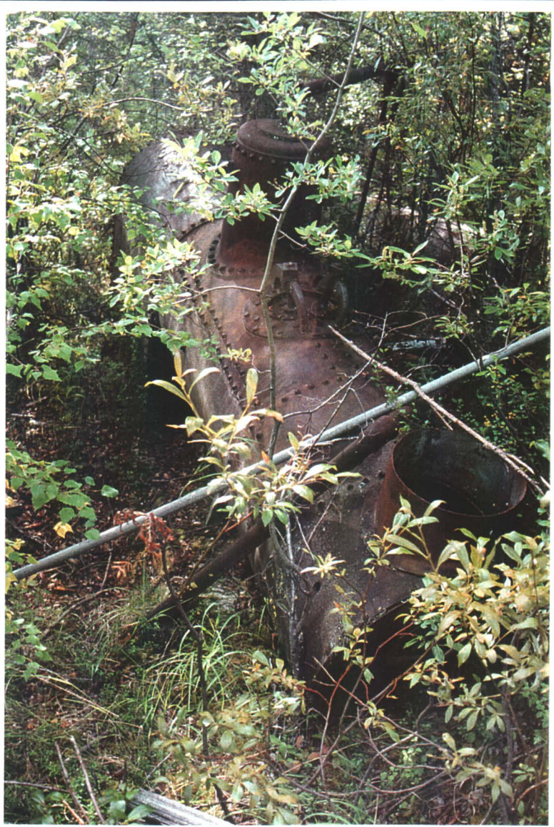
Photo # 9 - Boiler Unit near Maintenance Building
