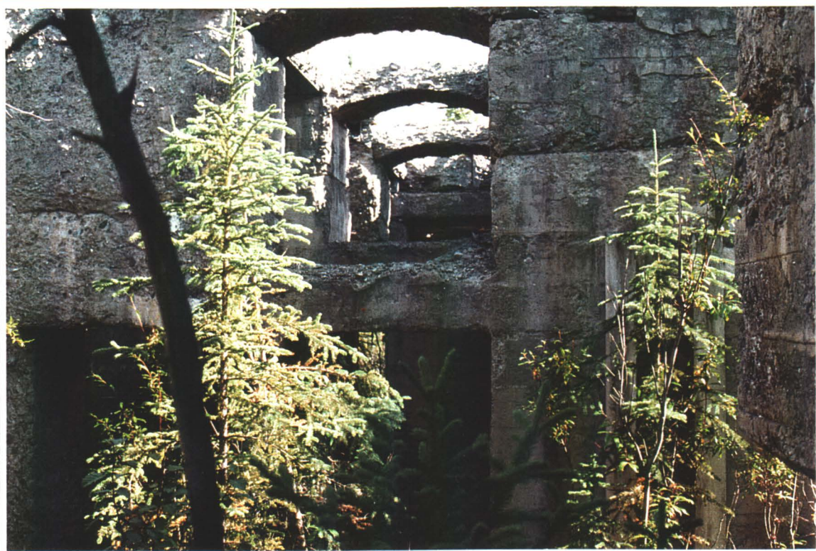
Photo # 16 - Powerhouse Structure
