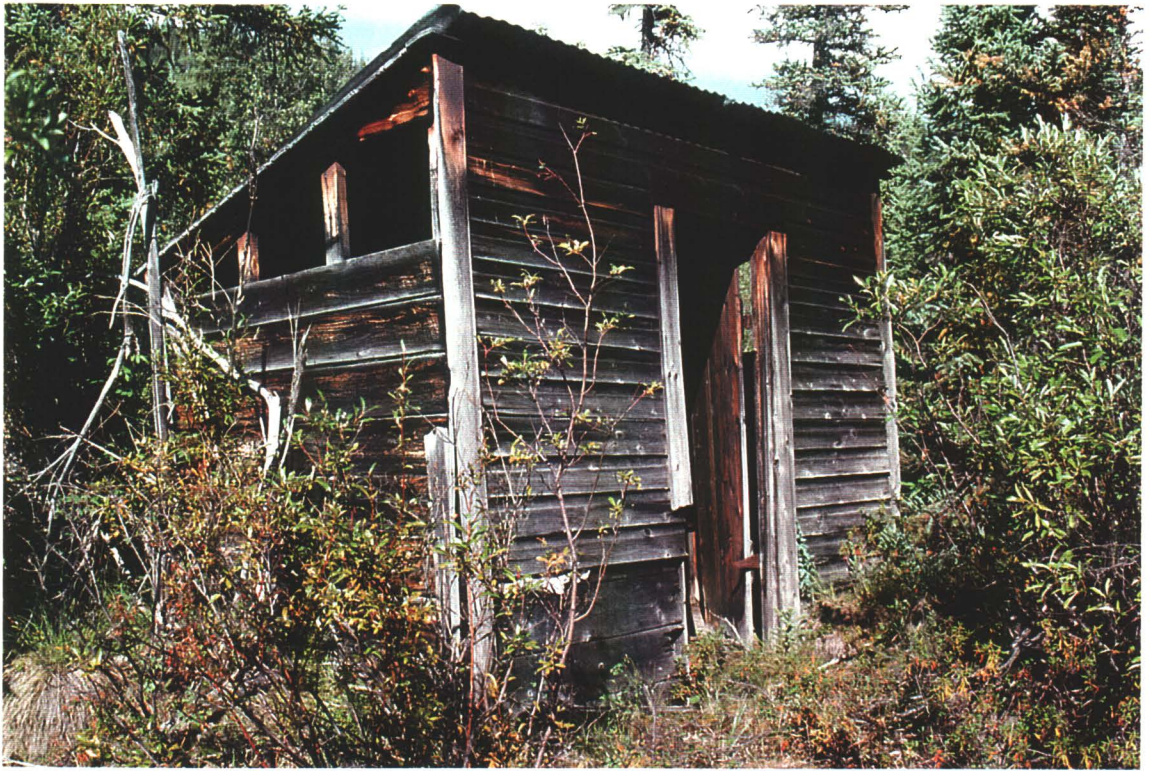
Photo # 21 - Shed across Stream, near Powerhouse
