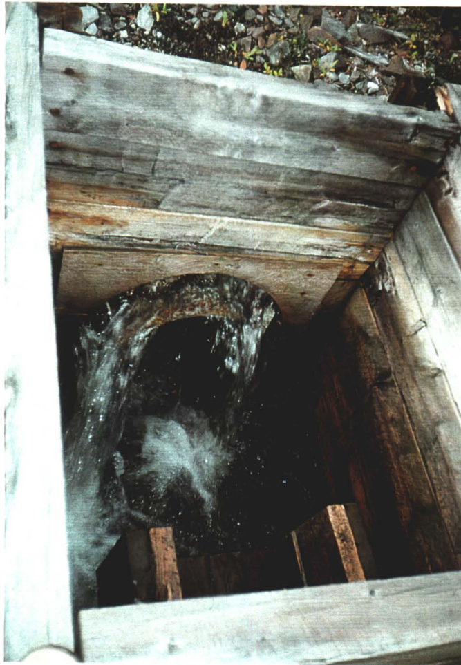
Photo 10. French drain entry adjacent to adit opening.
