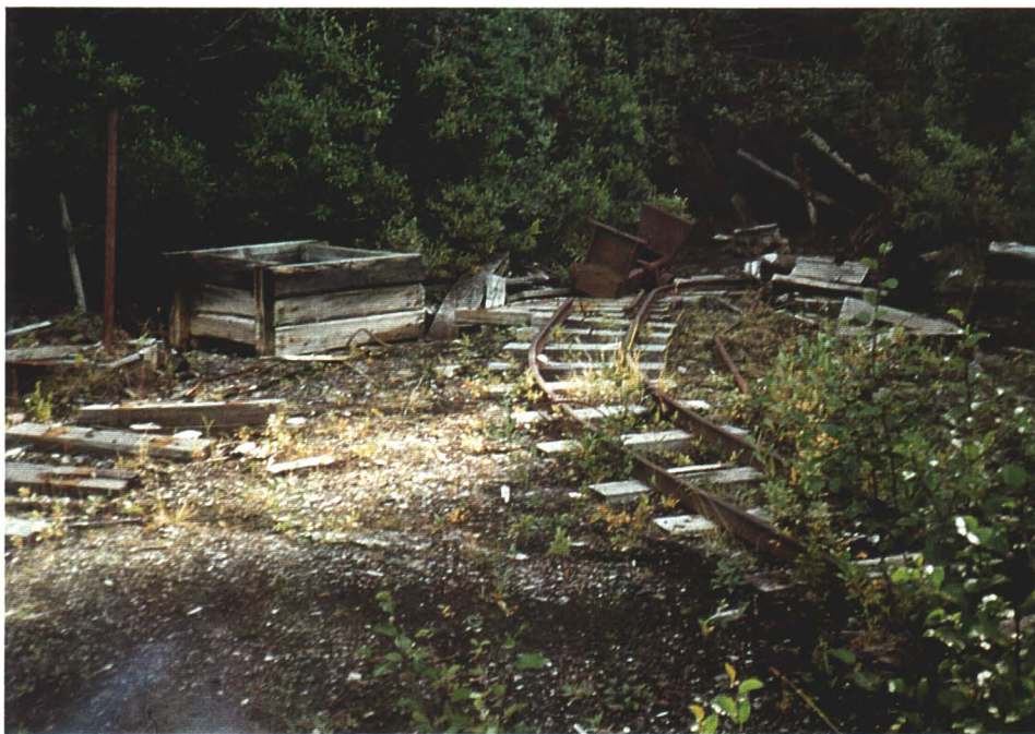
Photo 4. Trestle leading towards covered adit entrance. Note ore cars (rear) & French drain (left).
