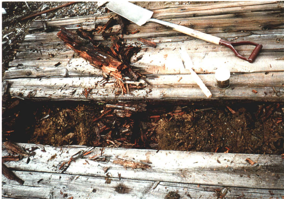
Photo 12. Site of SG-SL-201 taken beneath floorboards of suspected generator shack.
