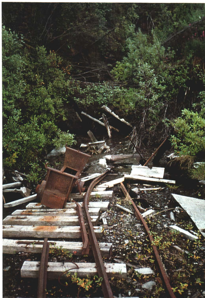
Photo 18. Detail of trestle and covered over entrance to adit.
