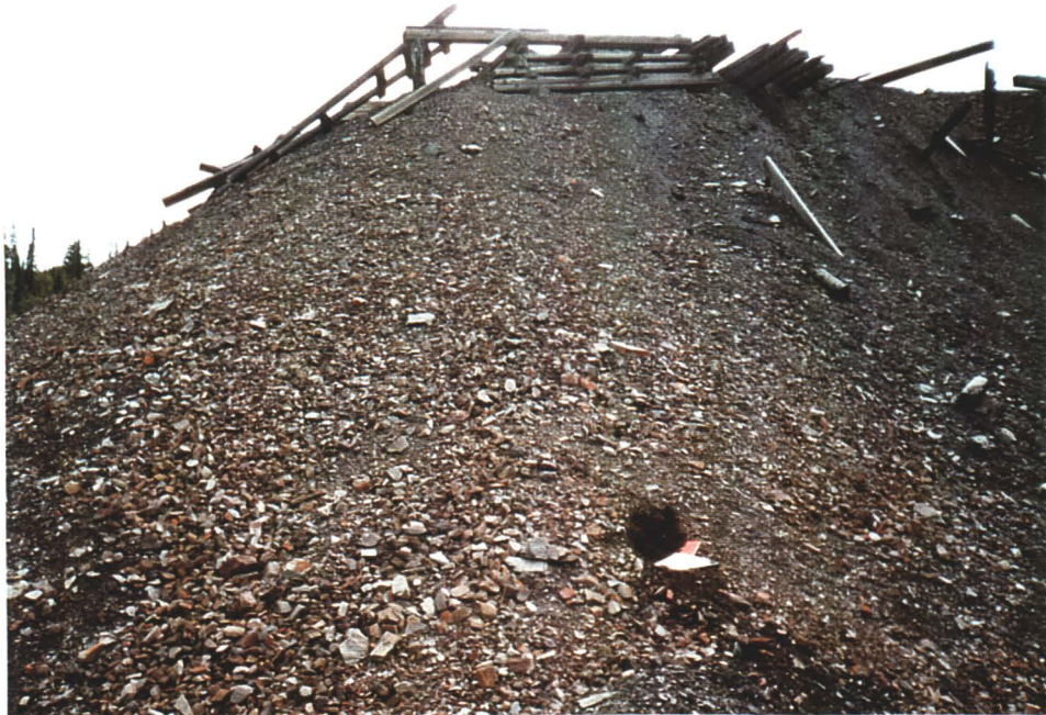
Photo 20. Test pit SG-WR-P305 looking east and located on northwest side of waste rock pile.
