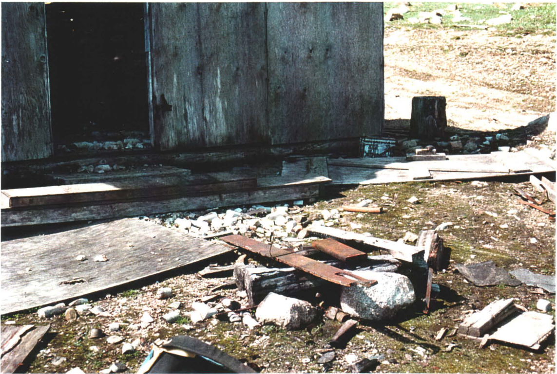
Photo#14: Site Debris by Core Storage and Assay Building
