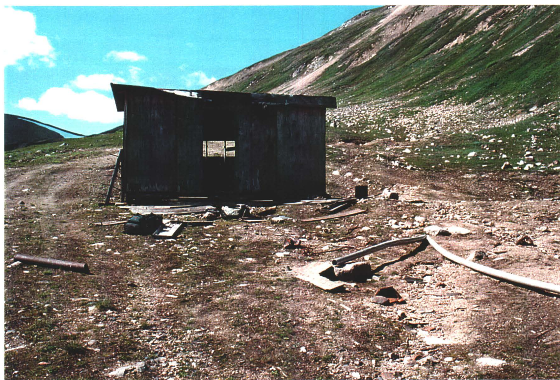
Photo# 12: Core Storage and Assay Building
