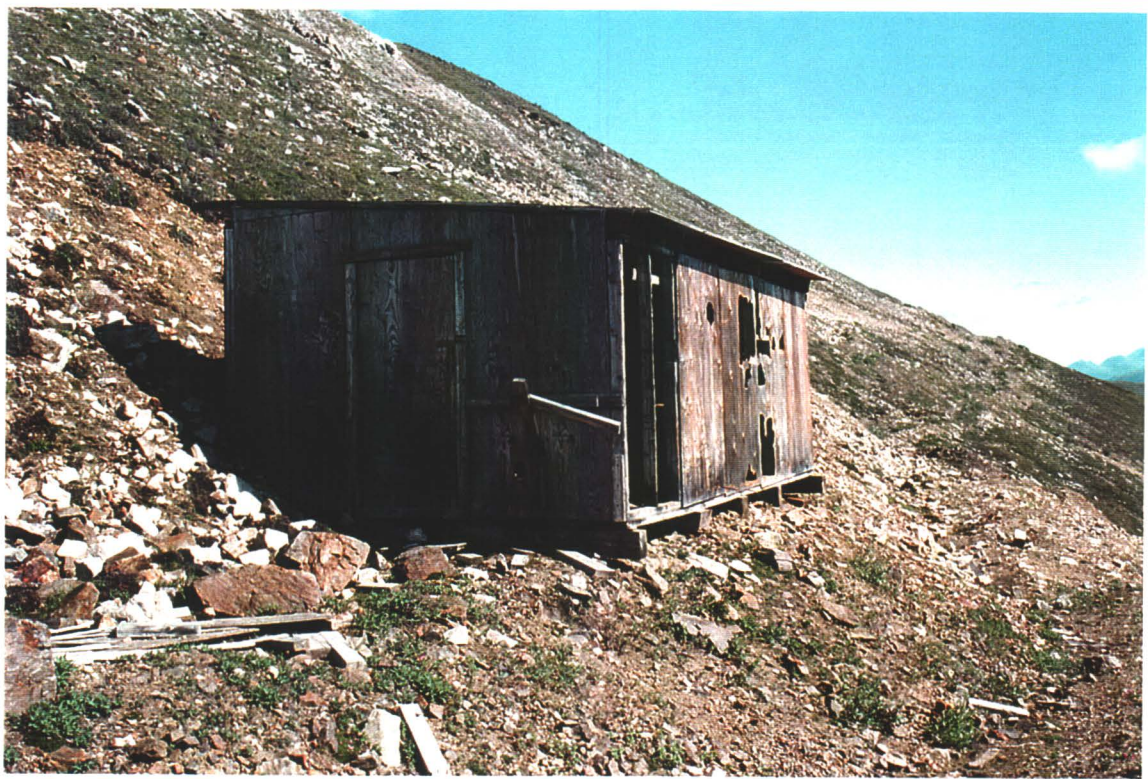
Photo# 8: Building at Upper Site
