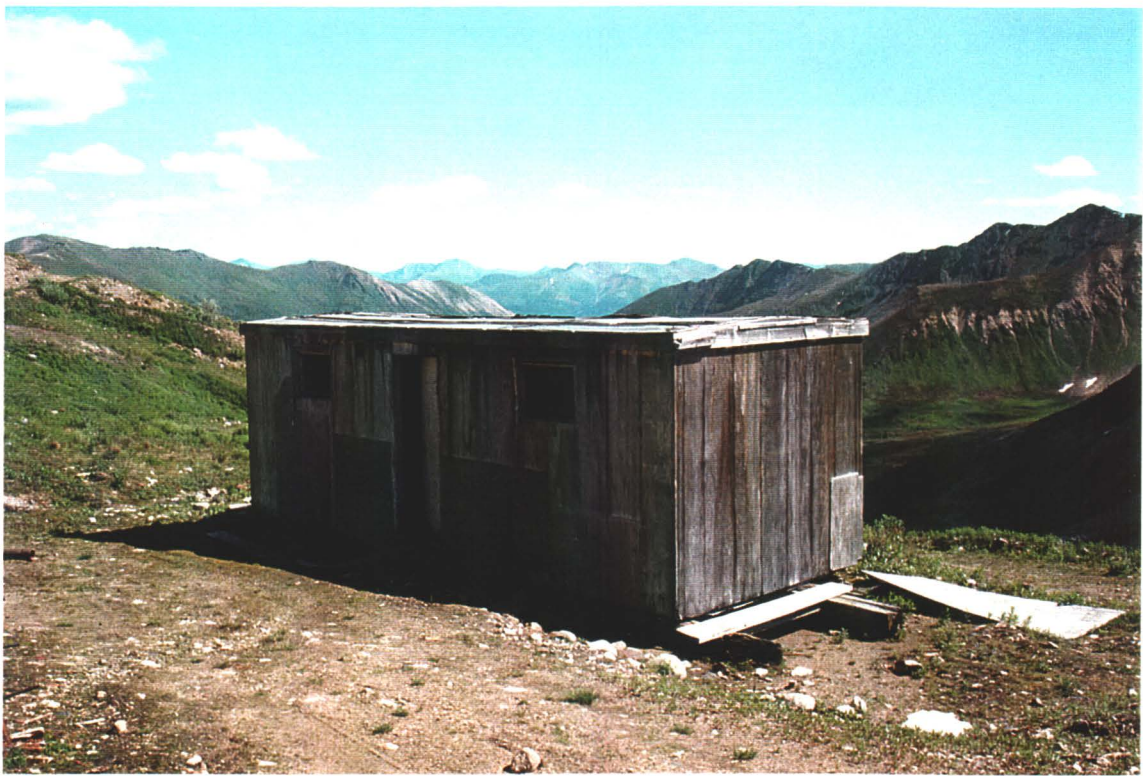
Photo# 10: Kitchen and Mess Building
