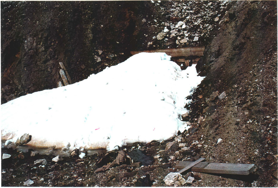
Photo# 5: Adit at Upper Site
