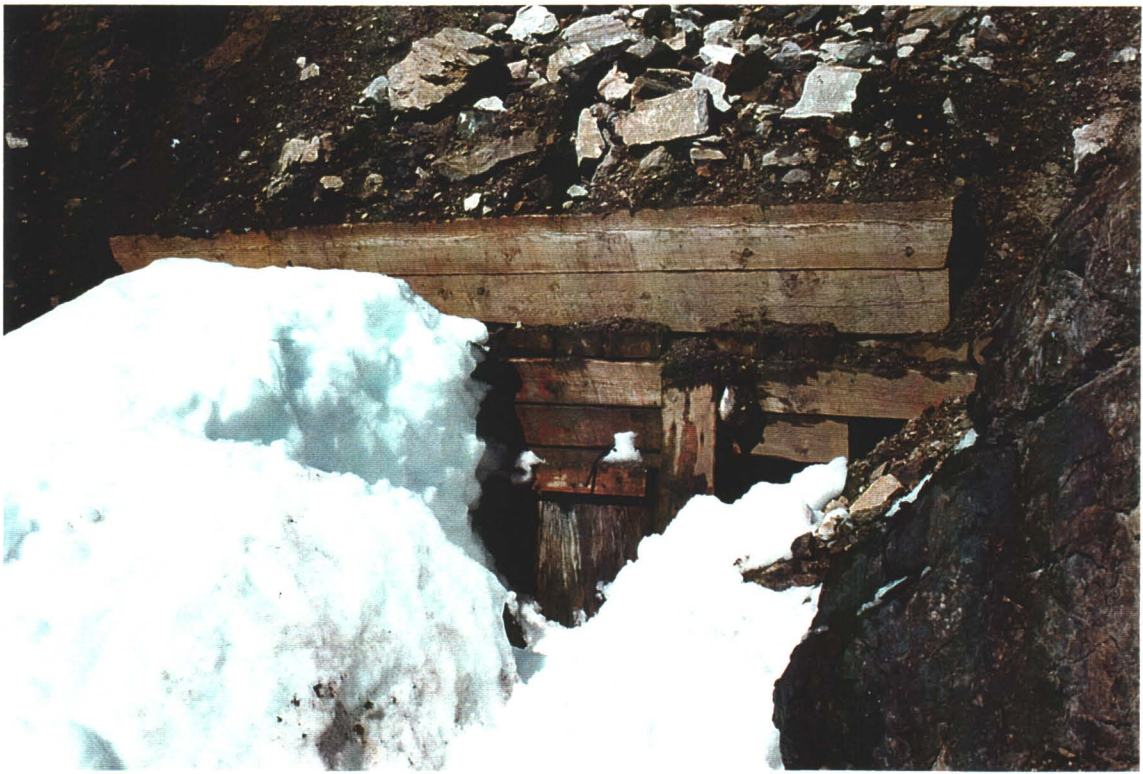
Photo# 6: Adit Seal
