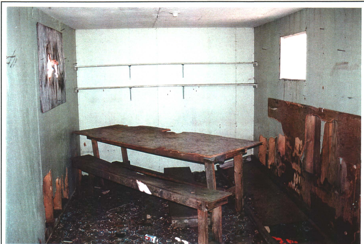
Photo# 11: Kitchen and Mess Interior
