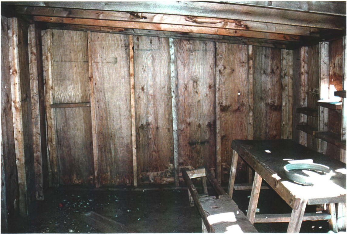
Photo# 9: Interior of Building at Upper Site
