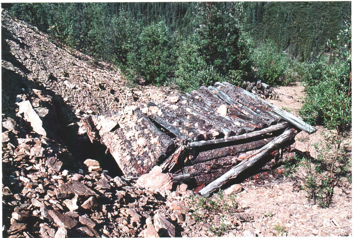
Photo # 14 - Upper Adit
