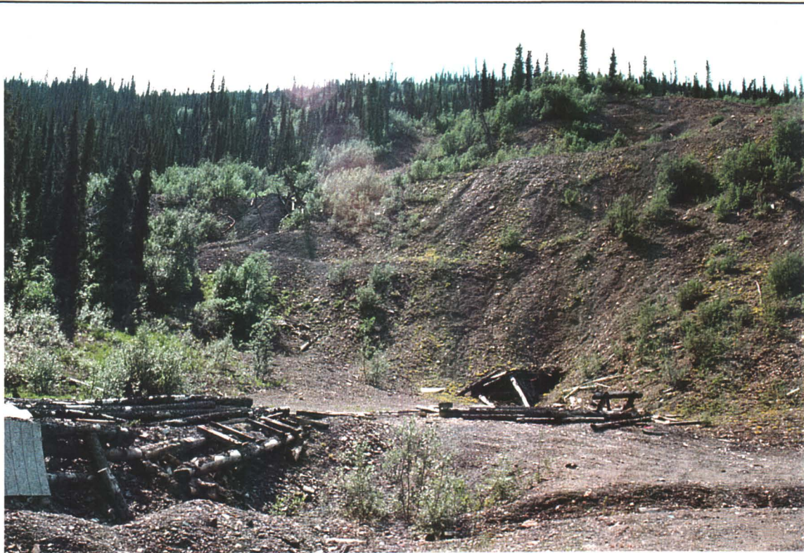
Photo # 4 - Load-out Ramp and Lower Adit
