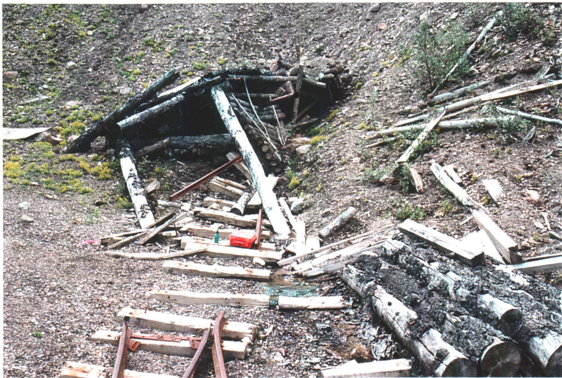
Photo # 7 - Seepage from Lower Adit
