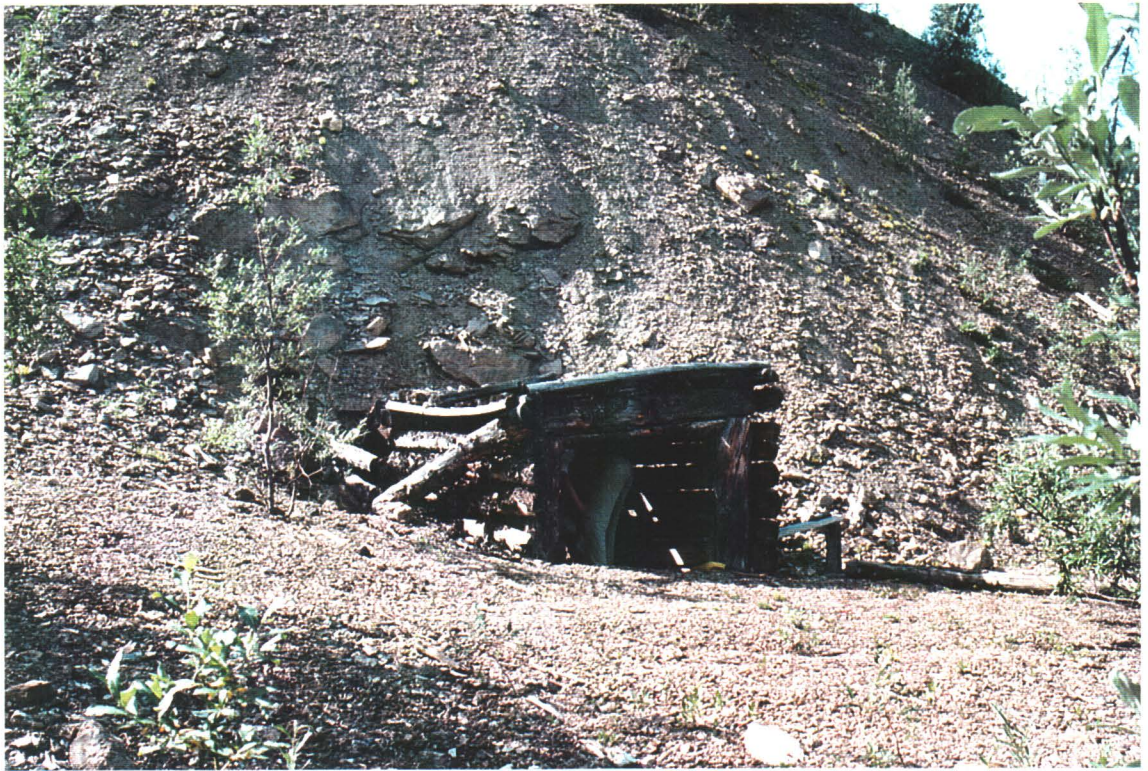
Photo # 13 - Upper Adit
