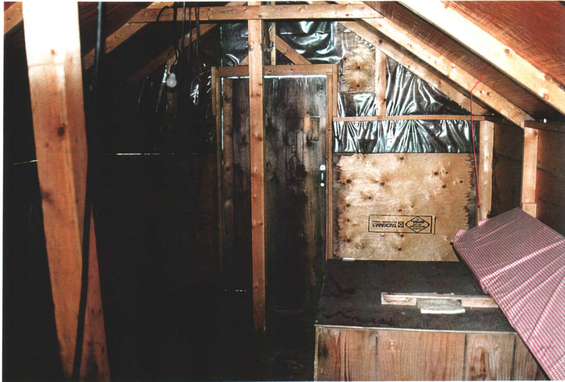
Photo# 11: Mess Hall Interior
