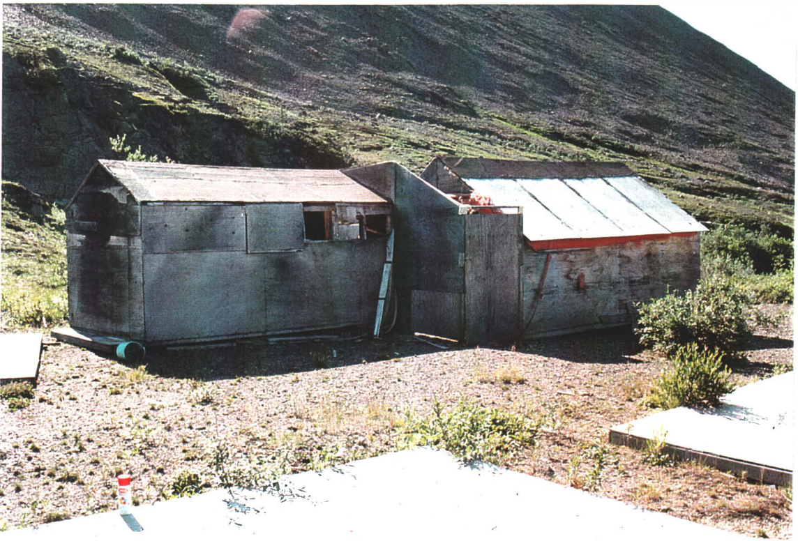
Photo# 10: Kitchen and Mess Buildings
