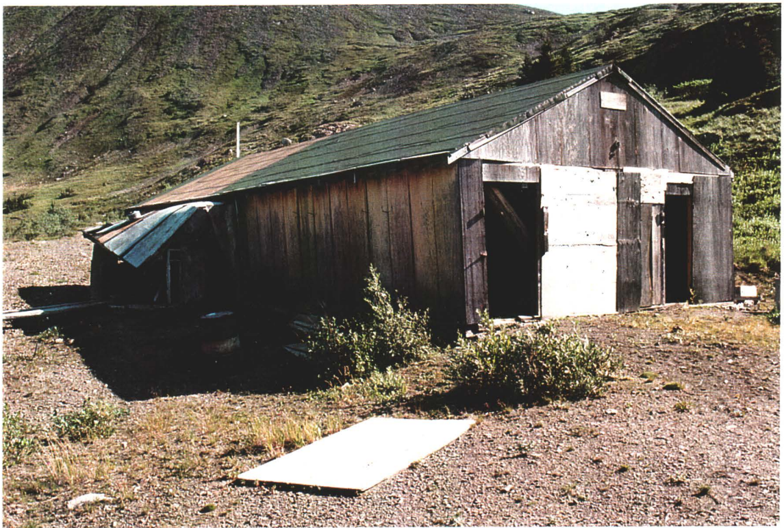
Photo# 8: Maintenance Shop
