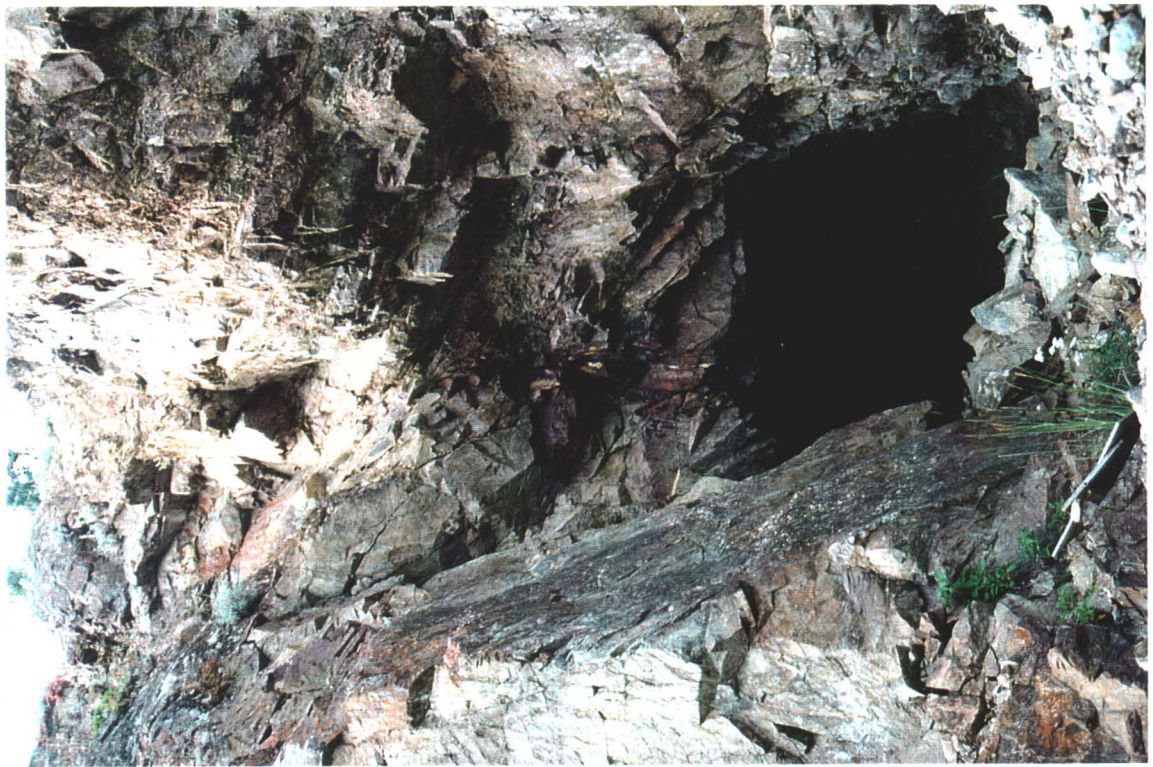
Photo # 2 - Adit, Right Site (East) - Lower Adits
