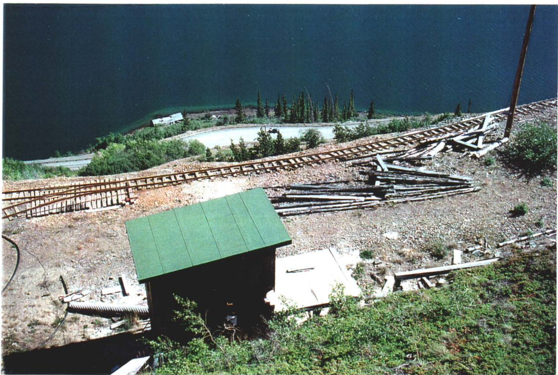
Photo # 27 - View from Ventilation Building - Track and Wood Debris
