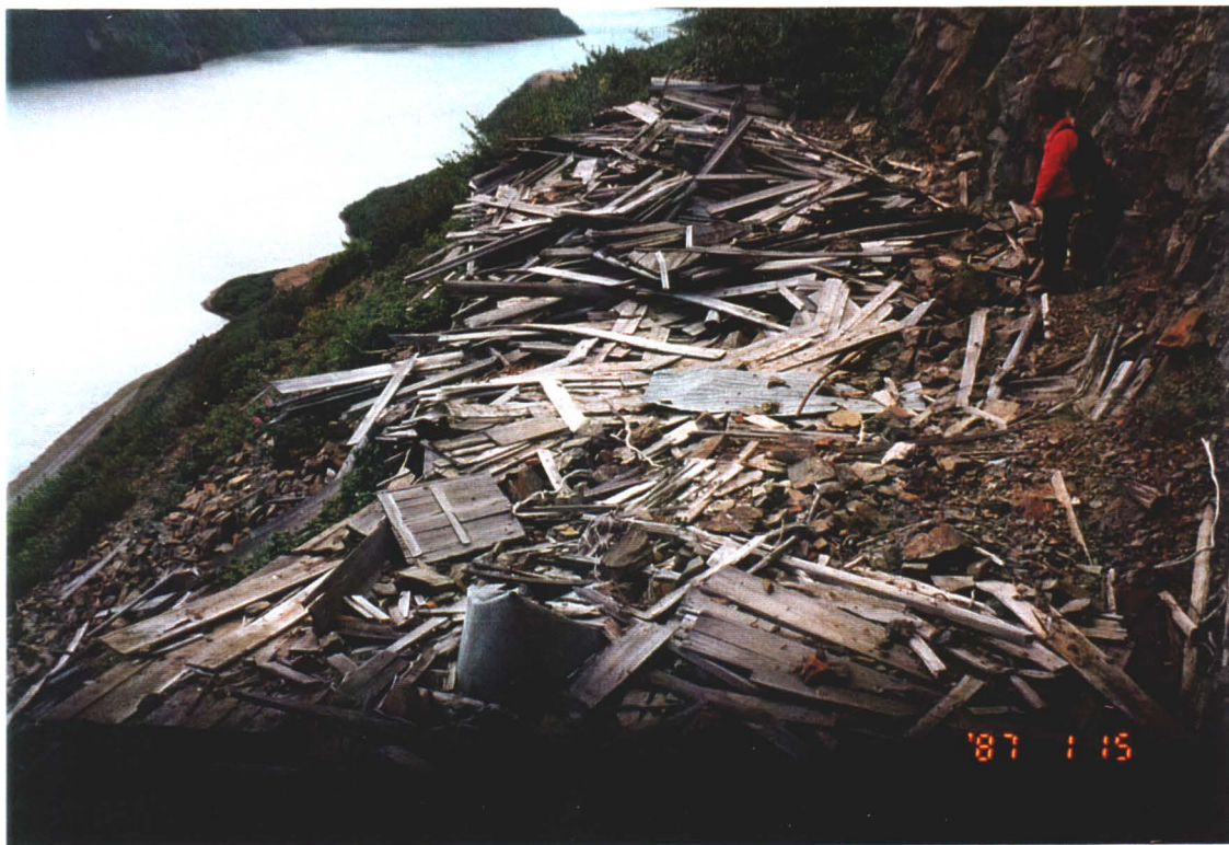
Photo # 33 - Wood Debris at Headframe
