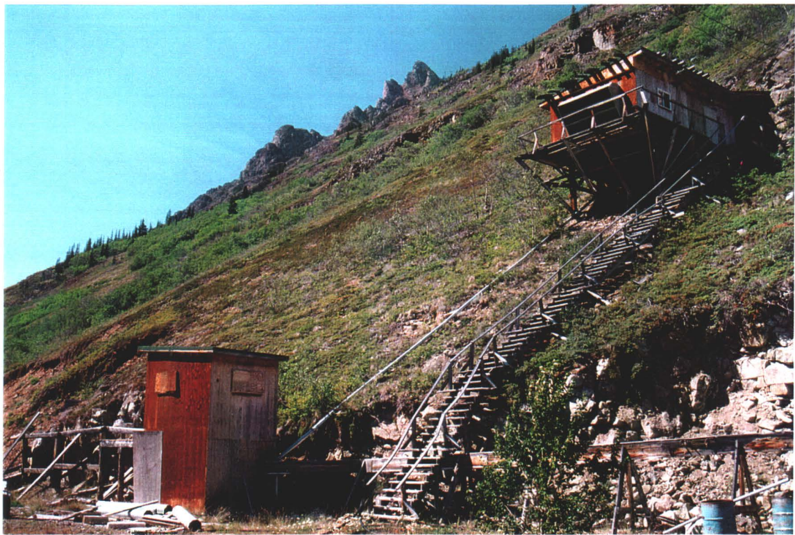
Photo # 17 - Mixing Tank and Ventilation Building
