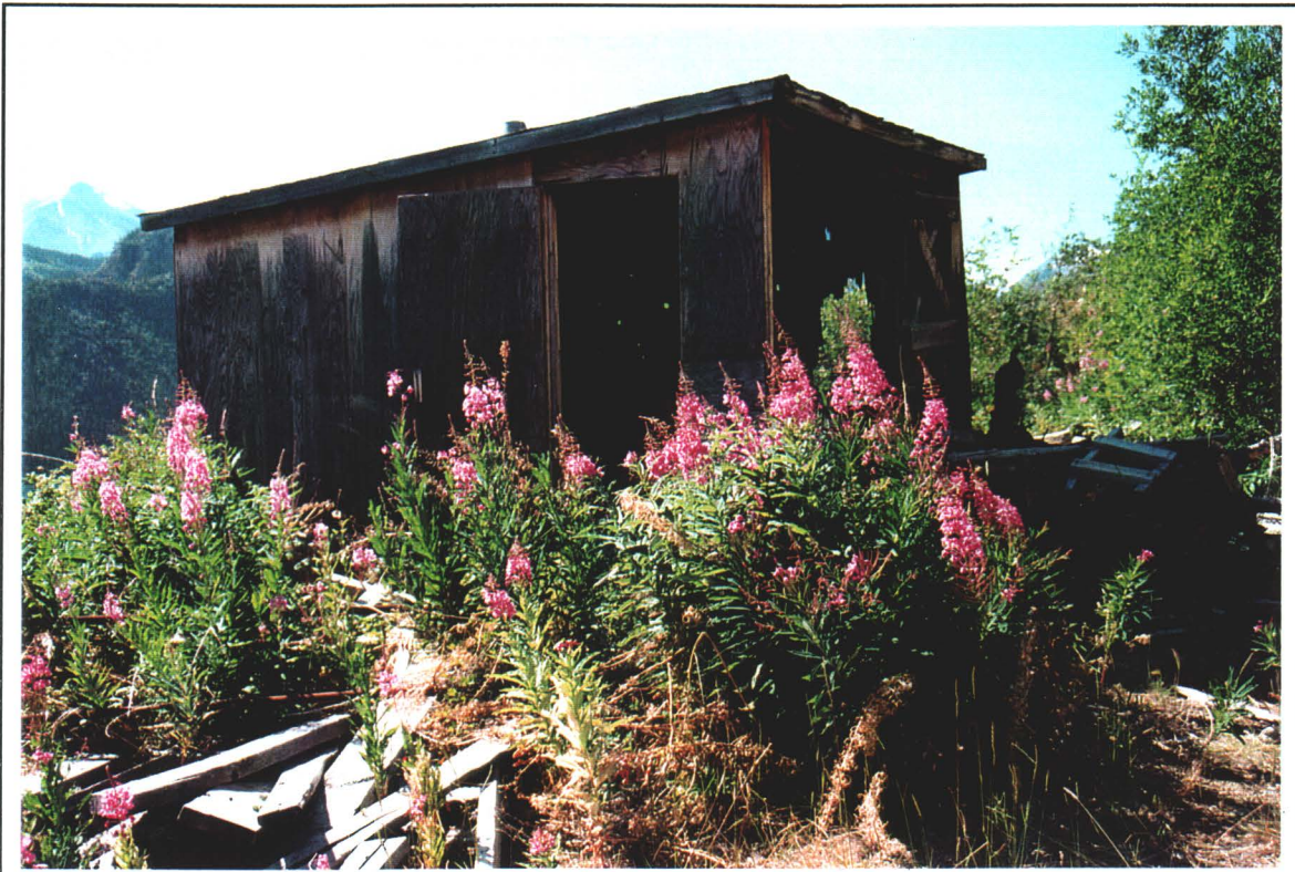
Photo # 1 - Storage Shack, South End - Adit 1
