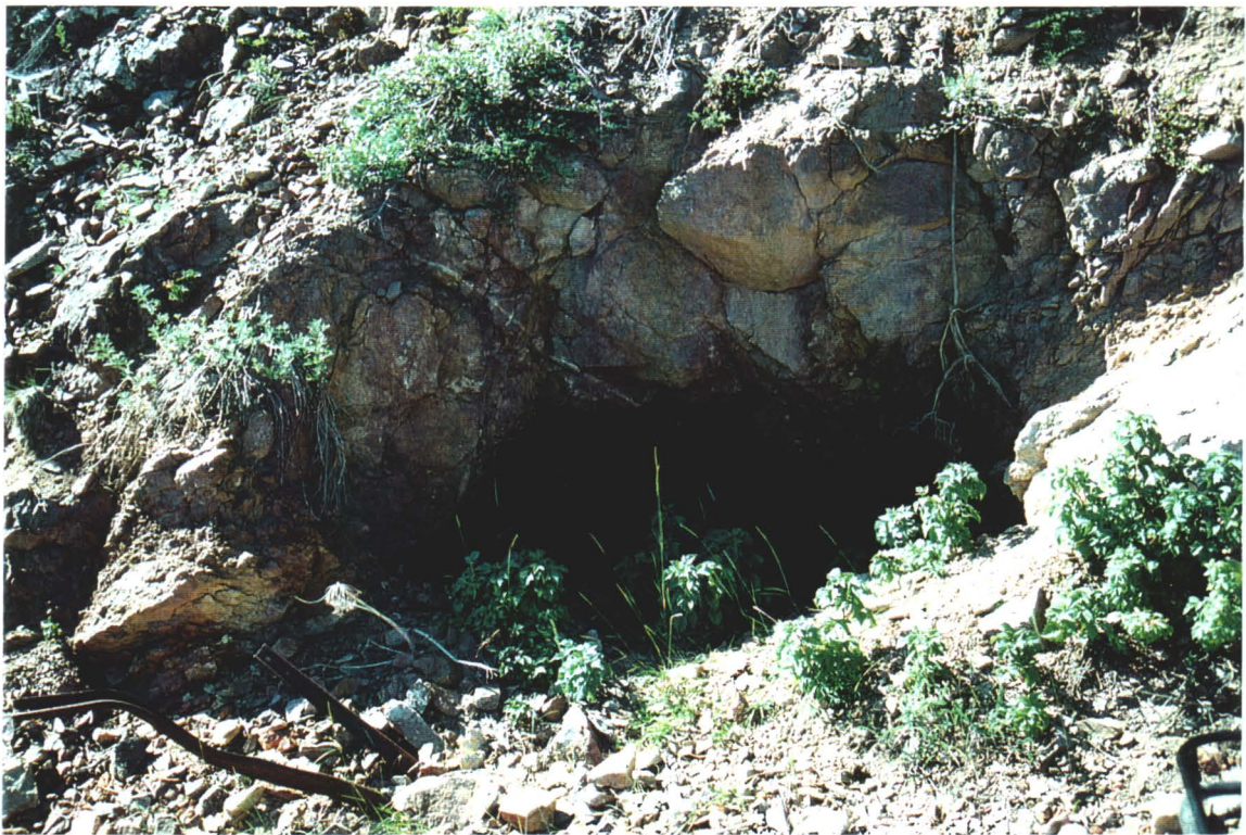
Photo # 31 - Collapsed Adit
