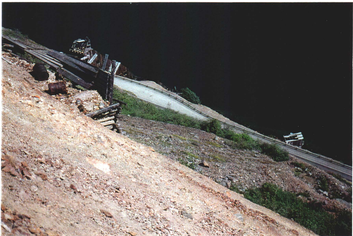
Photo # 29 - Lower Retaining Wall - Loadout Facility at Lake Bennett below
