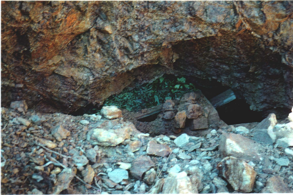
Photo # 30 - Collapsed Adit
