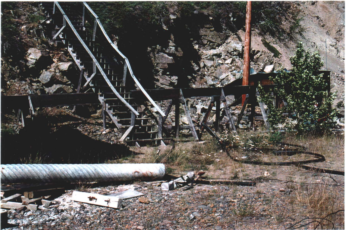
Photo # 19 - Part of Stairway and Trestle
