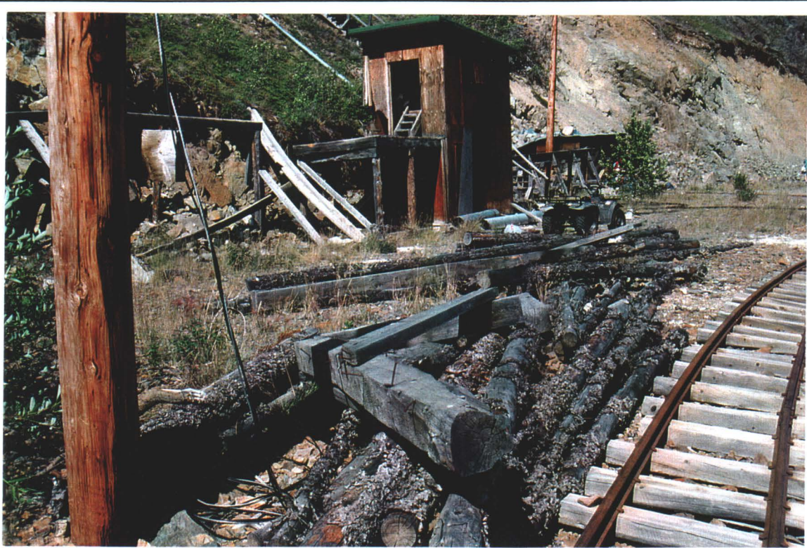
Photo # 18 - Wood Debris by Mixing Tank
