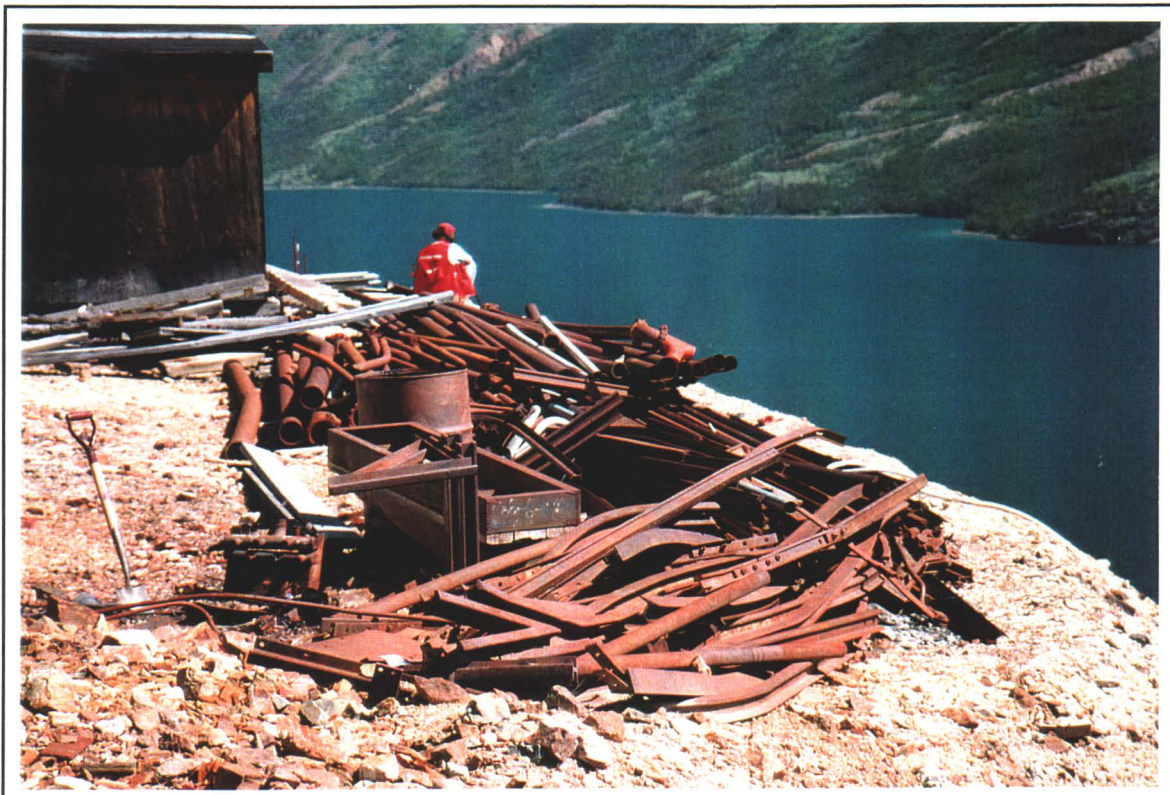
Photo # 14 - Overall View Miscellaneous Metals
