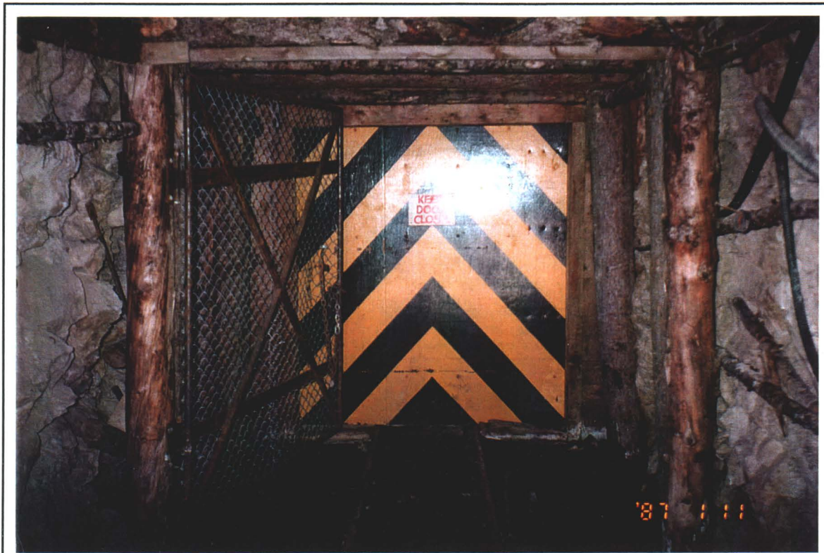
Photo # 37 - Detail of Adit 1
