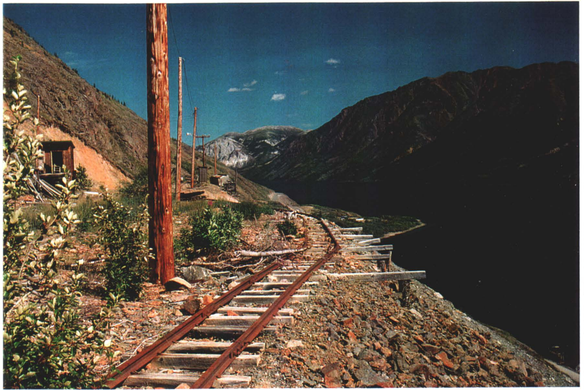
Photo # 16 - Extent of Track and Pole Lines
