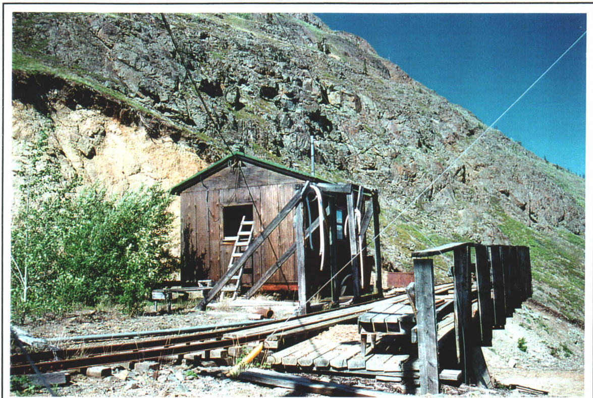
Photo # 24 - Storage Shed and Offloading Platform
