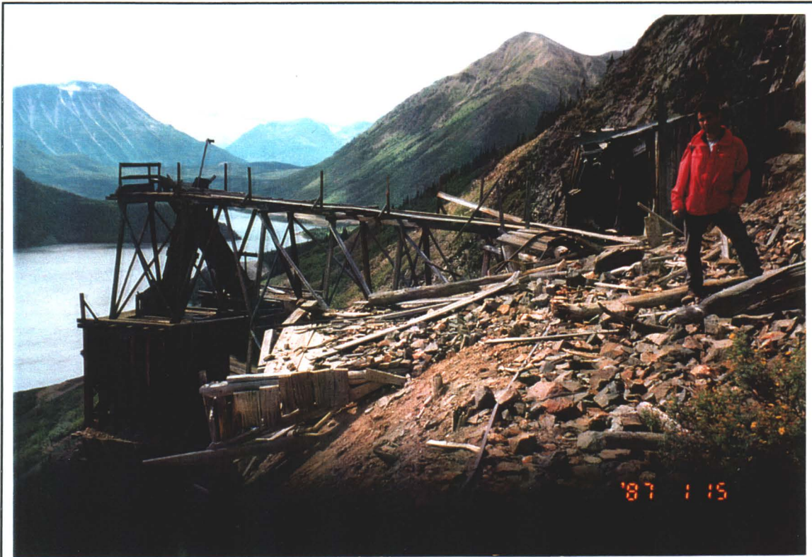
Photo # 34 - Loadout Facility at Headframe; and Trestle
