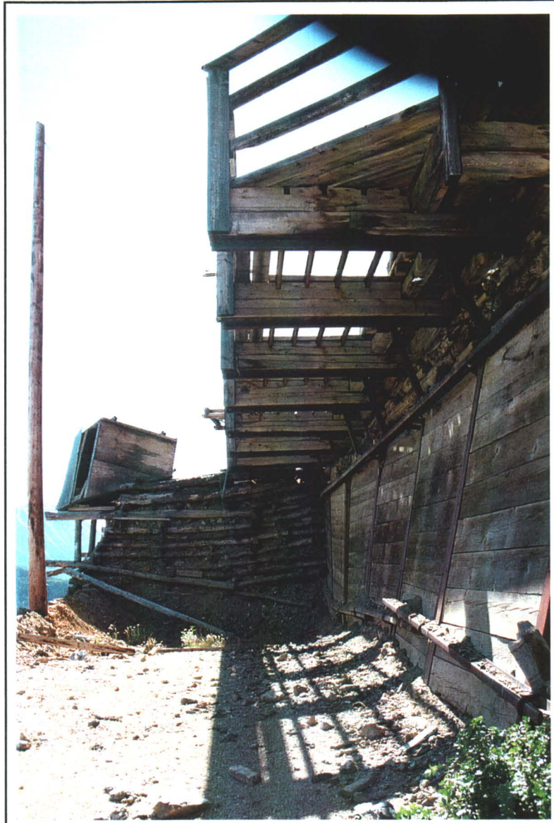
Photo # 25 - Retaining Walls at Offloading Platform
