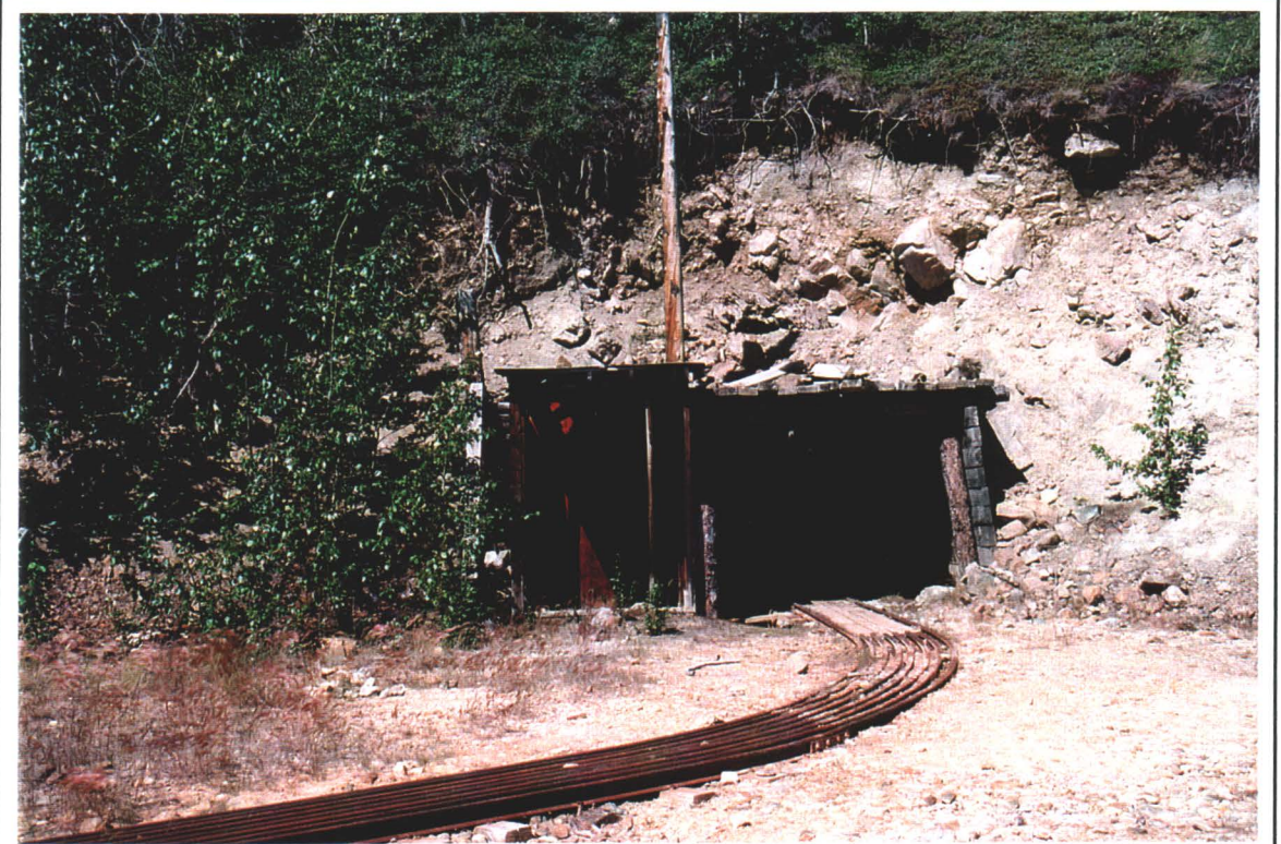
Photo # 7 - Adit No. 1
