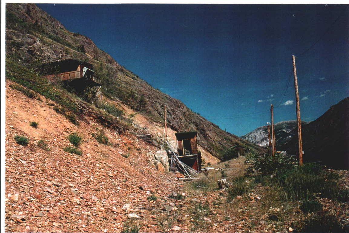
Photo # 15 - Overall View of Lower Adit Site
