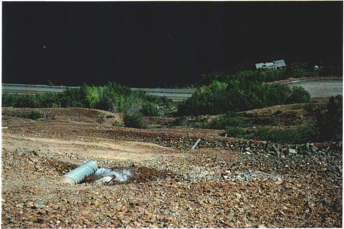
Photo # 28 - Pipe discharging Water
