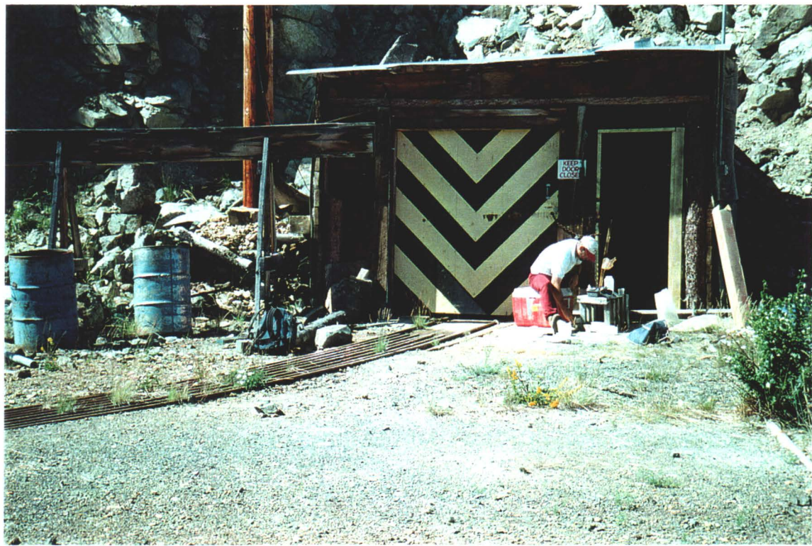
Photo # 21 - Adit No. 2
