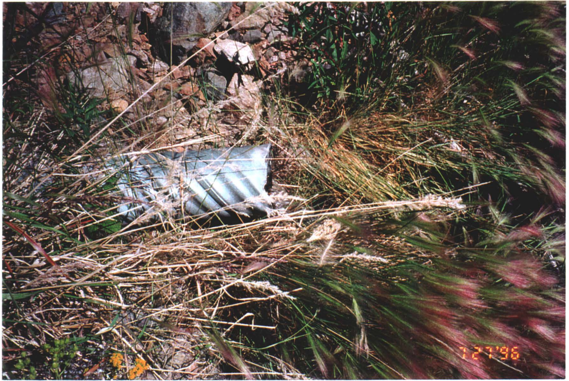
Photo # 44 - Culvert carrying Seep Water below Adit 2
