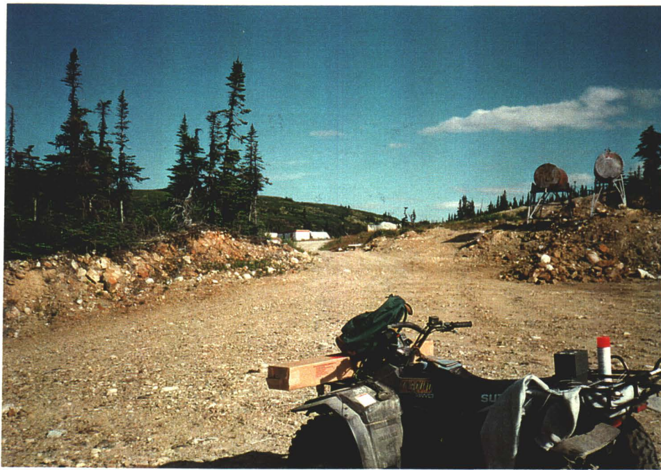
Photo 8. Service road to upper tent camp area with twin ASTs in trailer camp area (right) and tent camp area (background).
