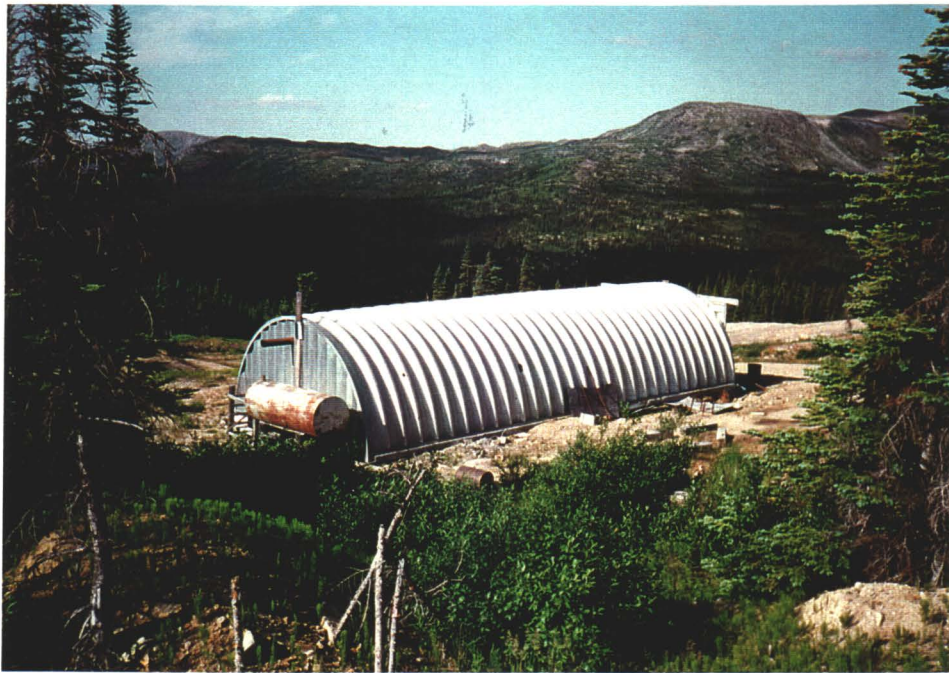
Photo 2. Prefabricated metal maintenance shed with AST and adit area (background).
