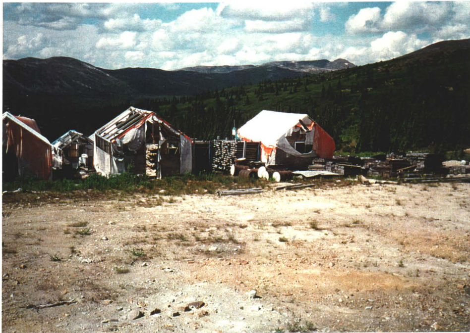
Photo 9. Sleeping tent frames with wood waste at right and metal barrels strewn about site.
