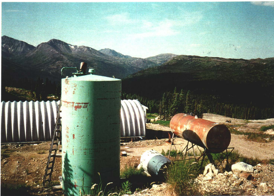
Photo 4. View of maintenance area ASTs with main adit and waste rock area below.
