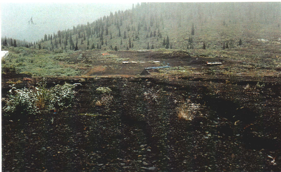
Photograph 5-1: Airstrip looking downslope to the west showing poor condition of grade. The open storage area can be seen further to the west
