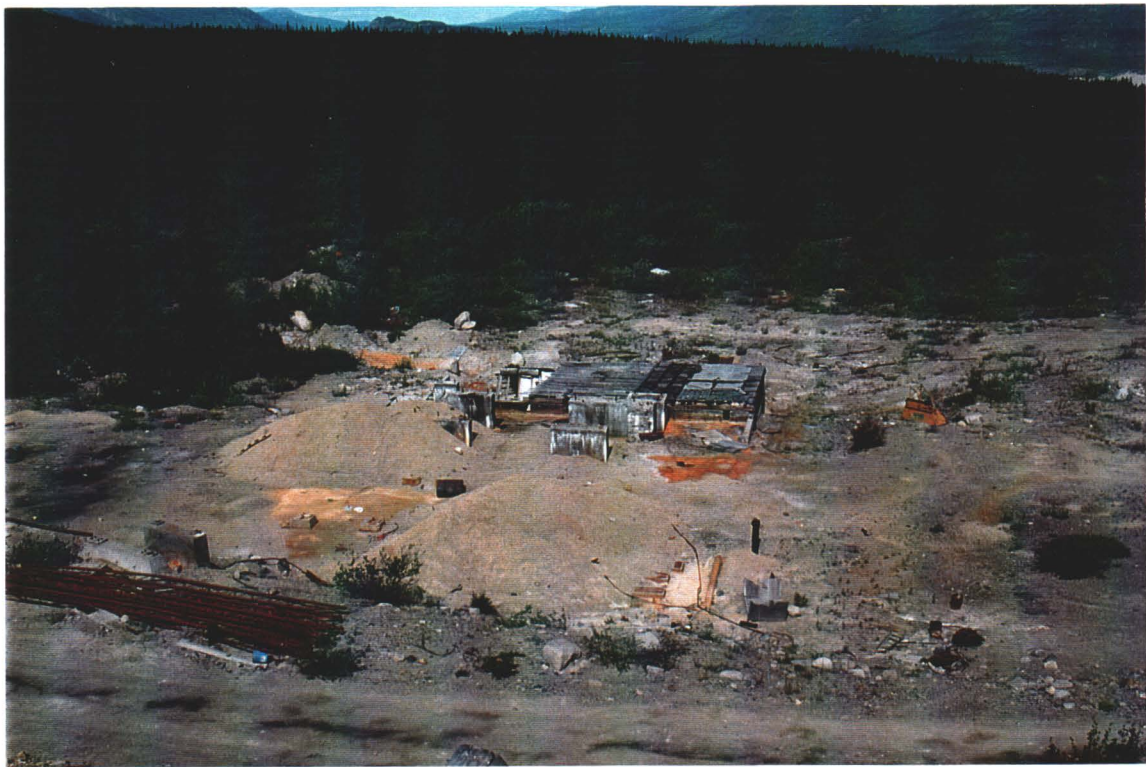
Photo# 11: Mill Site Foundation and Ore Piles
