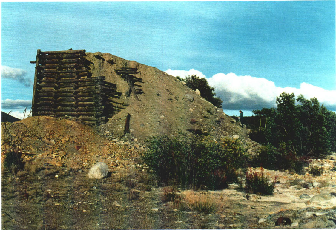
Photo# 10: Log Cribbing at West End of Loadout Ramp
