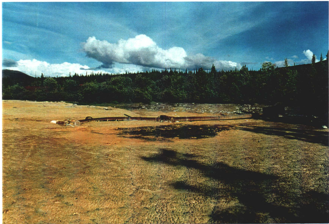
Photo# 4: Decant Pipe (note low lying wet area)
