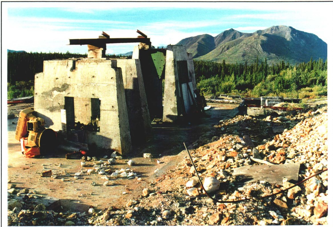
Photo# 12: Concrete Pillars on Foundation
