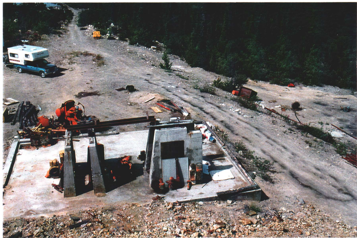
Photo# 13: Mill Foundation and Debris
