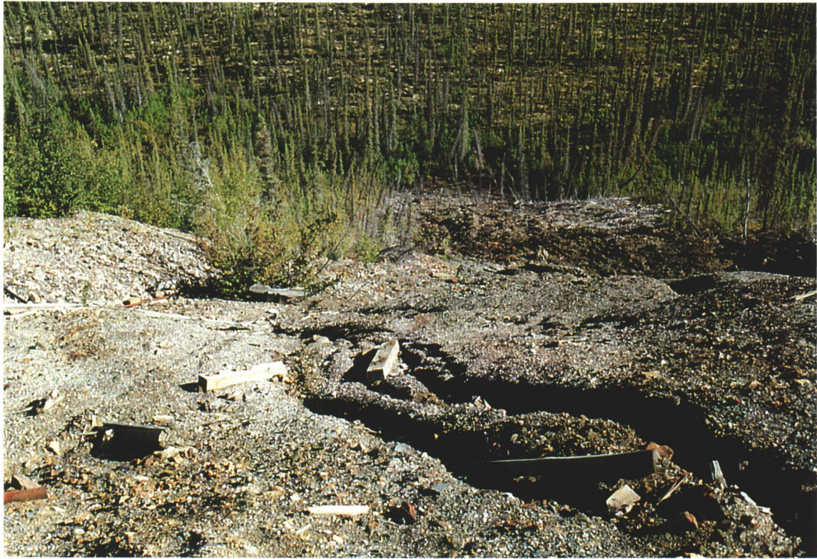
Photo 2. Tension cracks at crest of lower/eastern waste rock slope.
