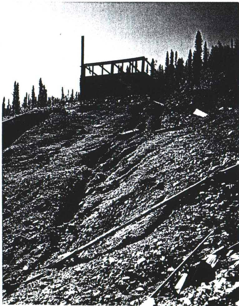
Photo #F1: Looking up the lower waste rock pile slope at the old garage. Note rivuleting due to surface runoff.
