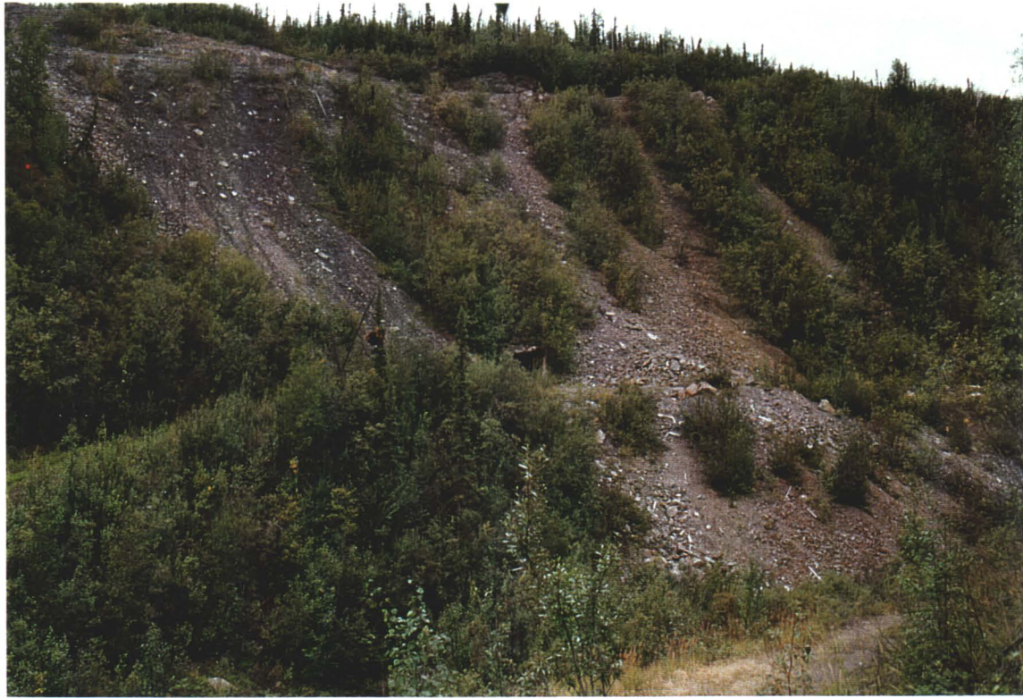
Photo 3. Paddy waste rock slope. Upper Road is visible at top left of photo; adit is visible at center of photo.
