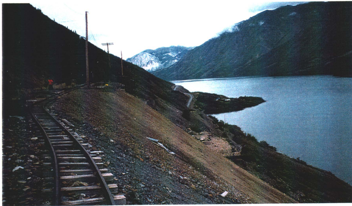
Photo #V2: Looking north along tracks at area of adit 2. Note culvert along waste rock pile slope; note lower retaining wall built of log cribbing.
