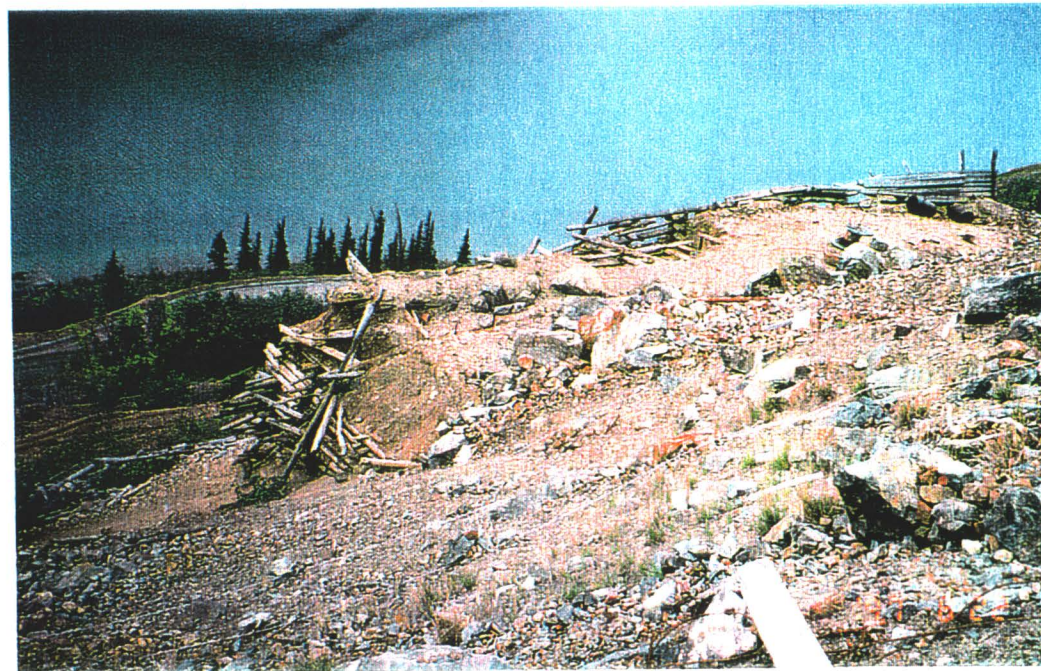
Photo #V4: Looking south east at lower retaining wall. Note sloughing of waste rock material; note poor condition of log cribbing supports.
