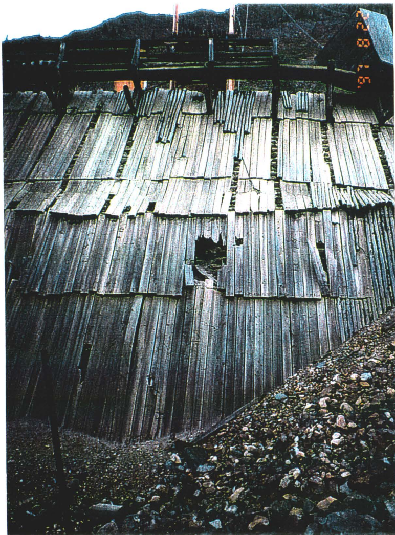
Photo #V3: Looking west at log cribbing retaining structure. Note log cribbing construction; note shack fallen over at top right;
