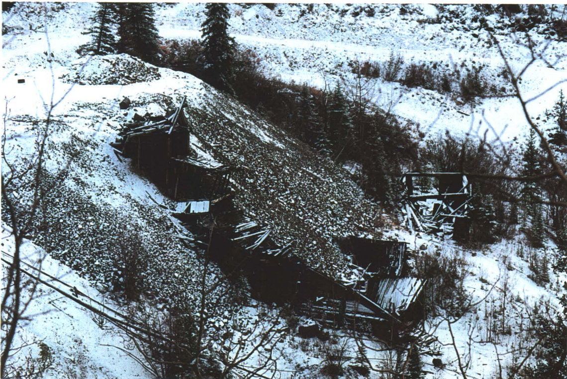
#15 - The same mill in 1999, filled in with waste rock from Level two underground development.
