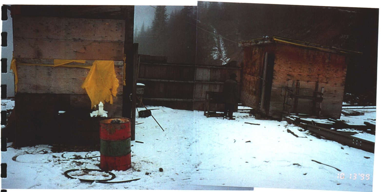
#6 - Buildings at Level Two Adit.
