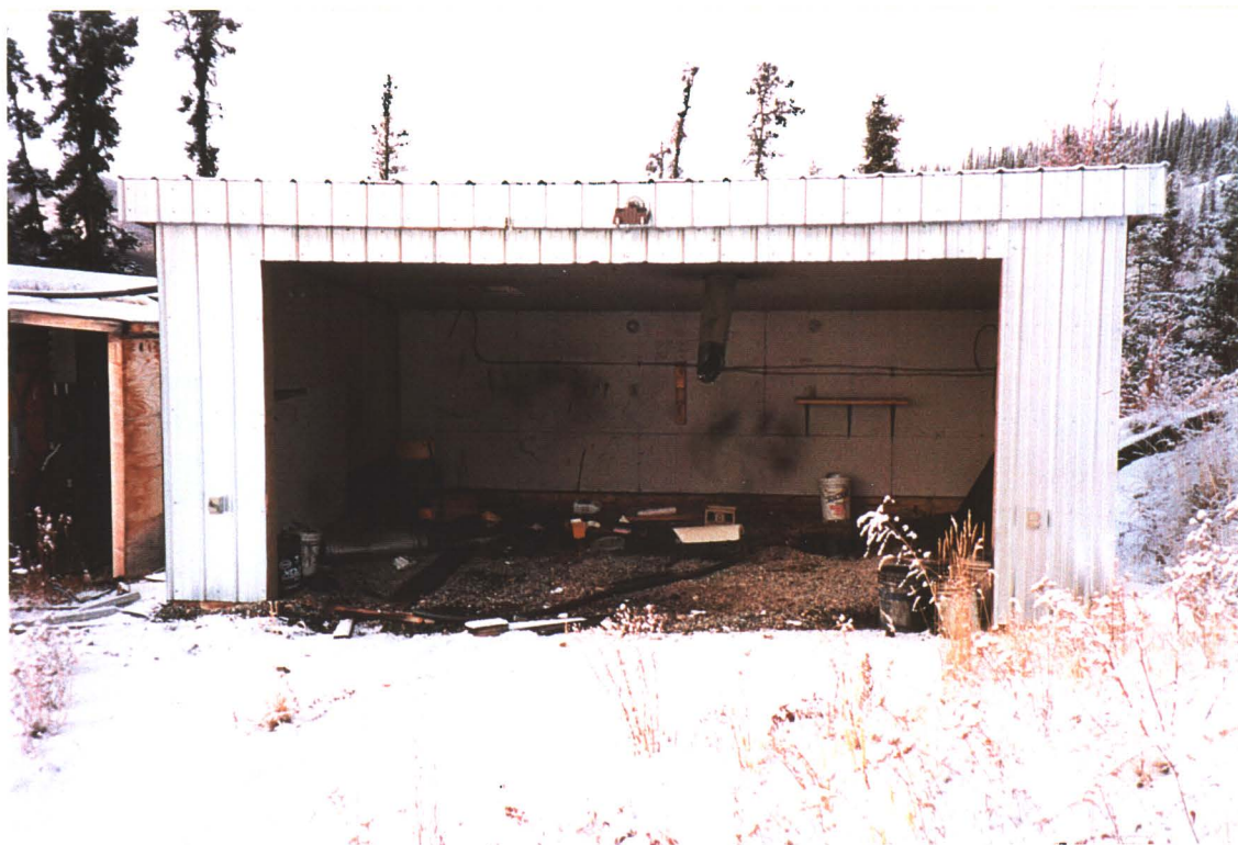
#5 - Generator building at camp. October 14, 1999
