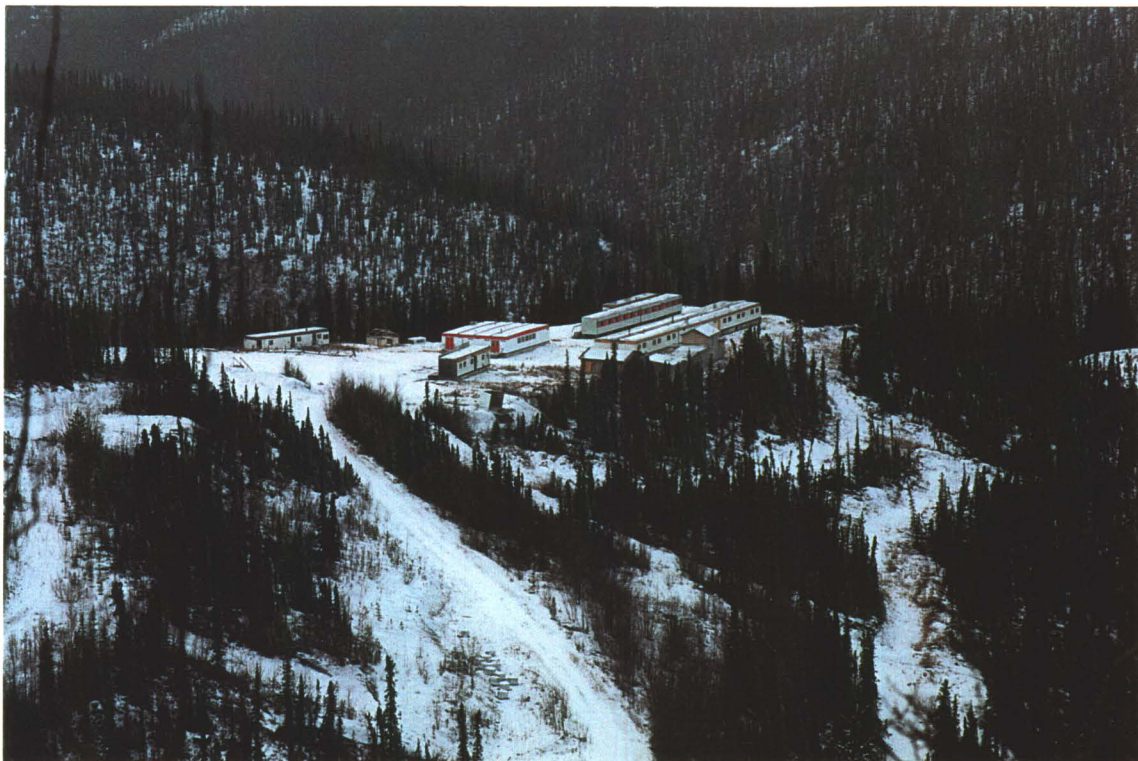
#4 - Camp viewed from Level Two Adit area, looking south.
