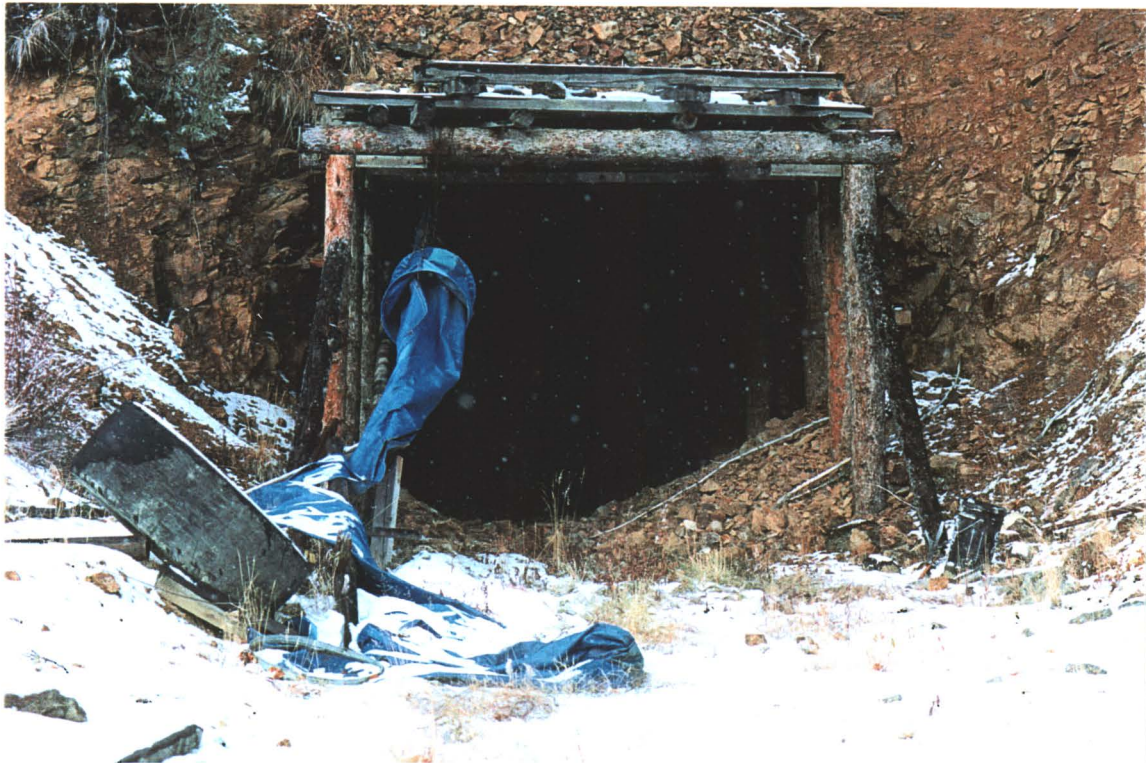
#7 - Level Two Adit opening.
