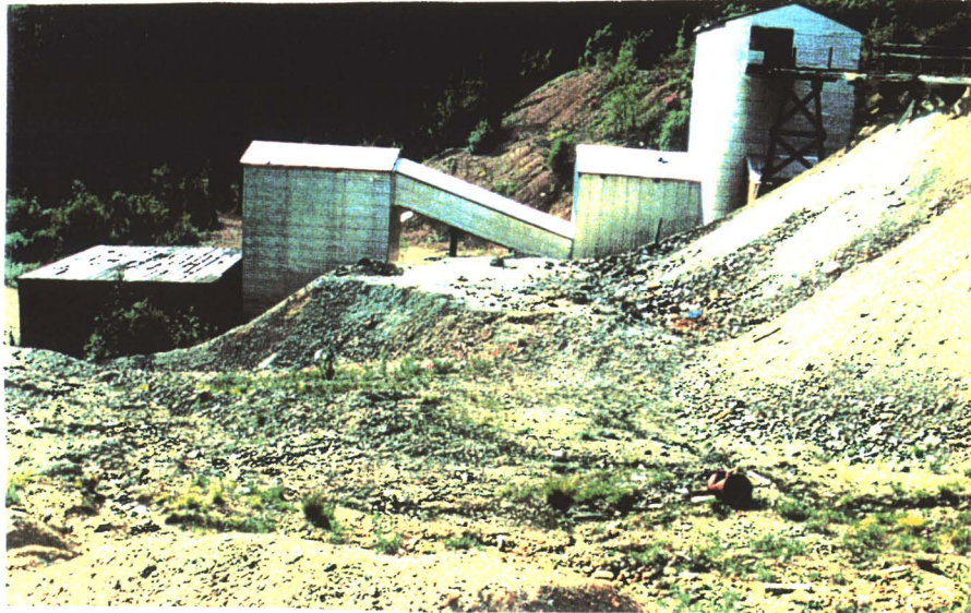
# 8 - Mill built in 1964/5 at Level Four. This structure was demolished to make way for the existing mill buildings, below. (Photo taken 1993)
