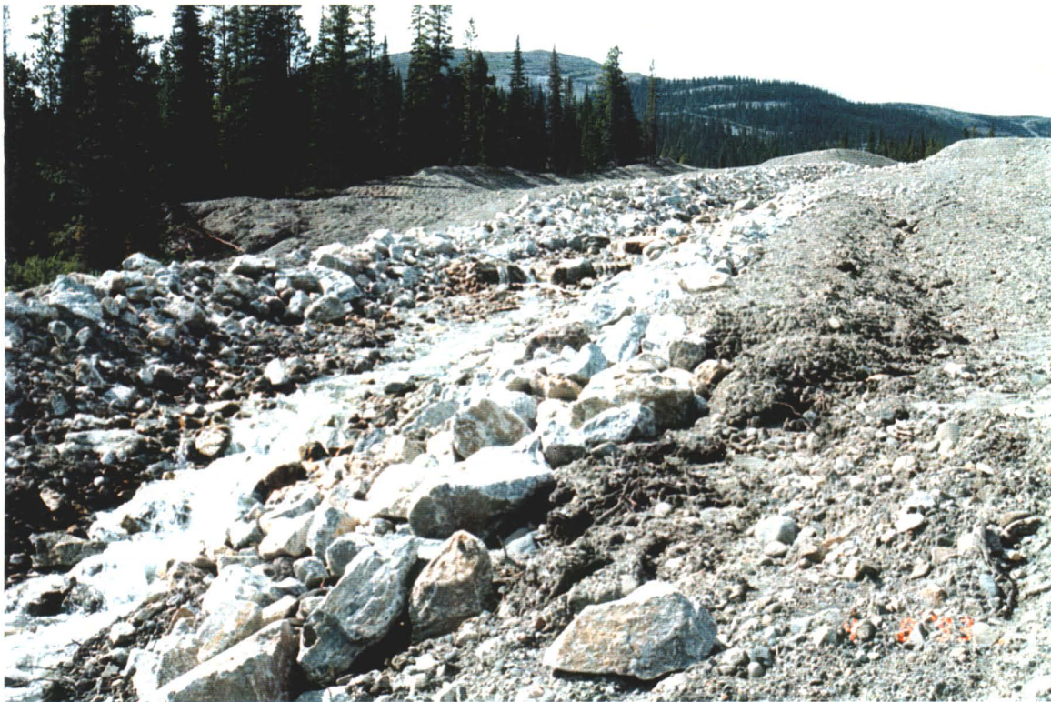
Photo 5 : Detail view of the chute.
