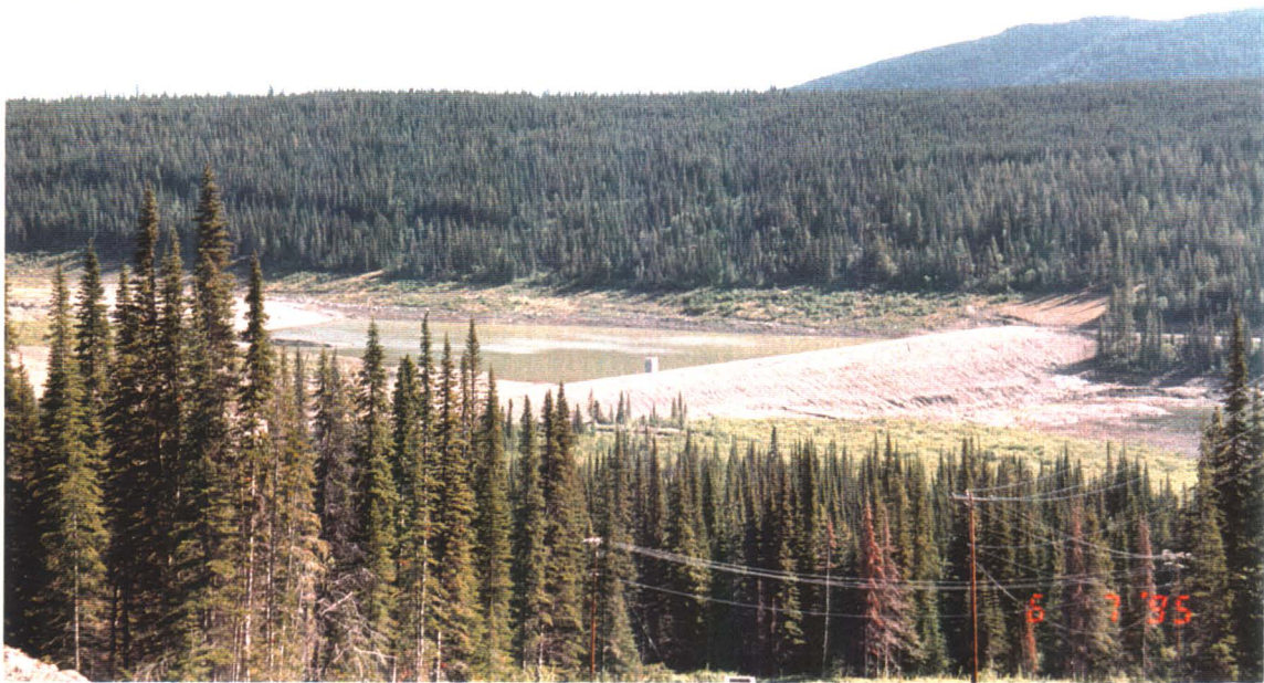
Photo 2: View of the South Dam and deposited tailings.
