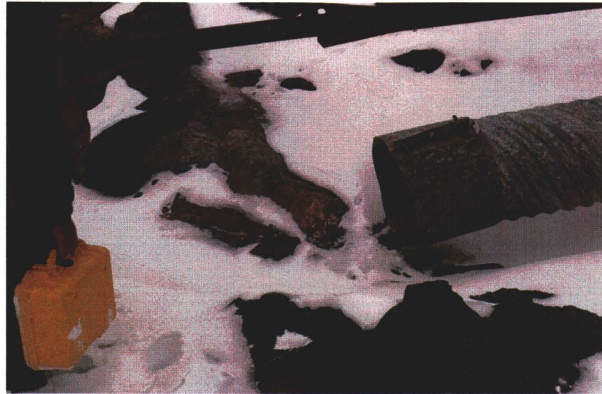
Photograph 16: Drainage pipe from lower adit with no flow
