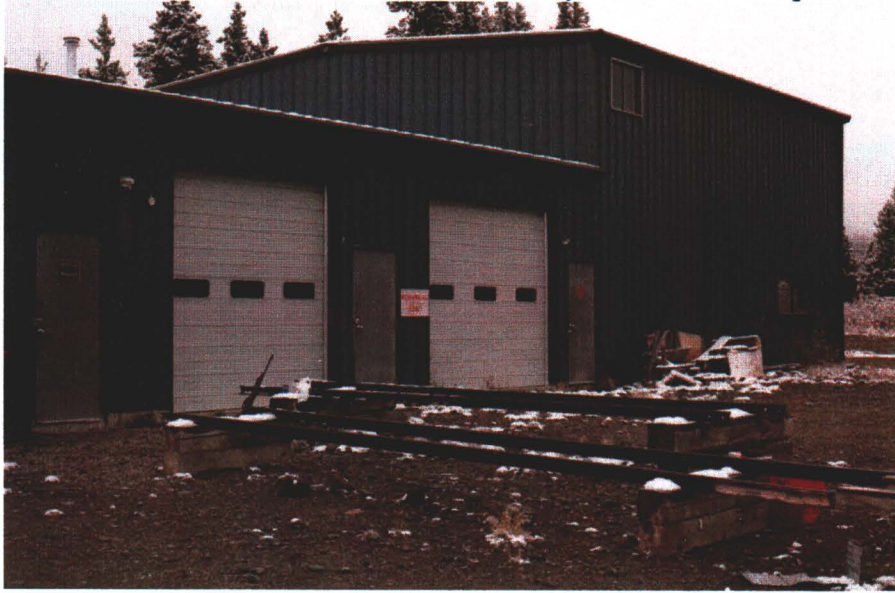
Photograph 2: Front of maintenance and core storage building
