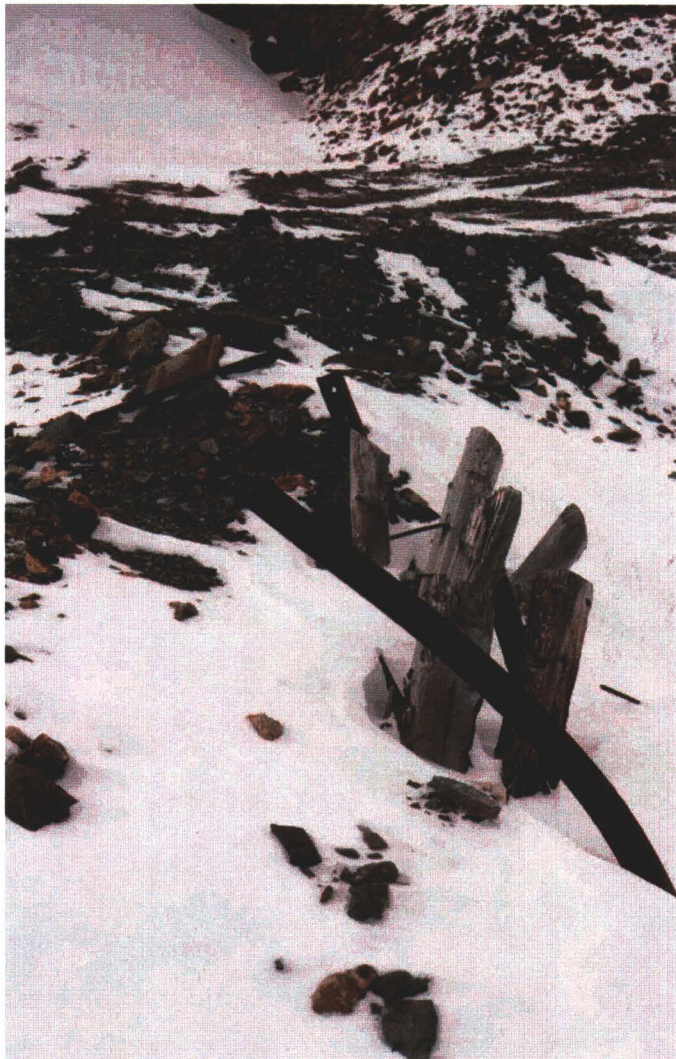
Photograph 17: Wood and metal debris at upper portal
