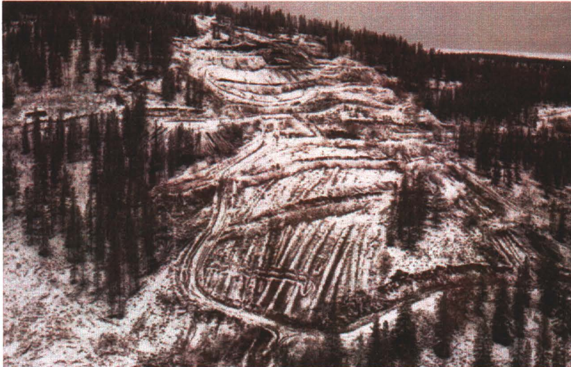
Photograph 12: Area of main ore body showing deforestation and extensive trenching which could result in increased erosion
