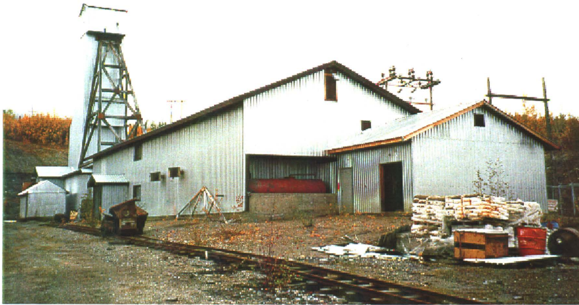
Photo 2-15: Structures at site.
