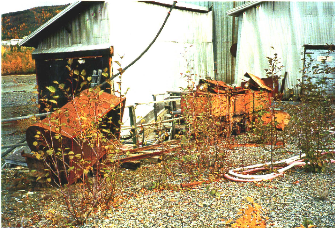
Photo 2-10: West side of headframe.
