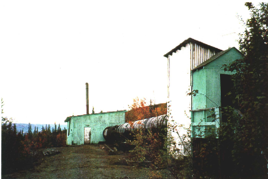
Photo 2-1: Boiler house down draft raise & duct.
