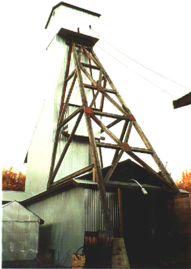
Photo 2-14: Shaft headframe house.
