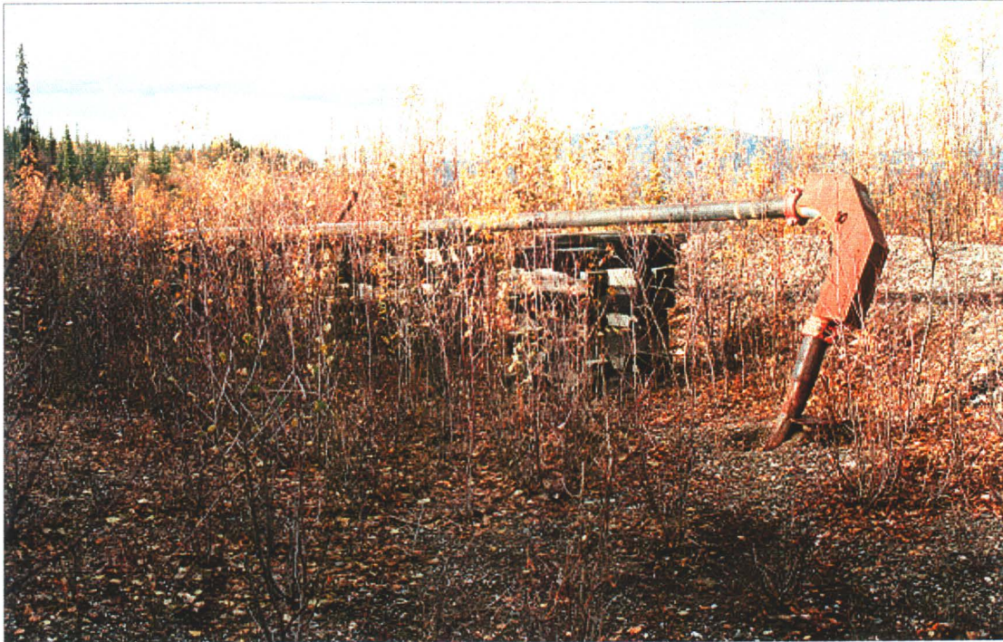
Photo 3-5 : Elsa Mine. Elsa mine backfill pipe. Looking west.
