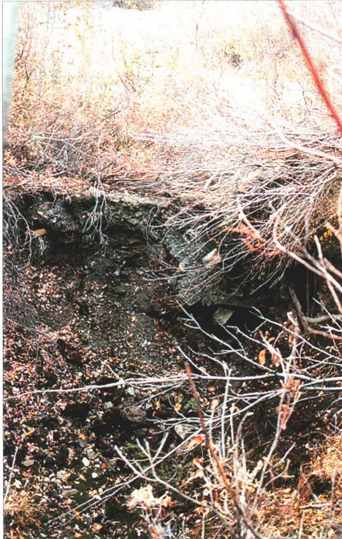
Photo 3-6 : Elsa Mine. Collapsed ventilation raise, Powderhouse Corner on Calumet Drive. Sink hole is about 10m by 10m by 5m deep. Looking north.
