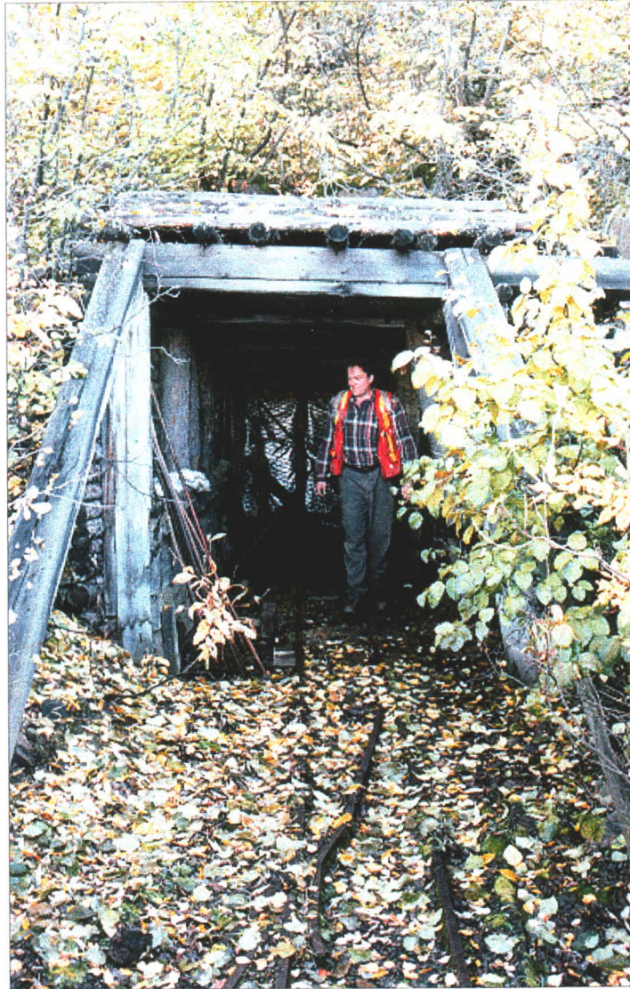
Photo 3-4 : Elsa Mine. Elsa 200 Level Portal. Looking south.
