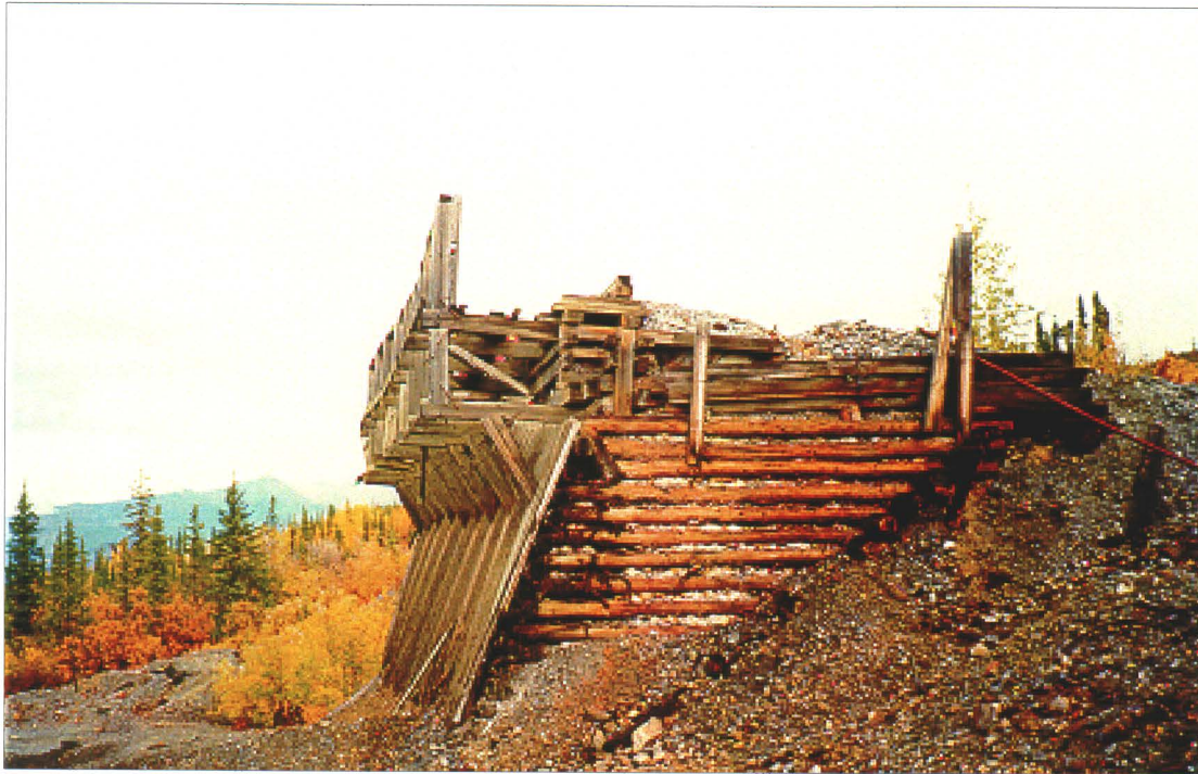
Photo 4-5: The loading area at the main Dixie mine site. (Azimuth 80°)
