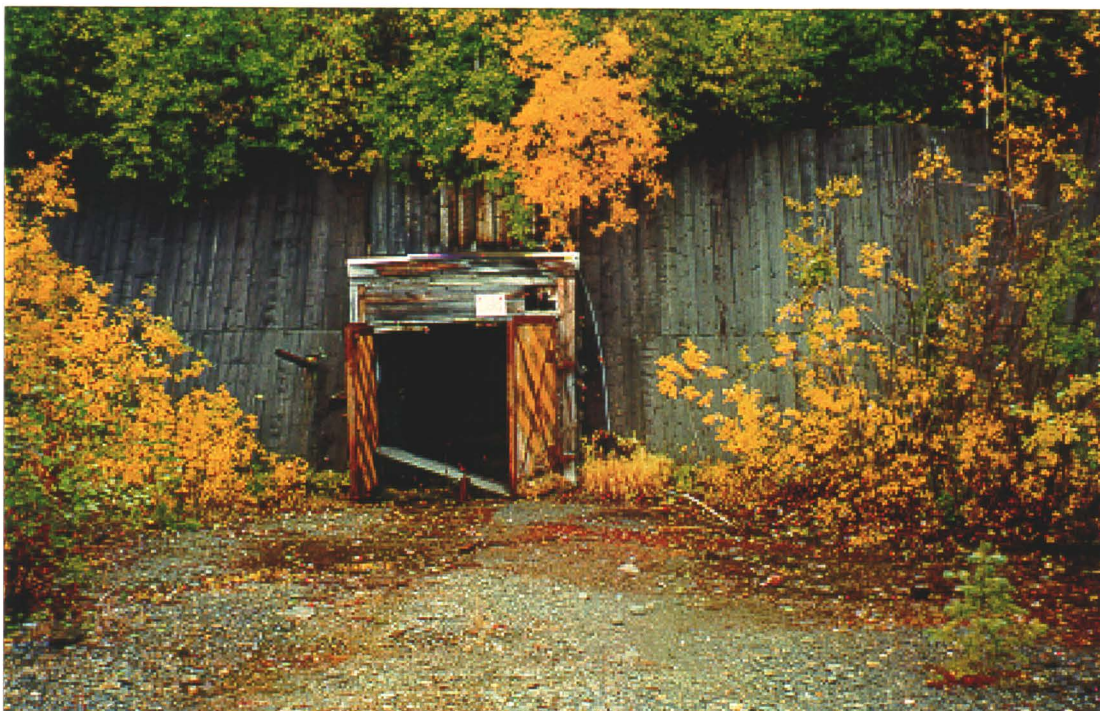
Photo 4-1: Photograph of the adit at Dixie Mine, note the portal entrance has been blocked off with timber cribbing. (Azimuth 145°)
