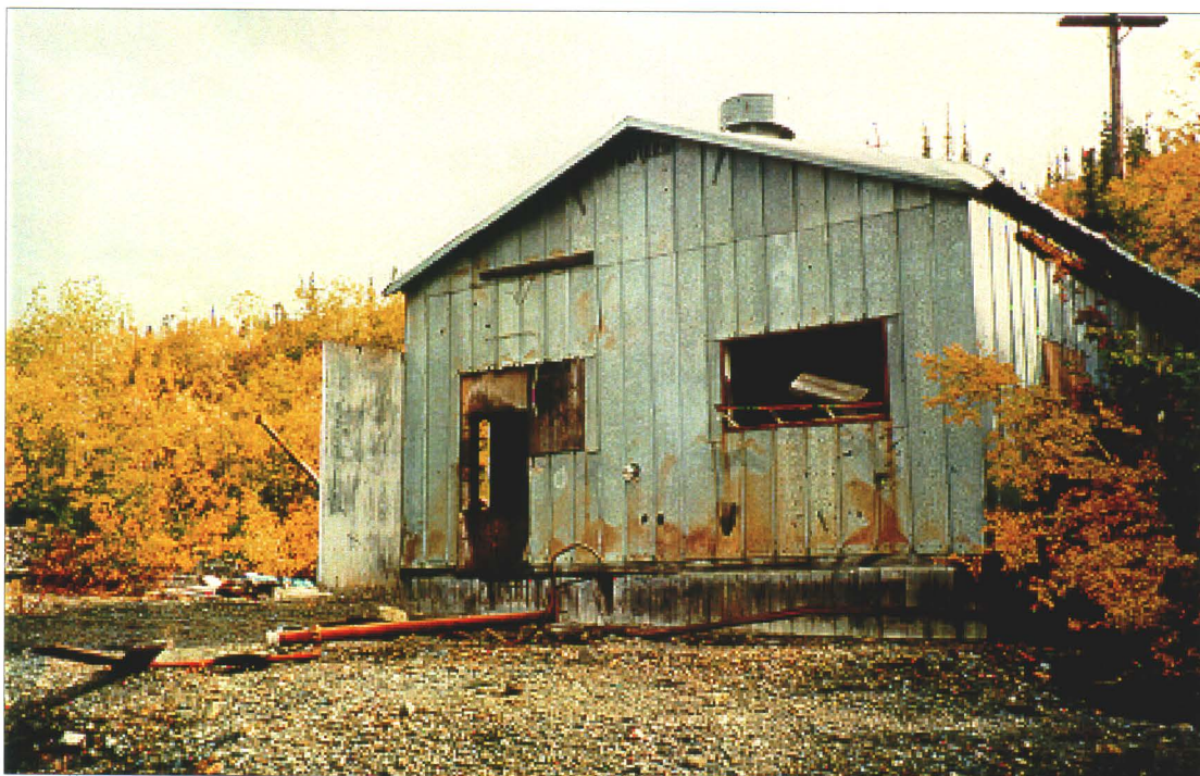
Photo 4-6: Building 4A (garage/office) facing NE. (Azimuth 75°)
