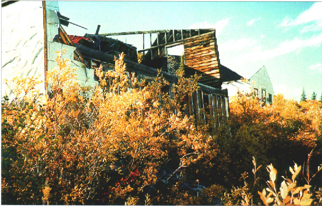
Photo 6-8 : Bermingham Adit. Buildings 4 & 5. Wood frame asphalt shingles - tar paper exterior. (Azimuth 195°)
