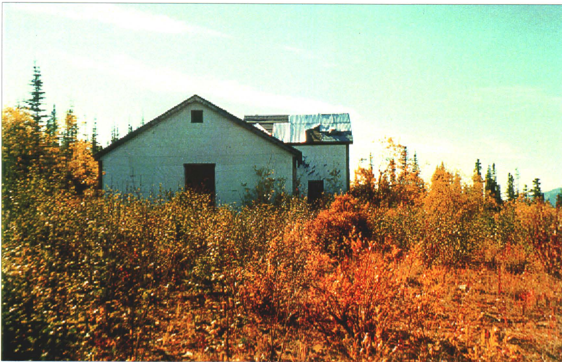
Photo 6-3 : Bermingham Pit. Building 1. Explosives magazine. (Azimuth 235°)
