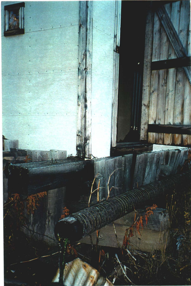
Photo 6-6 : Bermingham Adit. Wooden pipe extending from Building #3. (Azimuth 160°)
