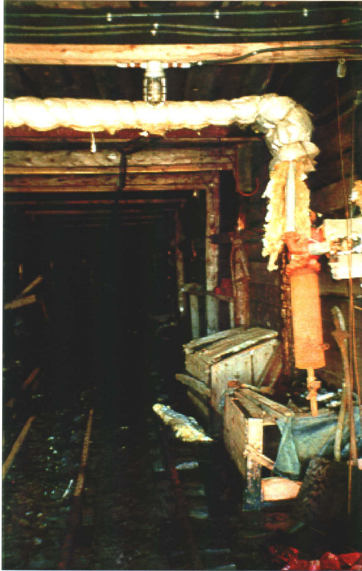
Photo 6-16 : Ruby 400. Interior photo of the adit structure.
