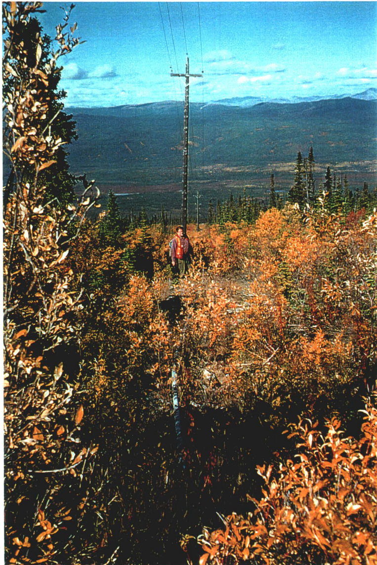
Photo 6-11 : Bermingham Adit. Powerlines from Adit. Also note wooden pipe extends down along powerline.
