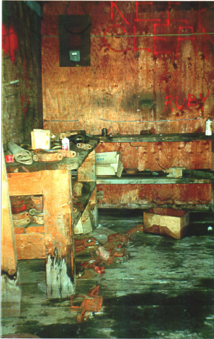
Photo 6-19 : Ruby 400. Interior of the shop area of the garage.
