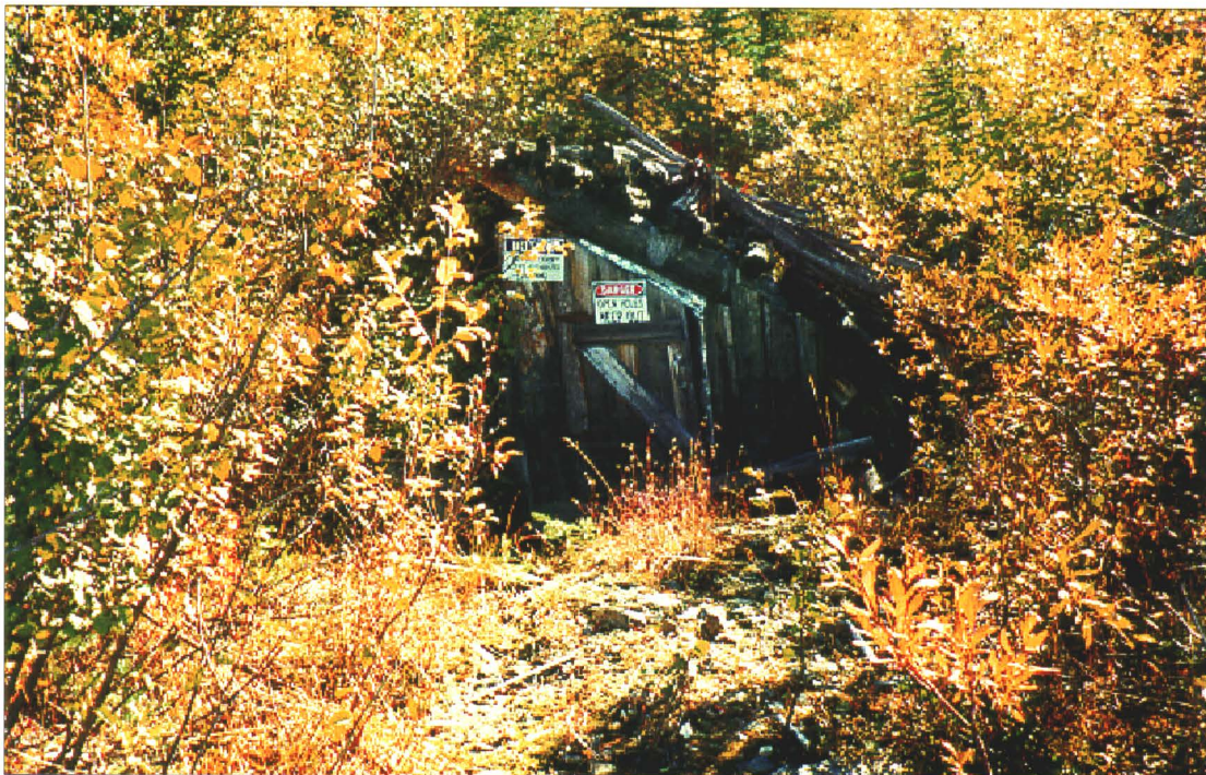
Photo 6-9 : Bermingham Adit. Portal at Bermingham Adit. (Azimuth 170°)
