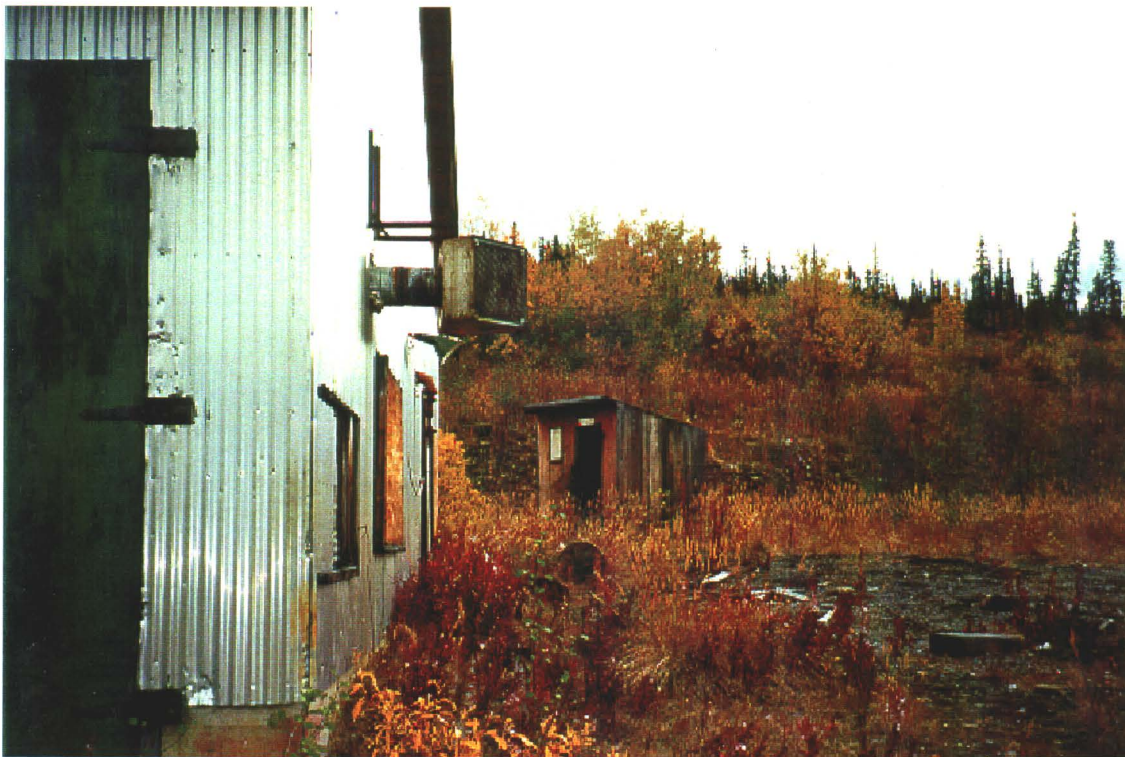
Photo 7-7: Shed on the southwest corner of garage that housed unknown product (samples taken).
