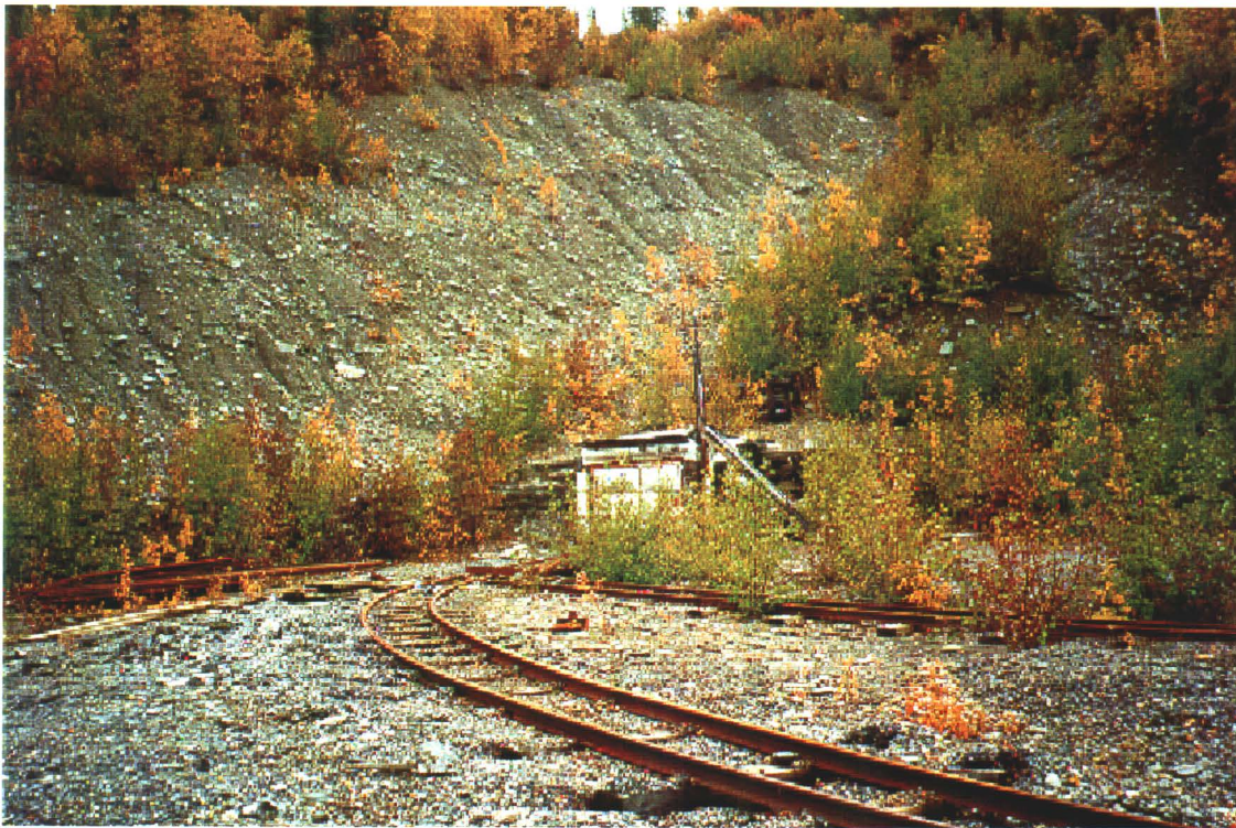
Photo 7-17: Rails extending from the adit.
