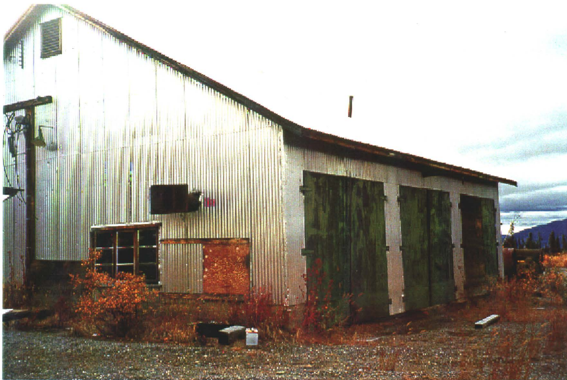
Photo 7-4: Garage structure located adjacent to the shafthouse. Note the batteries in the foreground.
