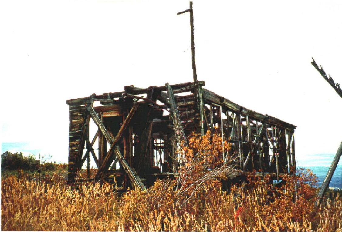
Photo 7-3: Tramway midstation structure.
