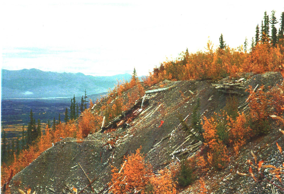
Photo 7-19: Waste rock dump with pipe in the background providing drainage from the underground workings.
