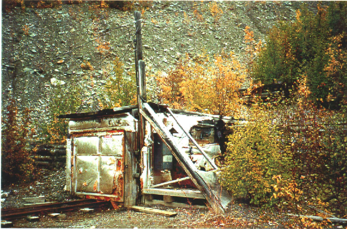
Photo 7-16: Adit structure leading to the 500 level..
