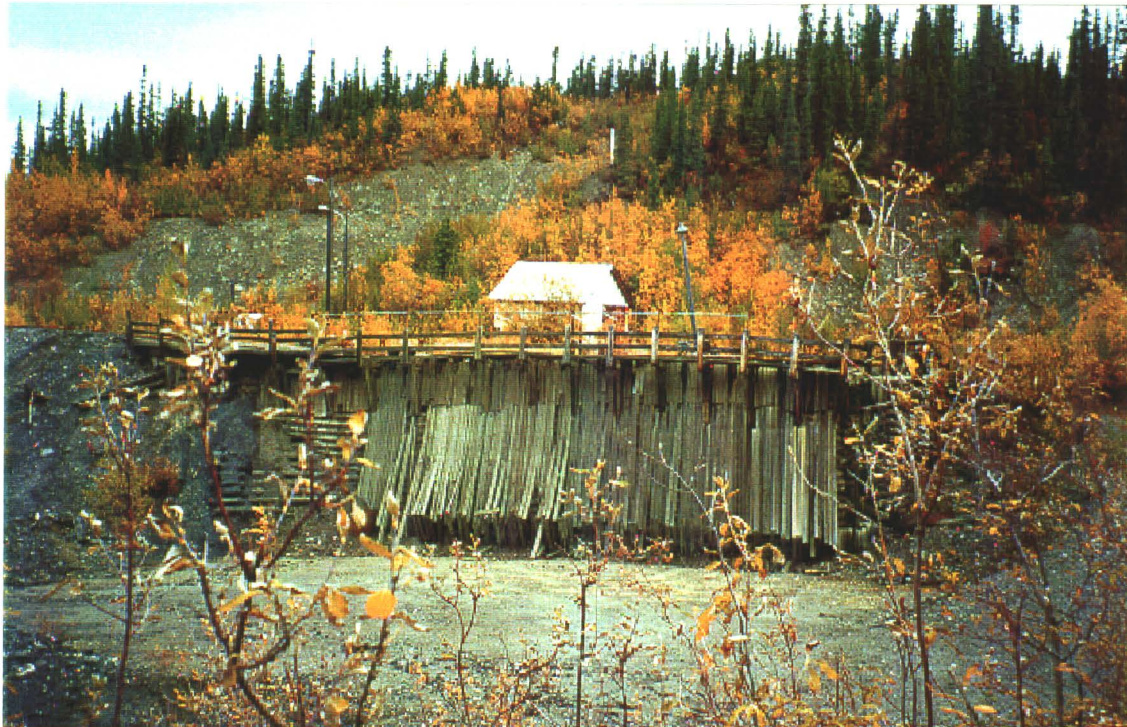
Photo 7-14: Timber retaining wall for the loading dock.
