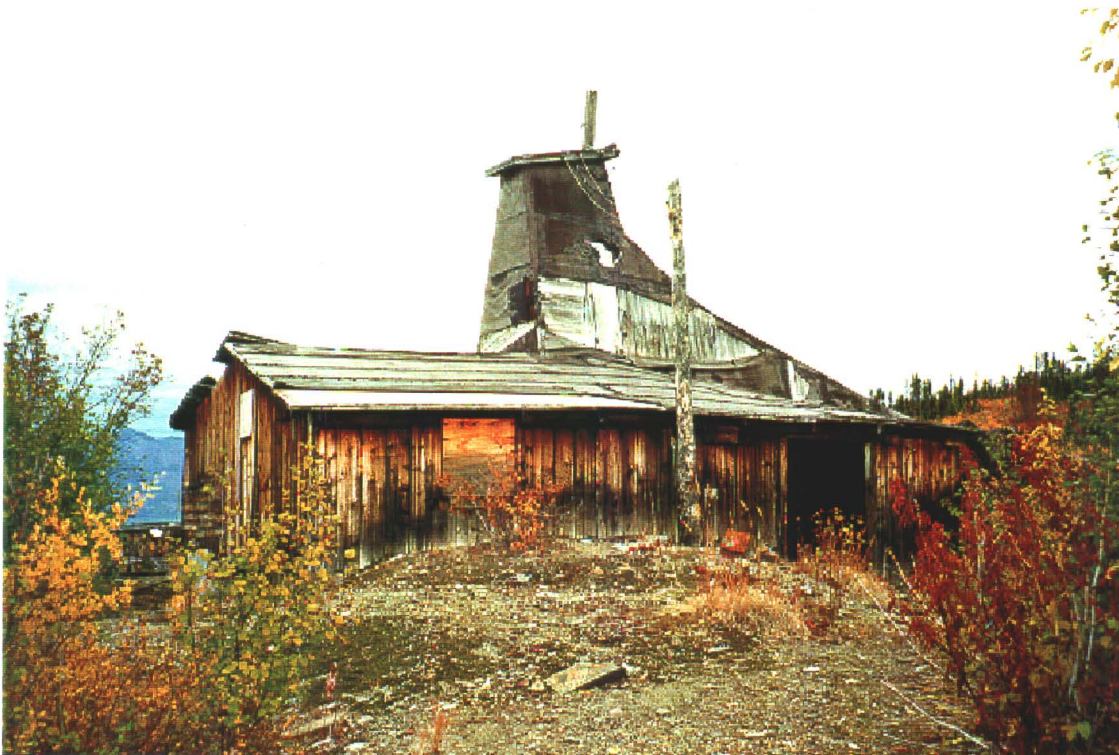
Photo 7-8: Shafthouse located to the east of the garage.
