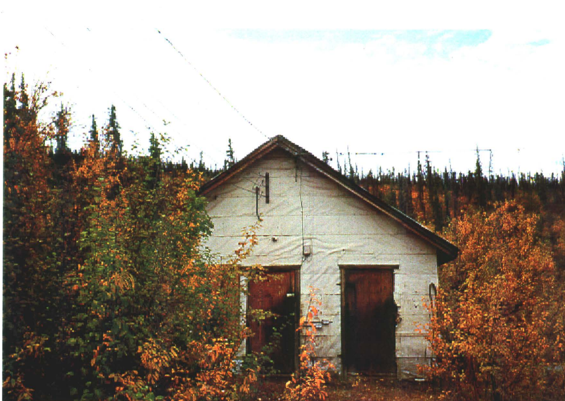
Photo 7-15: Garage structure located to the south of the adit.
